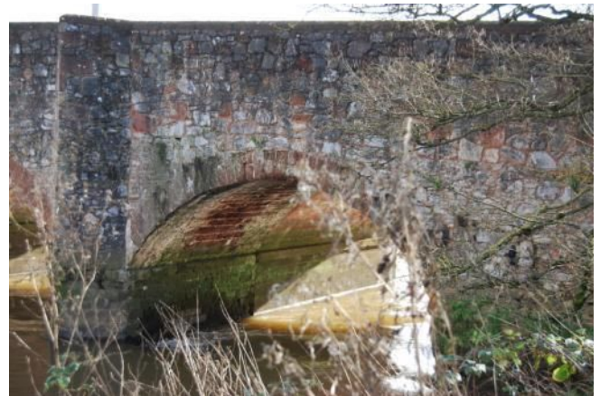
Plate 13. Western arch, upstream elevation (looking SE)
