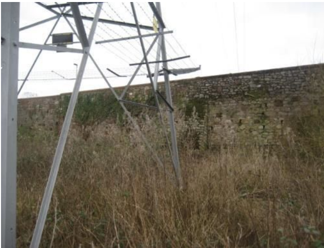
Plate 24. Eastern end of upstream elevation (looking SE)
