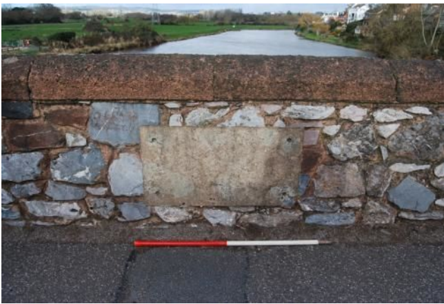
Plate 18. Backing stone for plaque, upstream parapet (looking NW) (1m scale)
