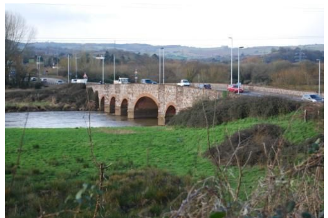
Plate 7. Downstream elevation (looking NWW)
