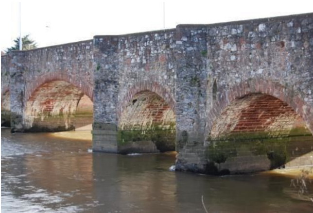
Plate 12. Cutwater Types A & B, upstream elevation (looking E)
