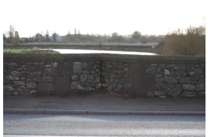
Plate 21. Refuge, downstream parapet (looking SE)
