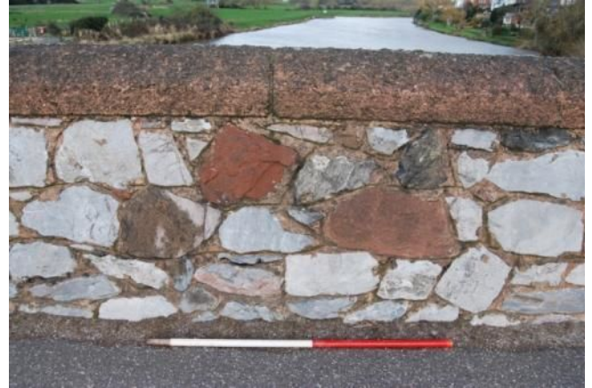
Plate 17. Upstream parapet (looking NW) (1m scale)
