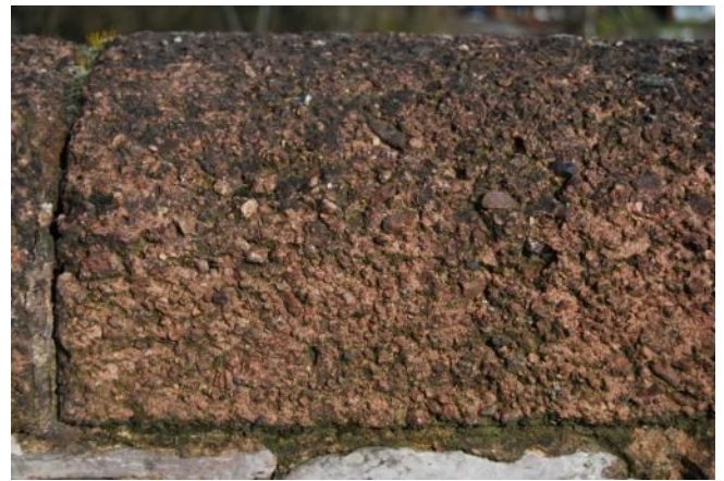
Plate 19. Red cement coping, upstream parapet (looking NW)
