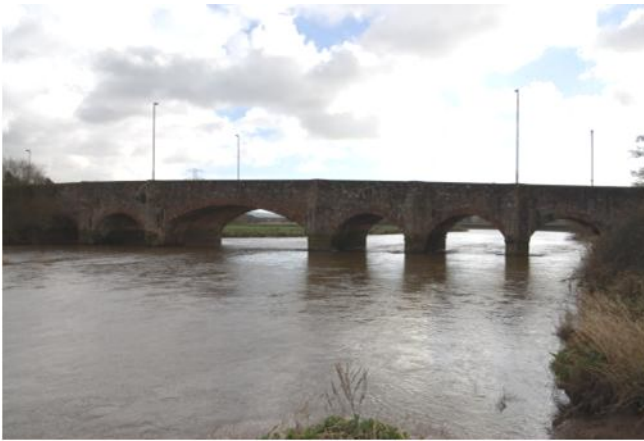
Plate 4. Upstream elevation (looking SE)
