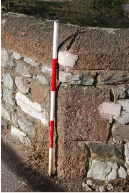
Plate 22. Quoin of refuge, upstream parapet (looking NW)
