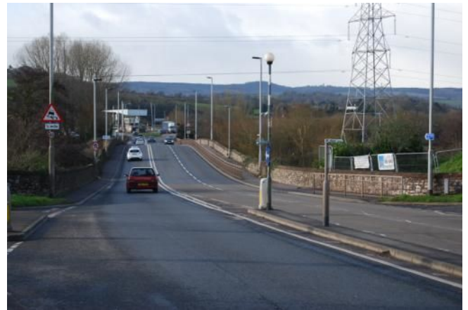
Plate 5. Carriageway across bridge (looking SW)
