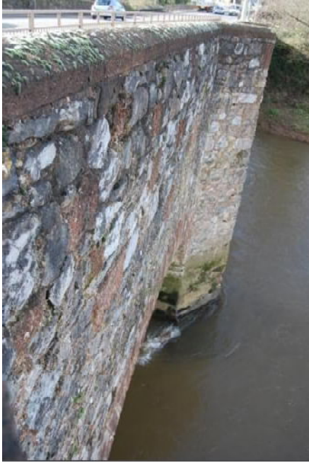
Plate 10. Cutwater Type A, upstream elevation (looking SW)
