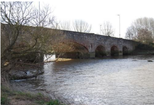
Plate 8. Upstream elevation (looking SW)
