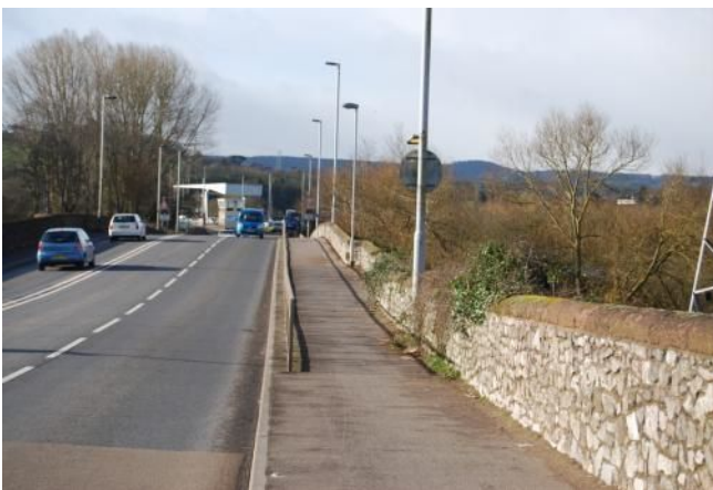
Plate 6. Upstream side of carriageway across bridge (looking SW)
