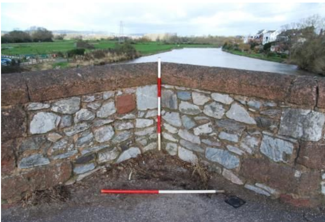
Plate 20. Refuge, upstream parapet (looking NW)
