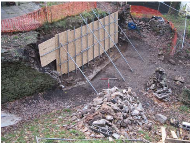
General view of the excavated trench, looking south-west (scales 1m)
