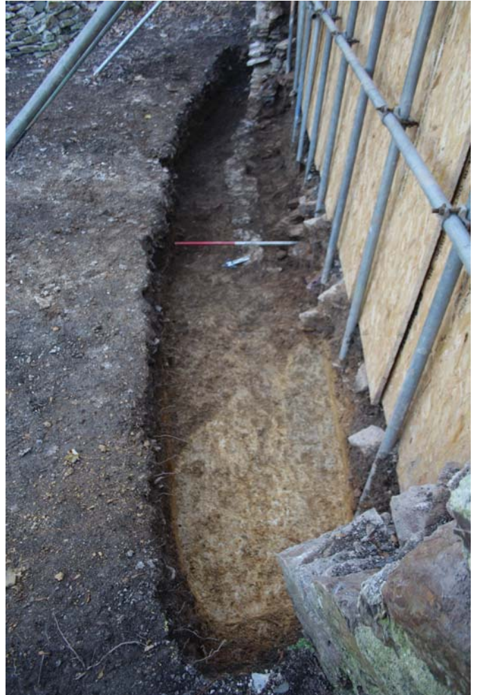
View of the excavated trench, looking south-east (scale 1m)
