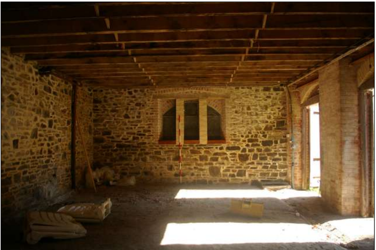
51. THE CARRIAGE HOUSE FROM THE WEST, WITH 2M SCALE.
