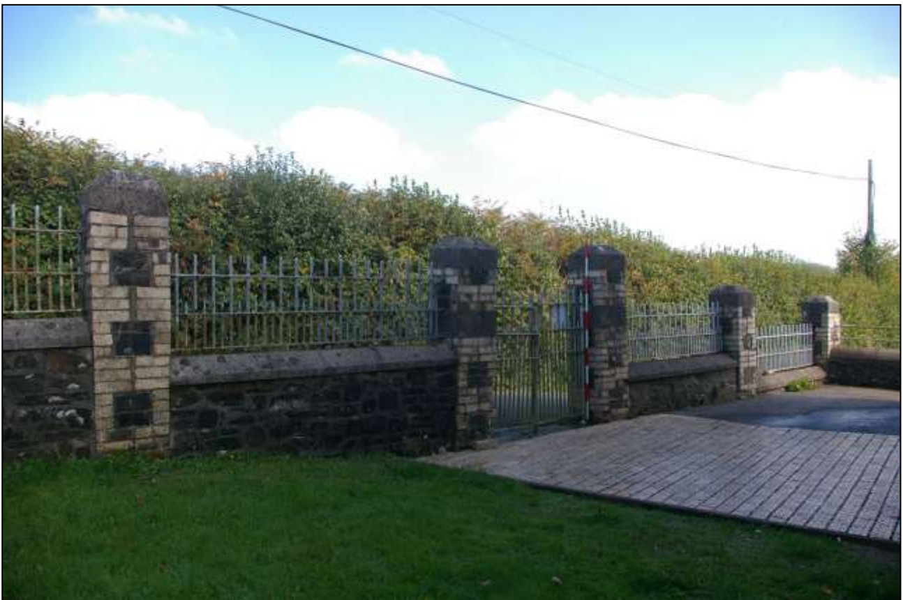
6. THE CERAMIC BRICK AND STONE RUBBLE DECORATIVE PIERS AND RAILINGS TO THE FRONT OF THE CHAPEL; FROM THE SOUTH-WEST.
