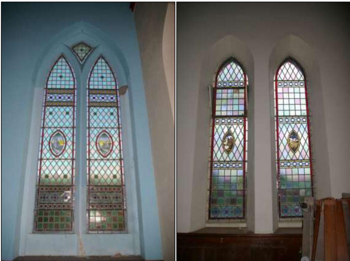
81. LEFT: WINDOW 2; FROM THE SOUTH.
