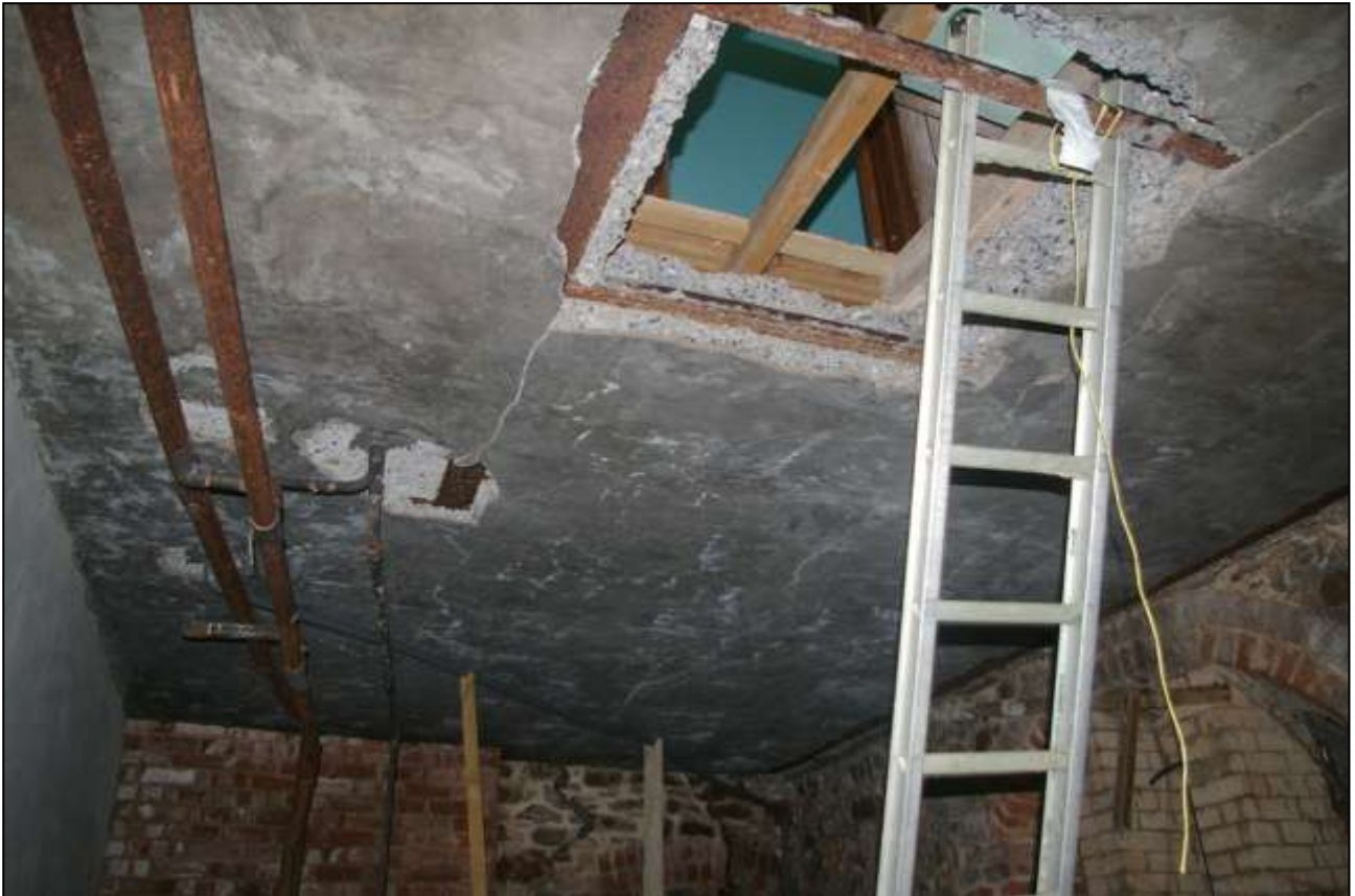
39. THE CONCRETE CEILING IN THE WESTERN END OF THE REAR CROSSWING, WHERE WOODEN JOISTS HAVE FAILED IN THE PAST, A LATER ALTERATION? FROM THE NORTH-EAST.
