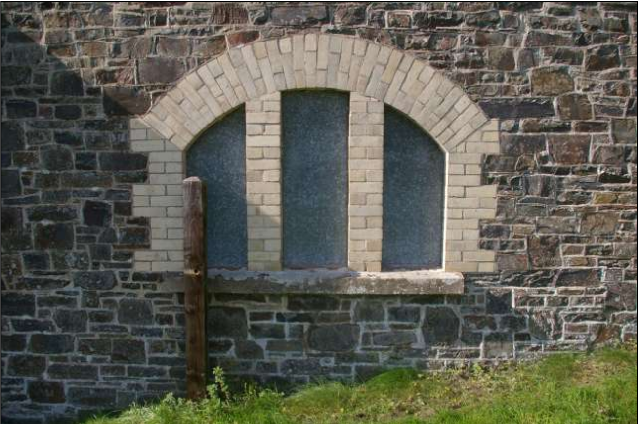
21. THE EAST TRIPARTITE WINDOW, LIGHTING THE CARRIAGE HOUSE, BLOCKED EXTERNALLY; FROM THE EAST.
