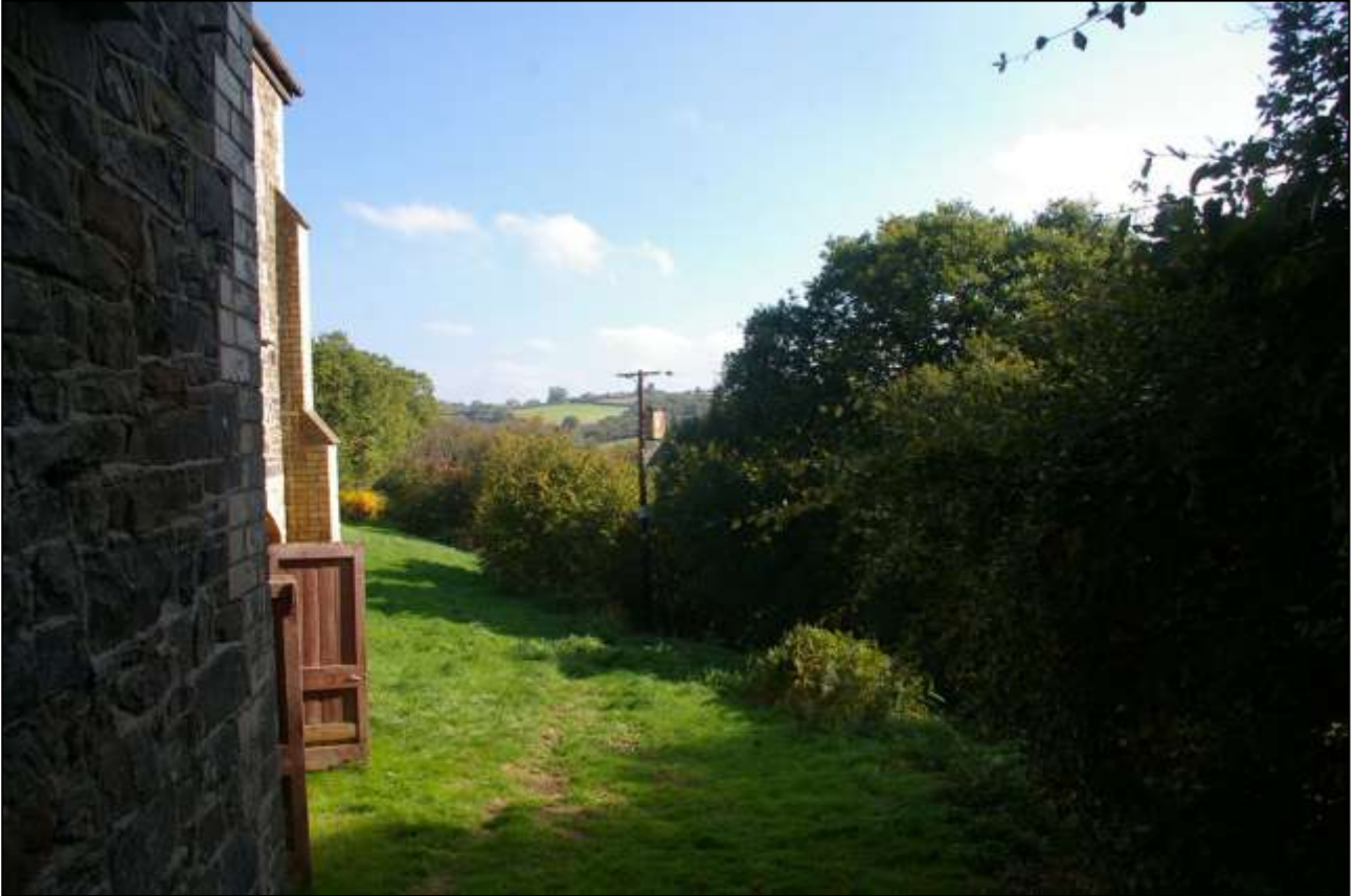
27. VIEW ALONG THE SOUTH ELEVATION OF THE REAR CROSSWING SHOWING THE CHAPEL'S SETTING; FROM THE WEST.
