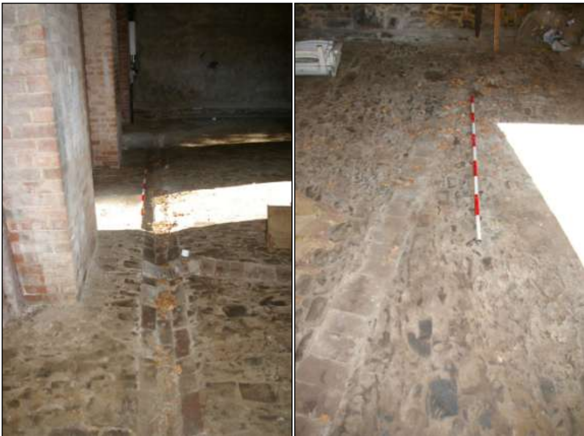
48. LEFT: THE BRICK DRAIN TO THE SOUTH SIDE OF THE COBBLED FLOOR IN THE CARRIAGE HOUSE, 2M SCALE; FROM THE EAST.
