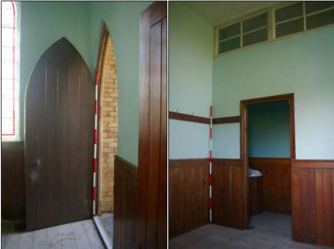
112. LEFT: D6, WITH 2M SCALE; FROM THE EAST.
