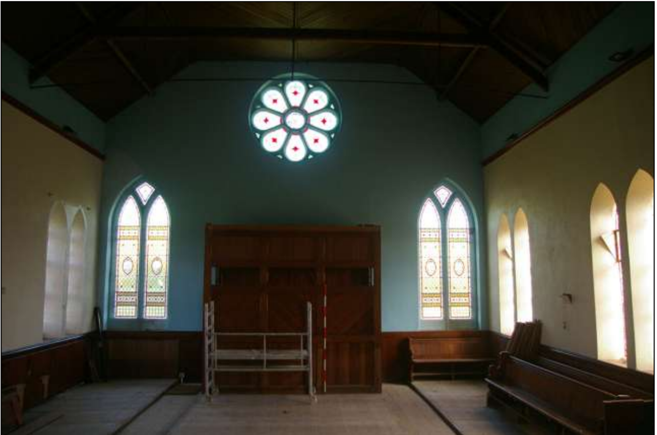
76. THE NORTH WALL OF THE CHAPEL, WITH 2M SCALE; FROM THE SOUTH.
