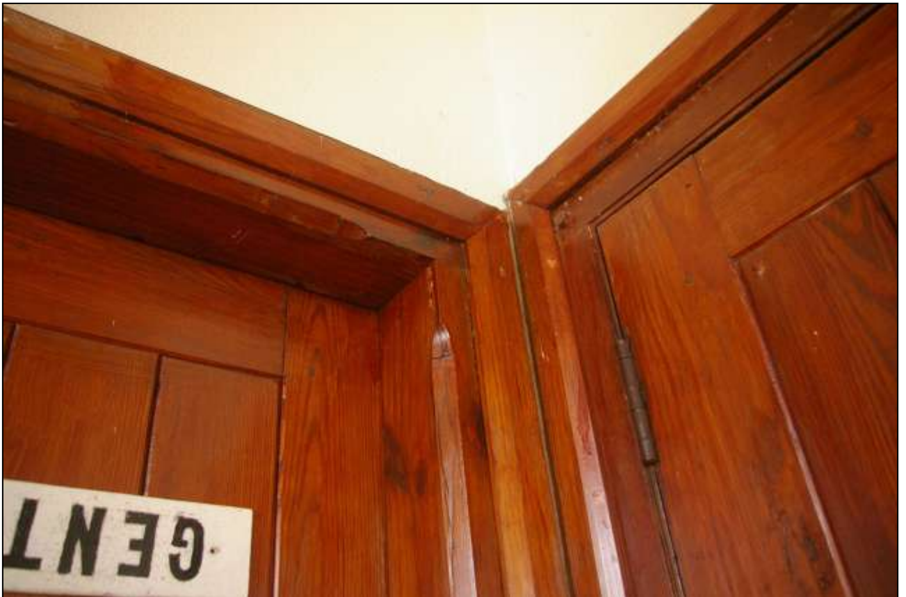
109. DETAILED VIEW OF THE DIFFERENT CHAMFERED OR BEADED DOORFRAMES IN THE BUILDING; FROM THE SOUTH-EAST.
