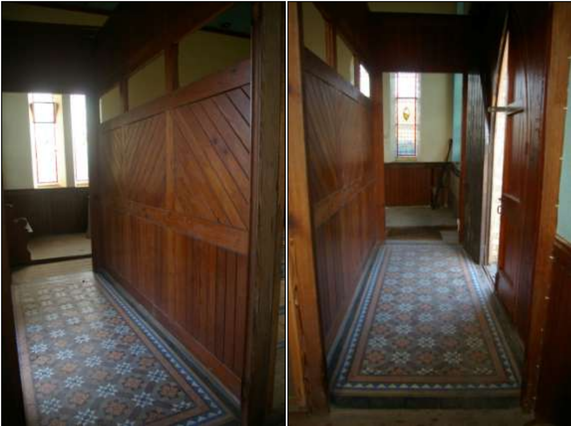
58. LEFT: THE FINE DIAGONAL BOARDING OF THE PORCH SCREEN; FROM THE WEST-NORTH-WEST.
