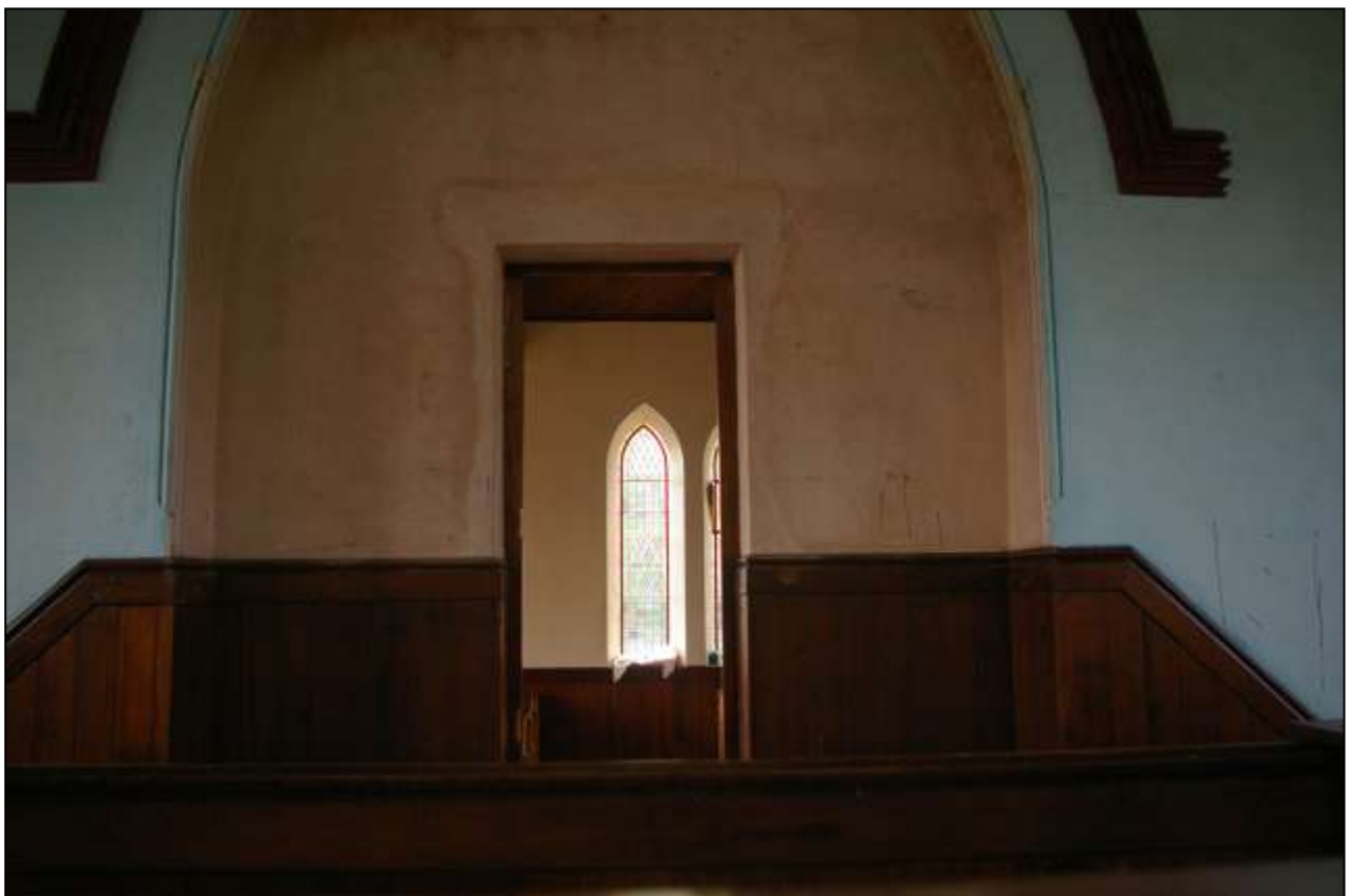
71. THE MODERN FORCING OF AN OPENING TO THE BACK OF THE ALCOVE ABOVE THE PULPIT; FROM THE NORTH.
