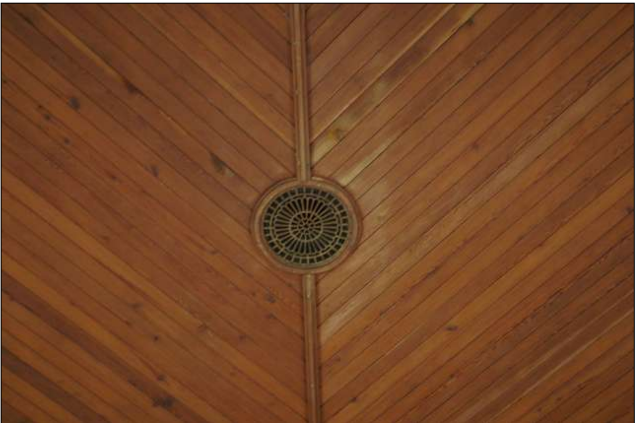
79. THE FOLIATE PATTERN ROOF VENTS IN THE CHAPEL; FROM BELOW.
