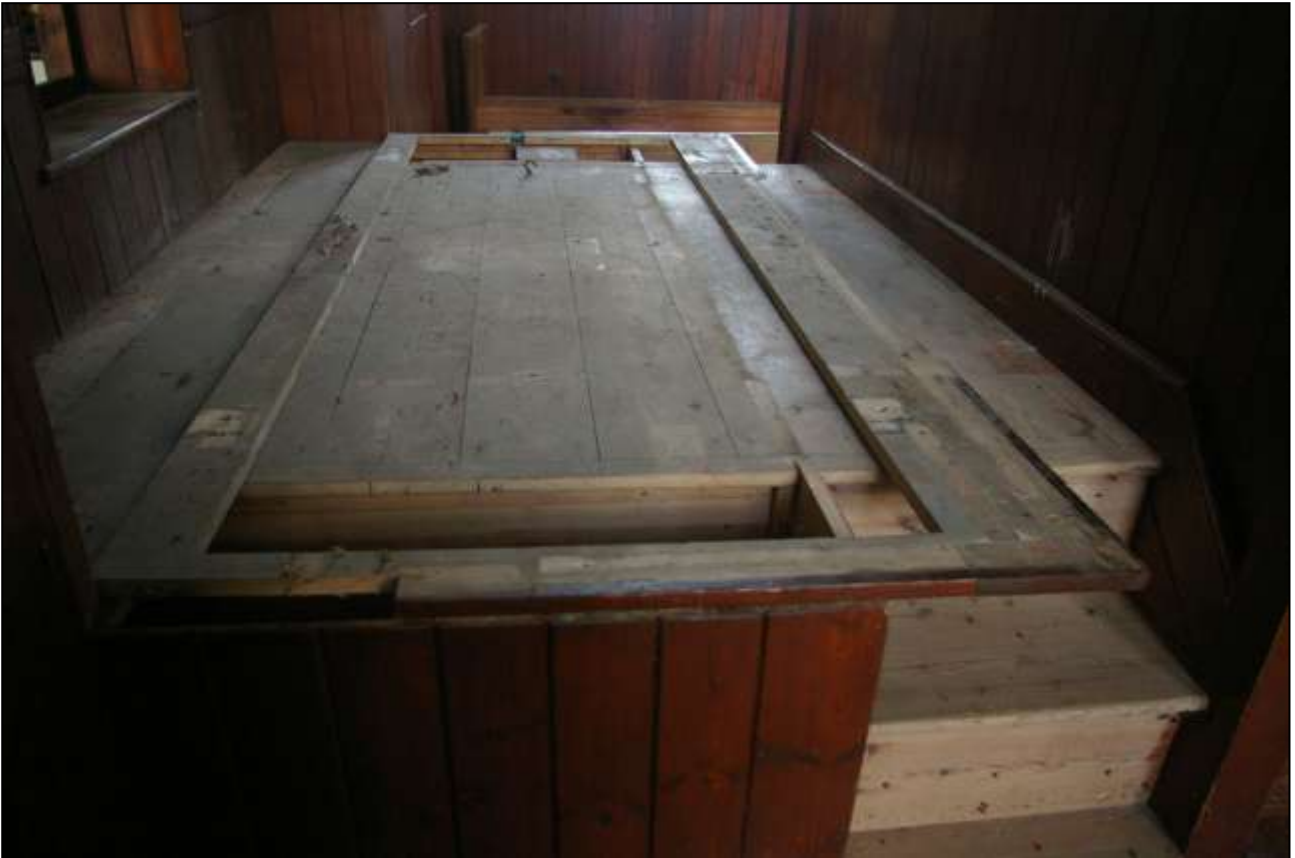
74. THE MODERN WOODWORK TO CARRY THE ORGAN, HIDDEN BEHIND RESET PANELLING, BEHIND THE PULPIT; FROM THE EAST.
