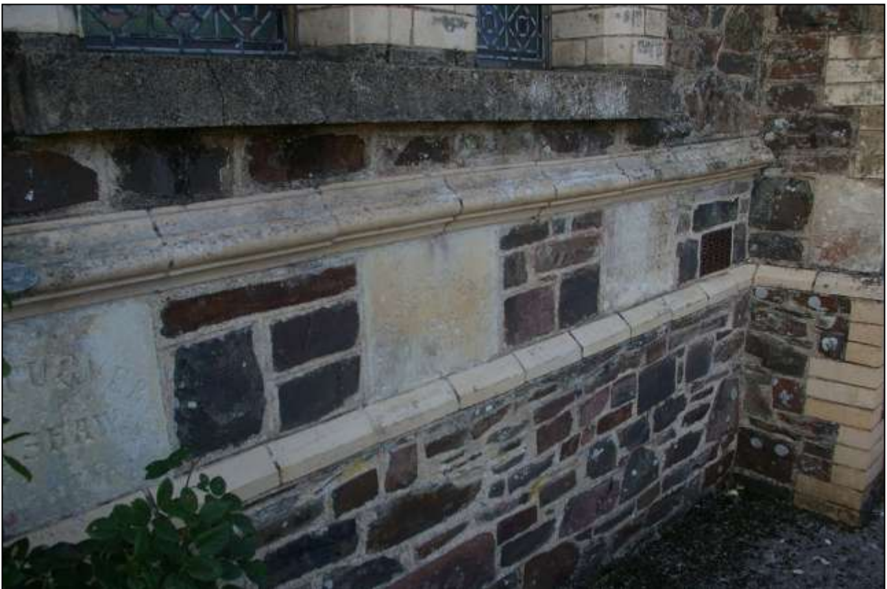
18. THE STRING COURSE AND DECORATIVE PLAQUES WITH THE NAMES OF THE CONTRIBUTORS; FROM THE SOUTH-EAST.
