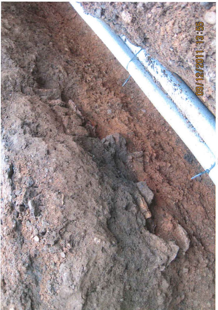
TRENCH 3. SECTION F-F NW END.
