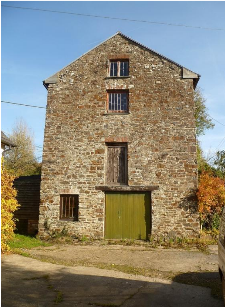
West gable end, from yard between mill and house
