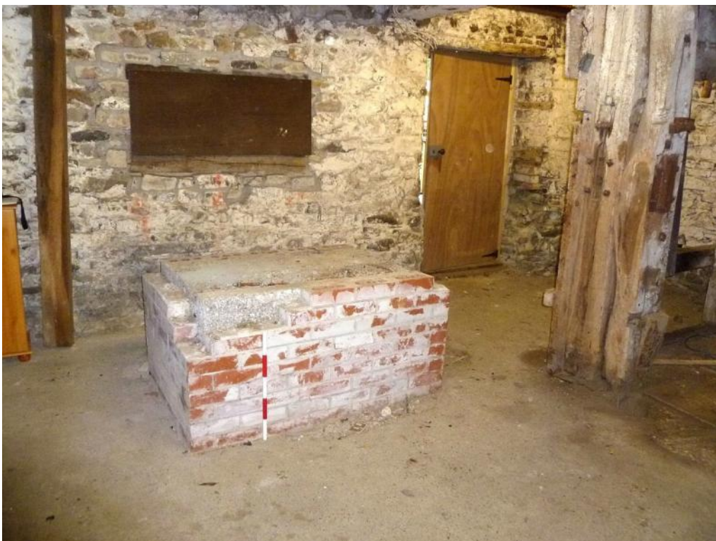
Ground floor. Brick plinth, opening in north wall and modern door
