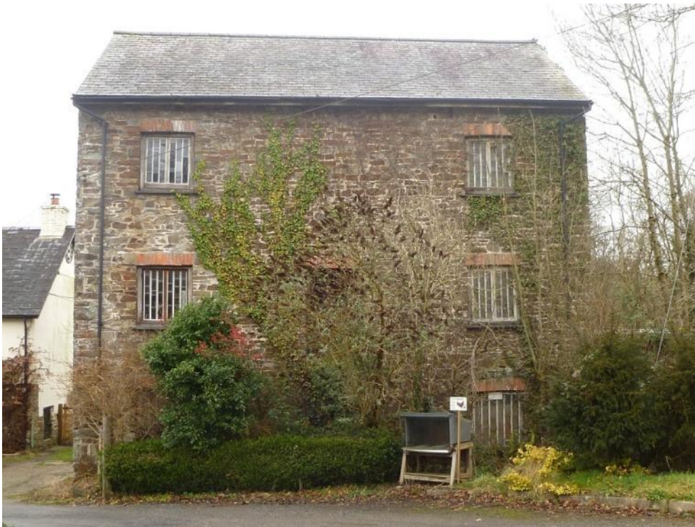
South elevation. The first floor loading door is partially obscured.
