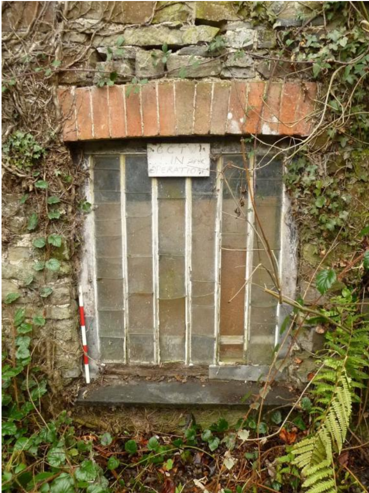
Detail of window opening and glazing, ground floor south
