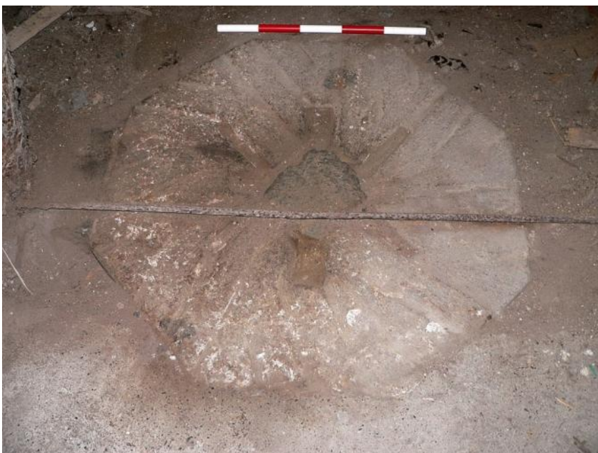
Octagonal granite millstone set in ground floor below hurst
