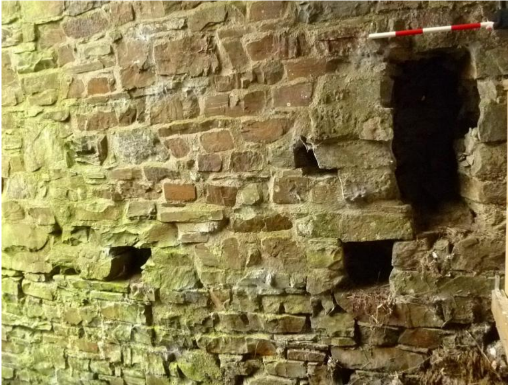
Recesses in pit (east gable) wall (half metre scale)
