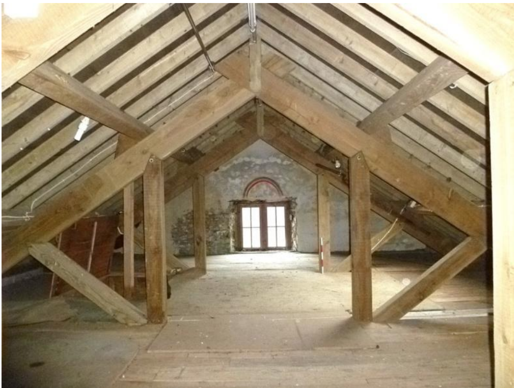
Reconstructed roof, looking west
