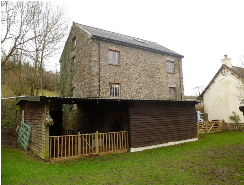
East gable end and north elevation with modern extension
