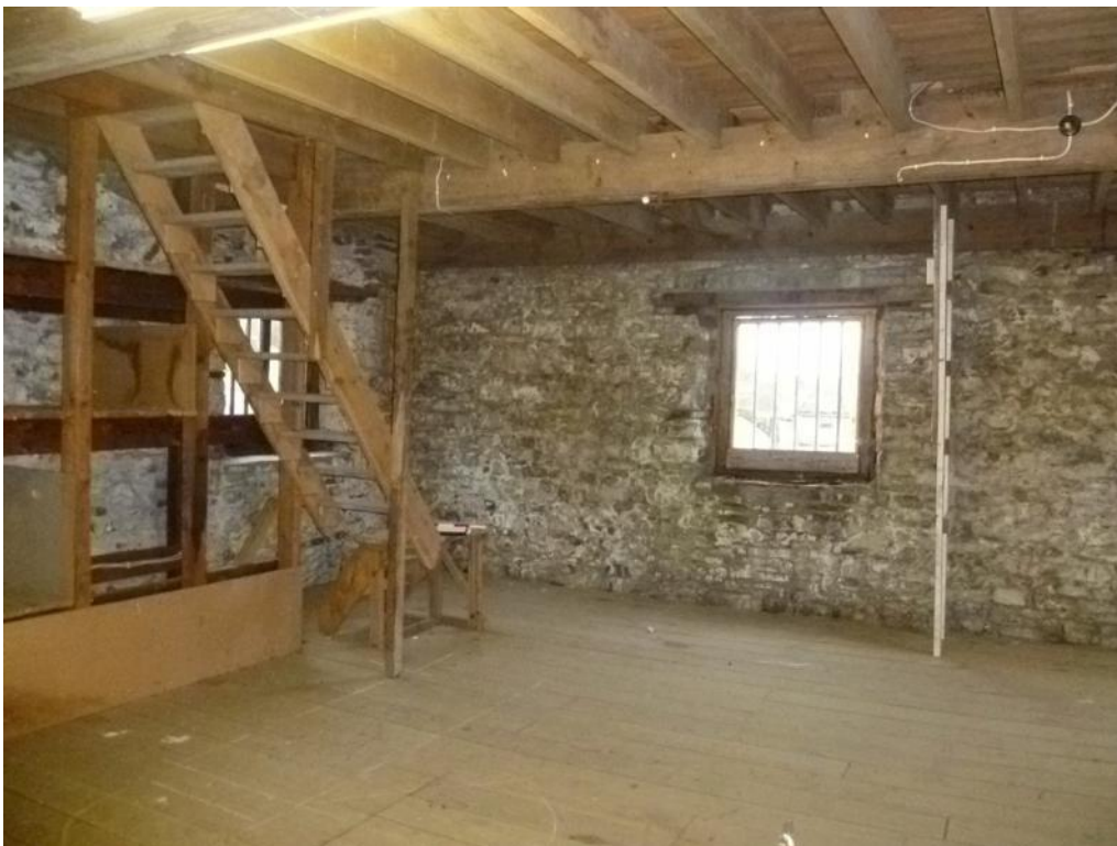
Steps in south-west corner from second floor up to loft
