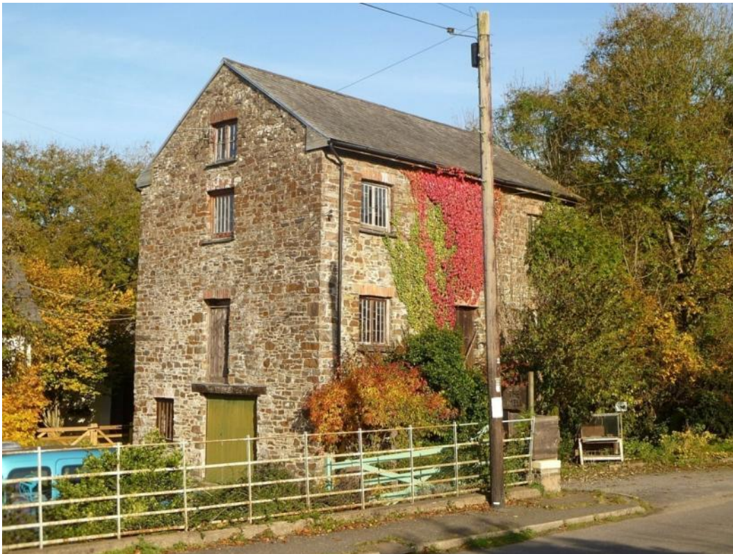
Bish Mill from the south west. 31 October 2016
