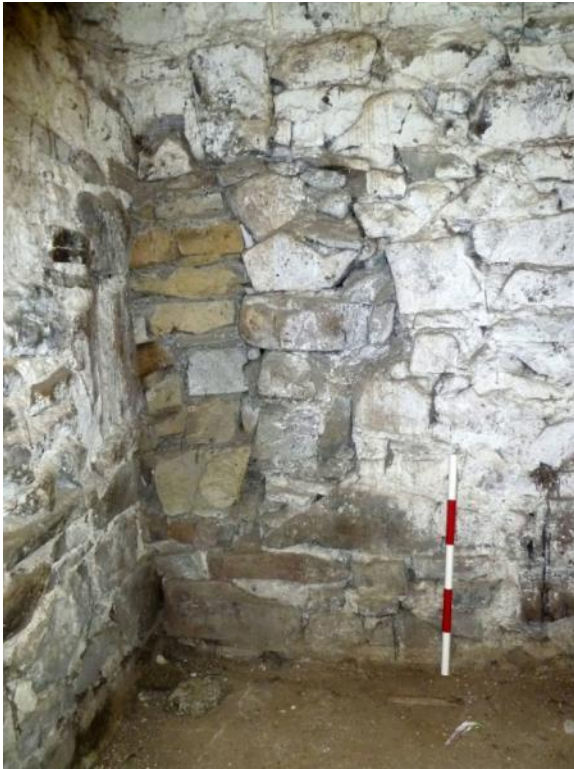
Blocked opening in north-east corner
