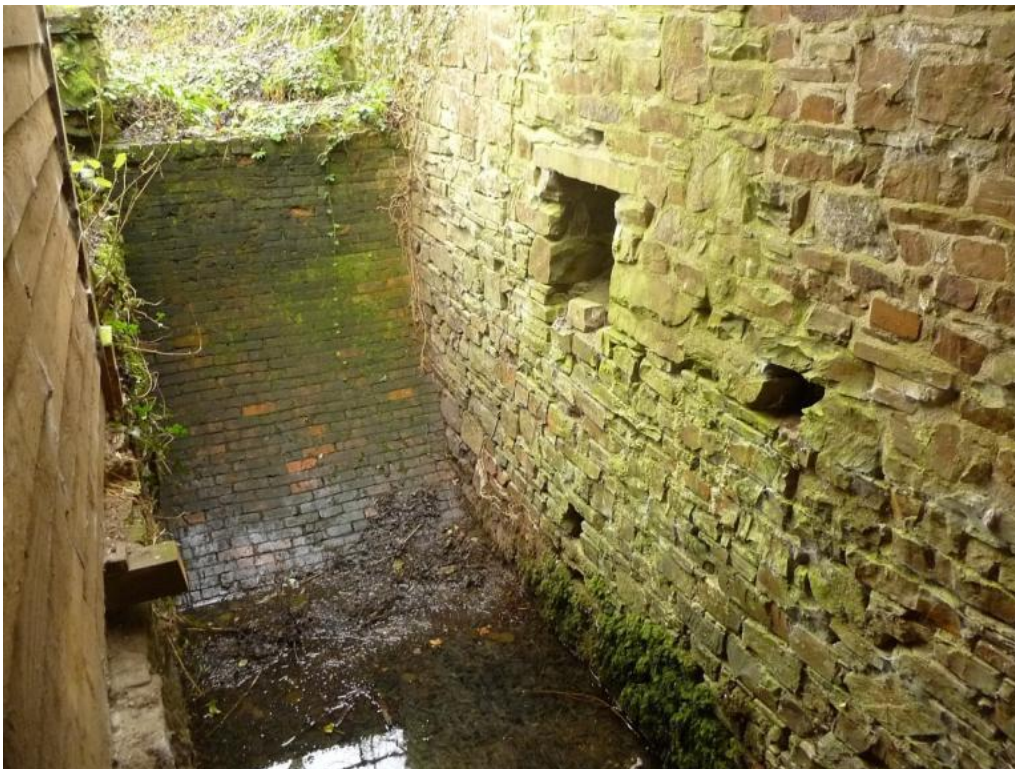
Wheelpit, showing curved brick breastwork at south end and wheelshaft opening
