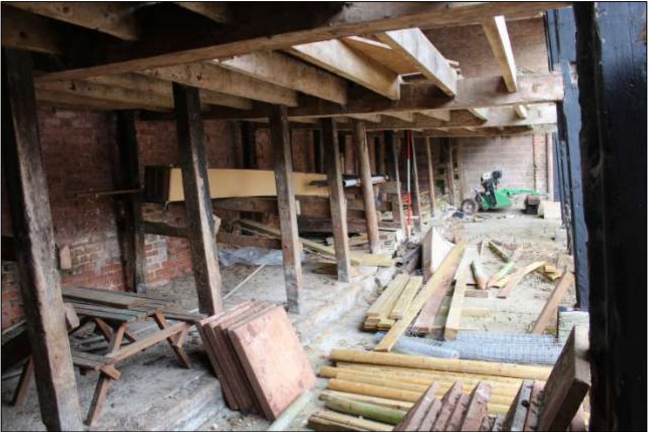
B7 GF INTERIOR; VIEWED FROM THE EAST (SCALE 2M).
