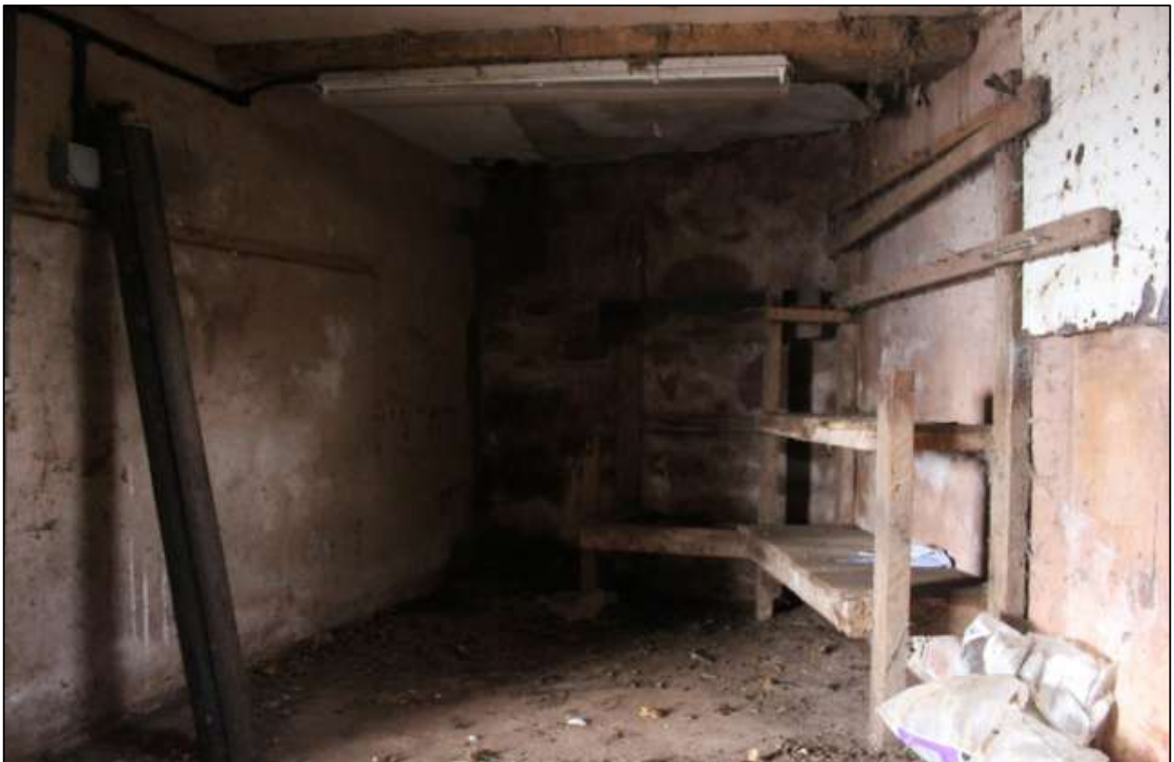
B5 GF INTERIOR; THE DAIRY; VIEWED FROM THE NORTH-EAST.
