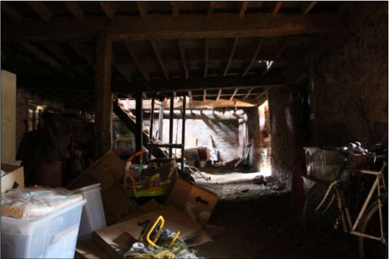
B2 GF INTERIOR; VIEWED FROM THE NORTH.
