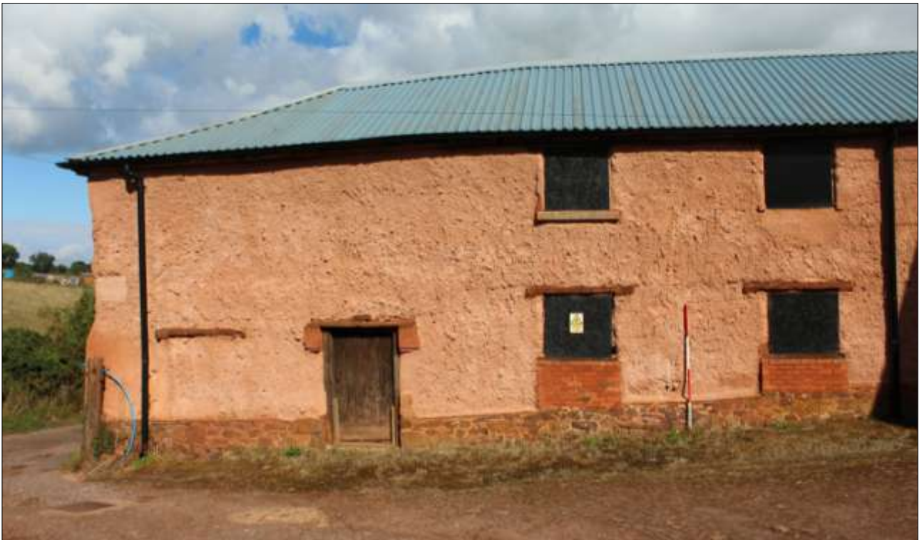
B1 EXTERIOR, THE WEST ELEVATION; VIEWED FROM THE WEST (SCALE 2M).
