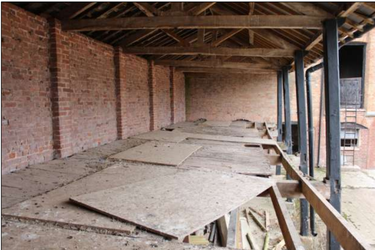
B7 FF INTERIOR; VIEWED FROM THE EAST.
