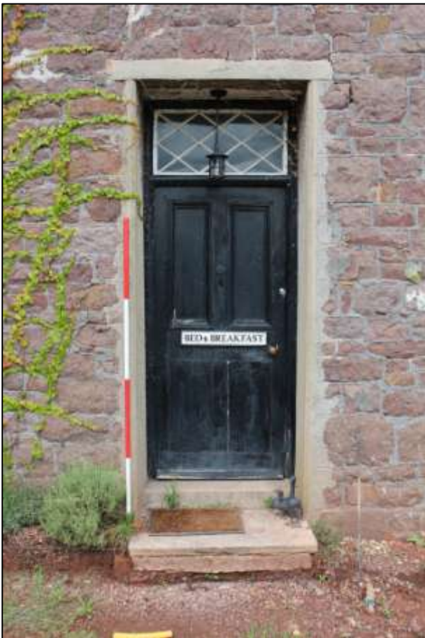
DETAIL OF THE FRONT DOOR OF THE FARMHOUSE; VIEWED FROM THE SOUTH (SCALE 2M).
