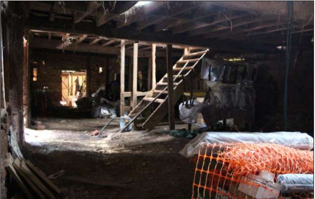
B2 GF INTERIOR; VIEWED FROM THE SSW.
