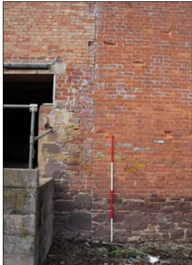
LEFT: AS ABOVE. RIGHT: B7 EXTERIOR, SOUTH WALL, SHOWING HOW THIS ELEVATION ABUTS B6; VIEWED FROM THE SOUTH (SCALE 2M).
