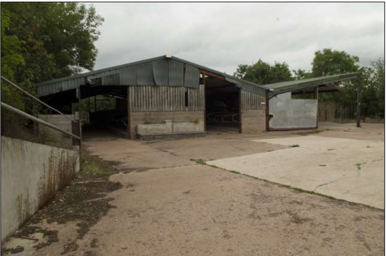
B11 EXTERIOR, THE MODERN COW CUBICLES; VIEWED FROM THE SOUTH.
