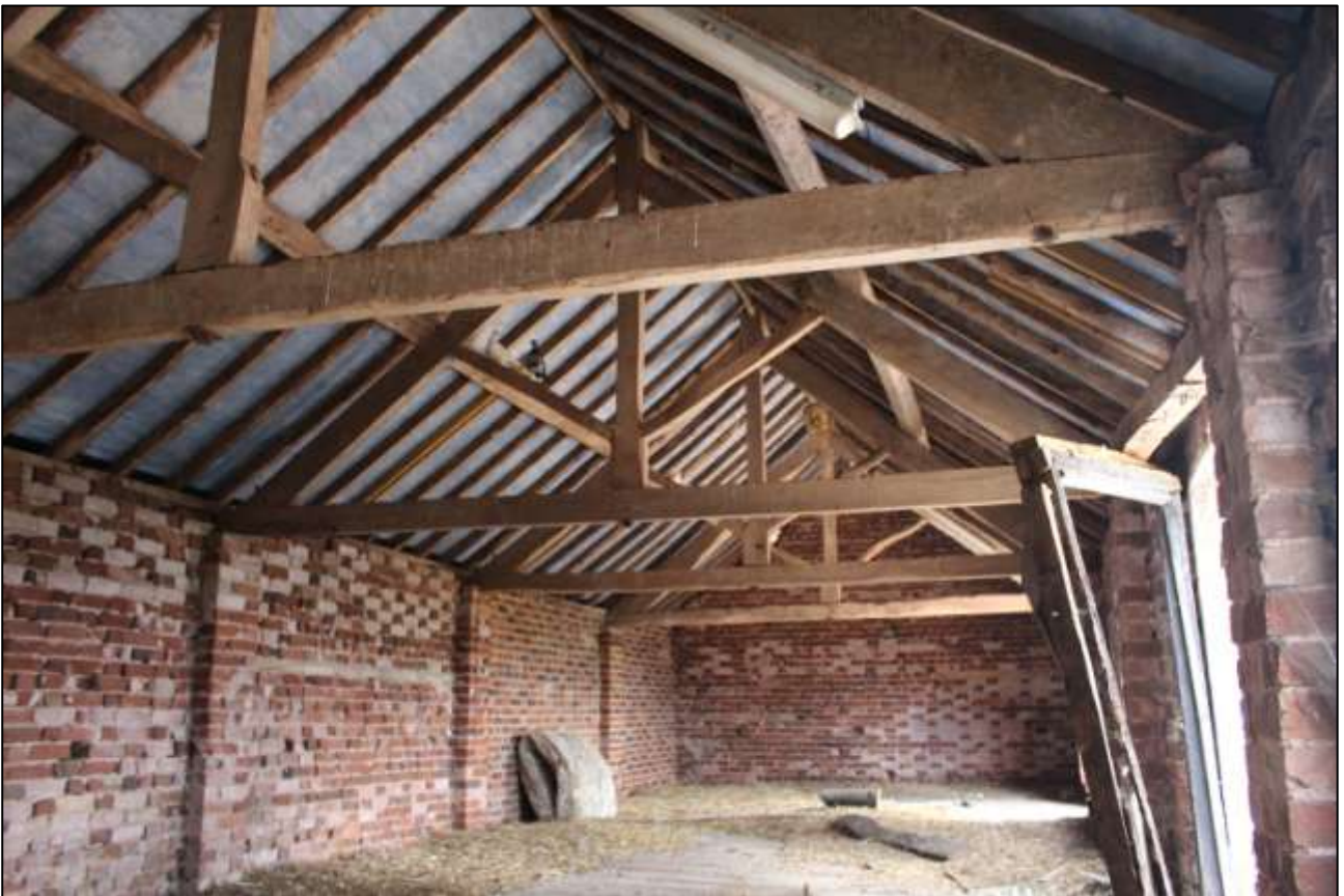
AS ABOVE, SHOWING MORE DETAIL OF THE ROOF TRUSSES.
