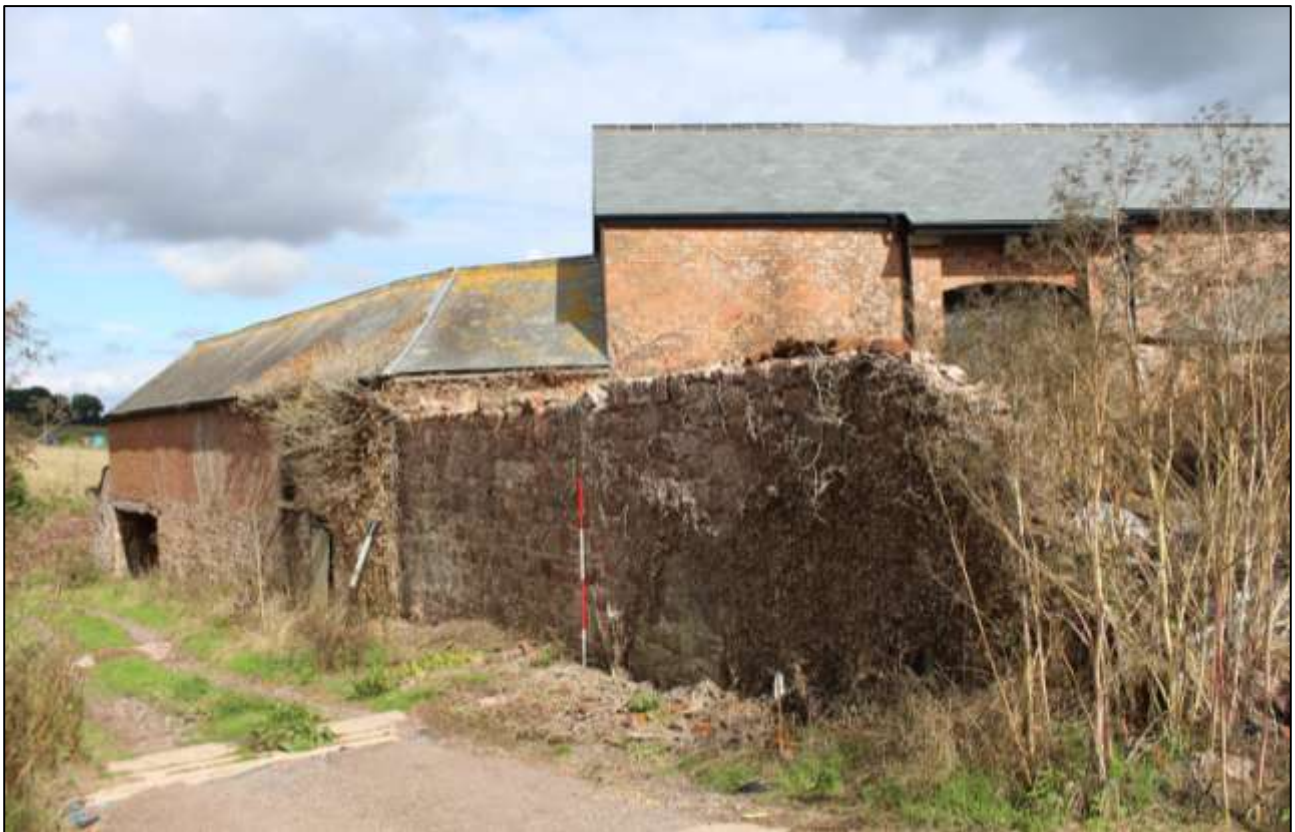
B6 EXTERIOR AND YARD WALL; VIEWED FROM THE WEST (SCALE 2M).
