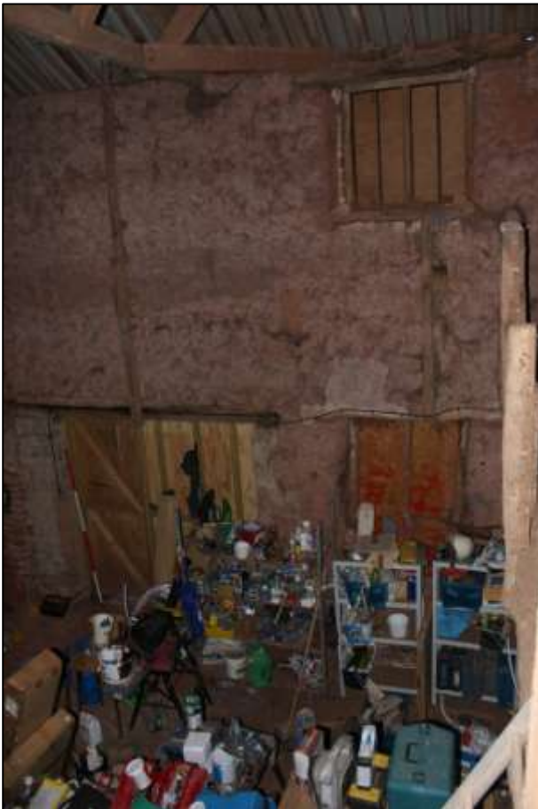
LEFT: B1 INTERIOR, NORTH WALL; VIEWED FROM THE SSE.
