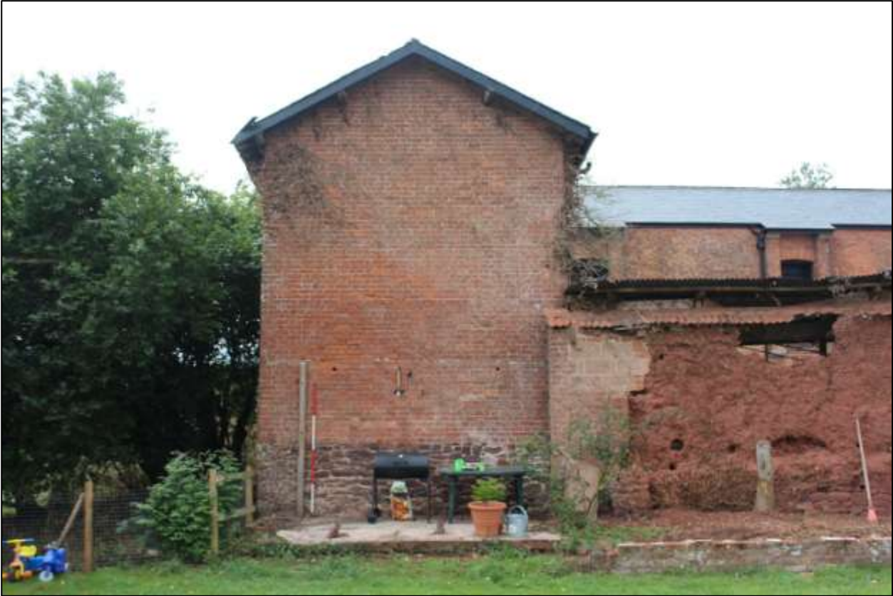
B7 EXTERIOR, EAST GABLE WALL; VIEWED FROM THE EAST (SCALE 2M).
