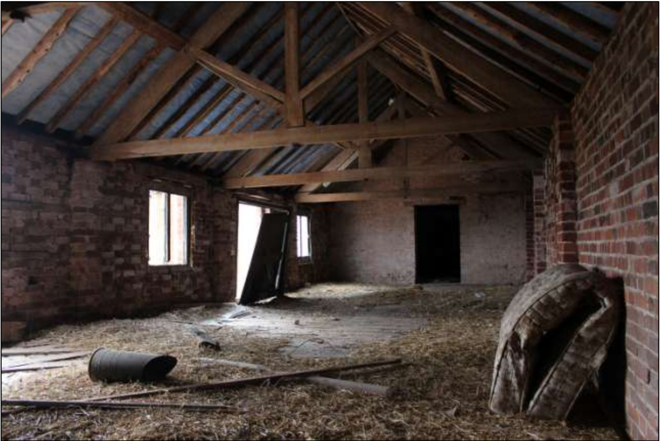
B4 FF INTERIOR; VIEWED FROM THE NORTH-EAST.
