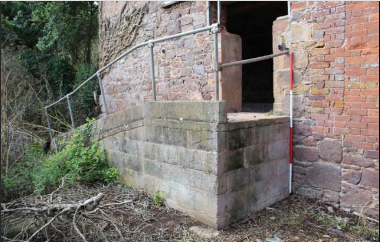
B6 EXTERIOR, SOUTH WALL, DETAIL OF THE CONCRETE RAMP PROVIDING ACCESS TO THE FORCED DOORWAY; VIEWED FROM THE SOUTH-EAST (SCALE 2M).
