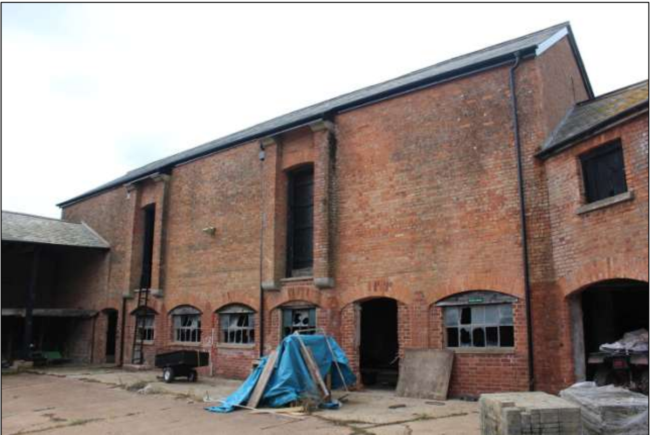
B6 EXTERIOR, EAST ELEVATION; VIEWED FROM THE NORTH-EAST (SCALE 2M).
