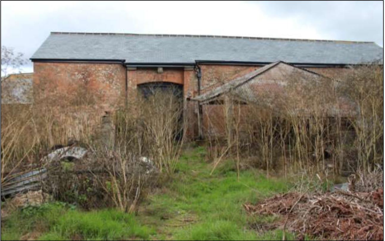
B6 EXTERIOR WITH B8, WEST WALL; VIEWED FROM THE WEST.
