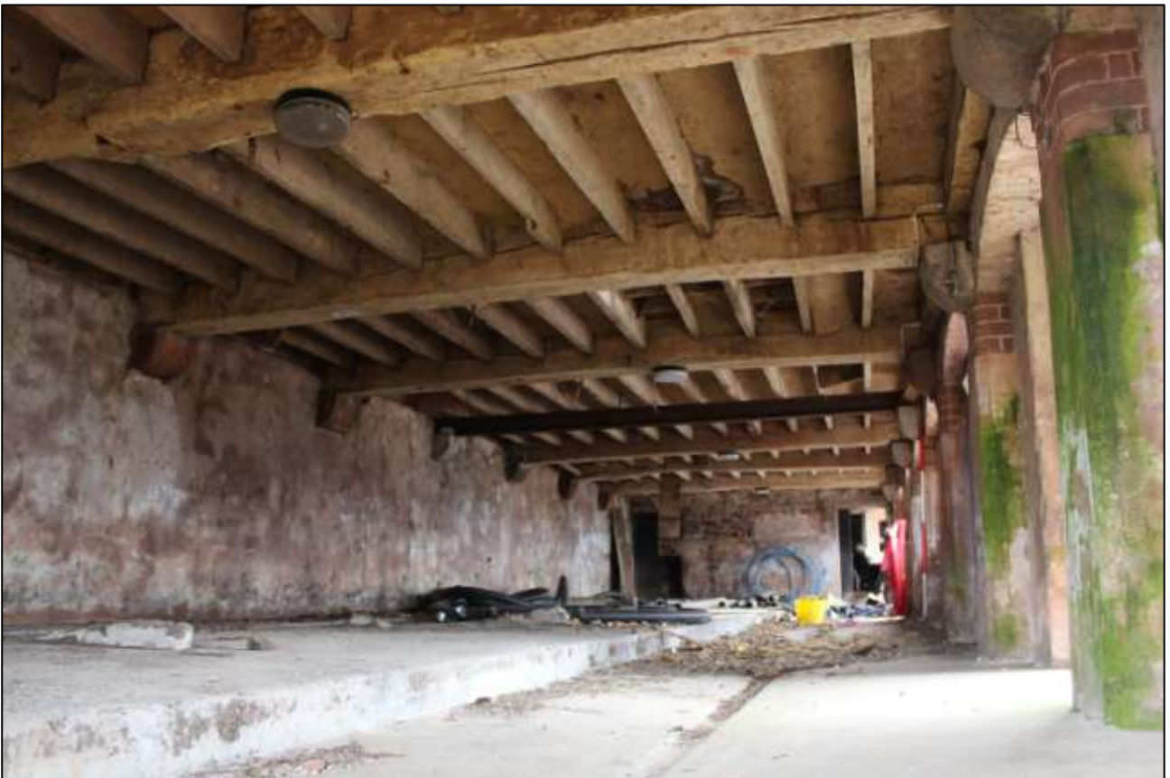
AS ABOVE, DETAIL OF THE CEILING.
