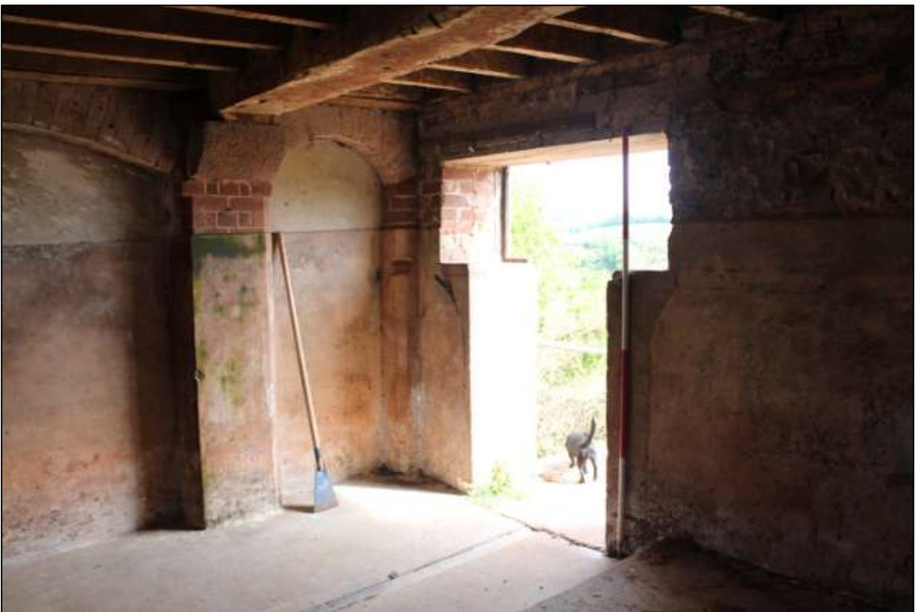
AS ABOVE; VIEWED FROM THE NORTH-WEST.
