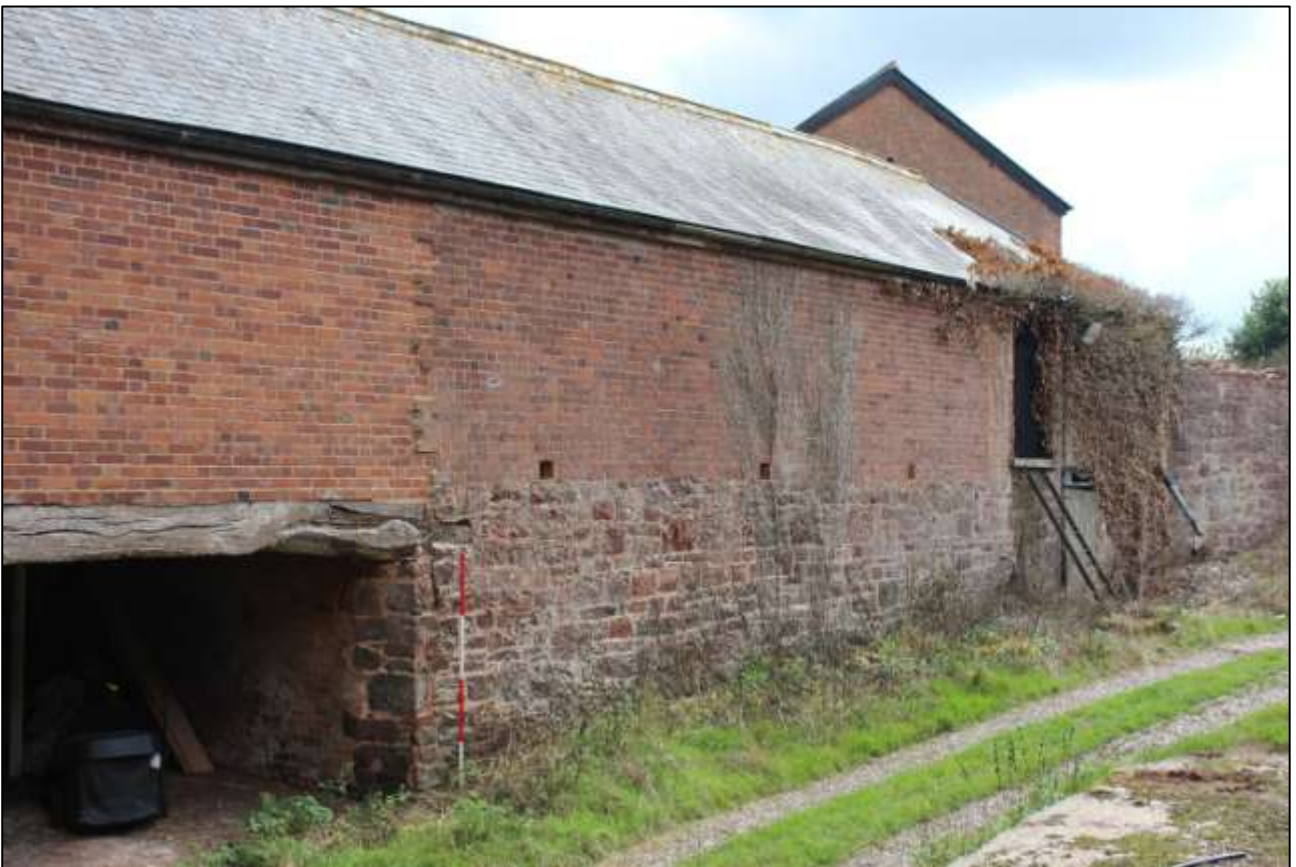
B4 EXTERIOR, NORTH-WEST WALL; VIEWED FROM THE NORTH (SCALE 2M).
