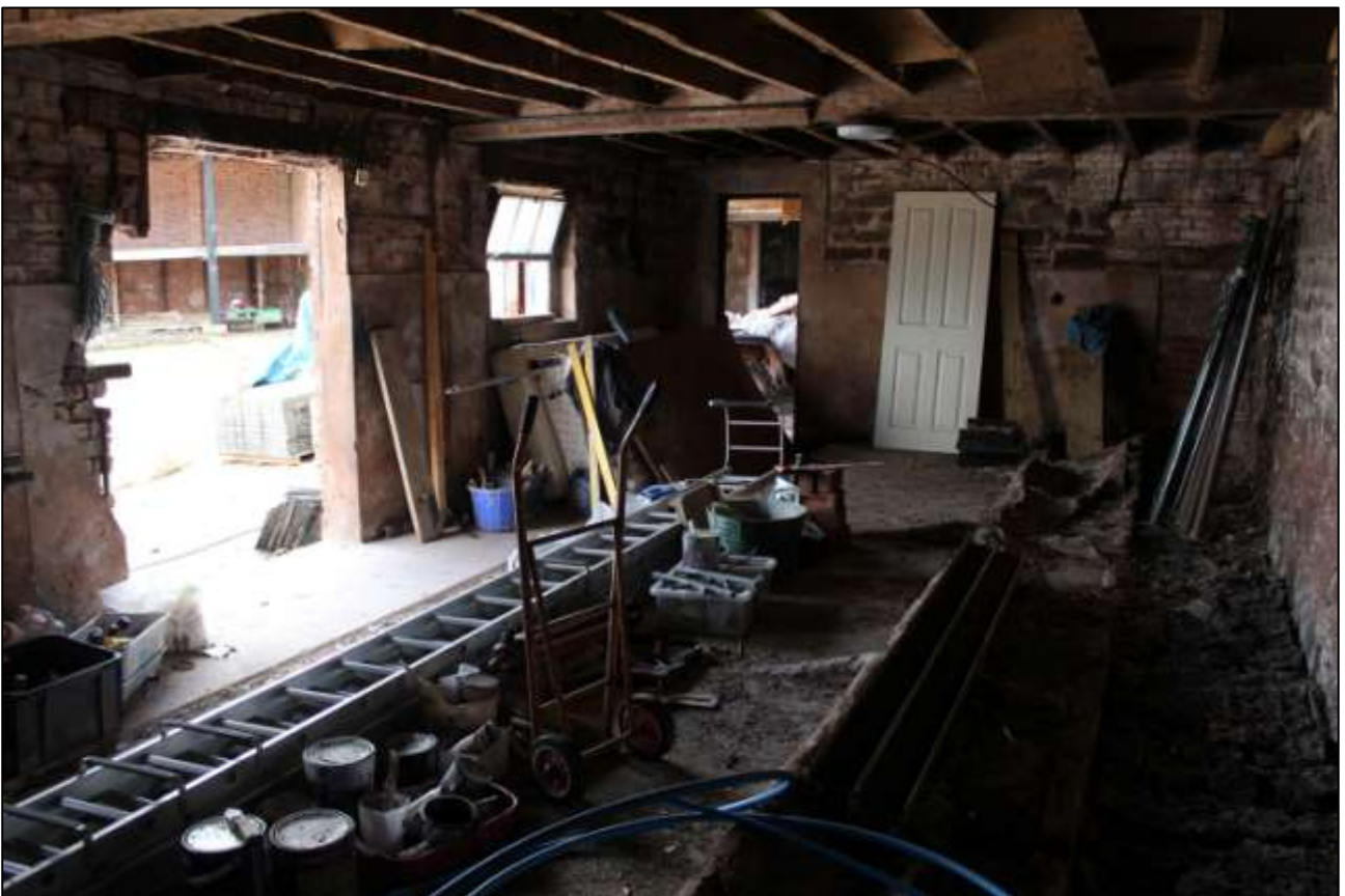
B4A INTERIOR; VIEWED FROM THE NORTH-EAST.
