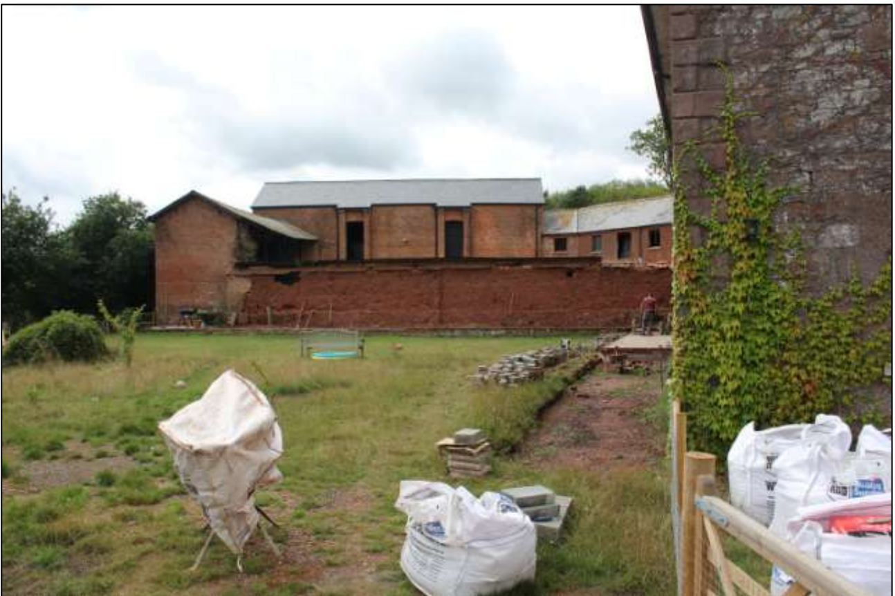
THE BRICK BARN (B6 TO CENTRE) AS VIEWED FROM THE GARDEN OF THE FARMHOUSE; VIEWED FROM THE EAST.
