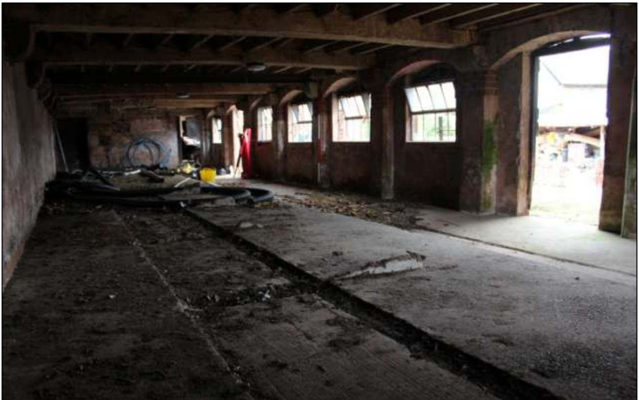
B6 GF INTERIOR; VIEWED FROM THE SSW (SCALE 2M).
