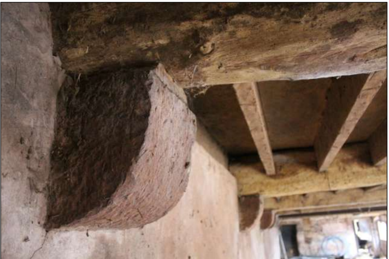
B6 GF INTERIOR, DETAIL OF ONE OF THE CORBELS SUPPORTING THE BEAMS; VIEWED FROM THE SOUTH.
