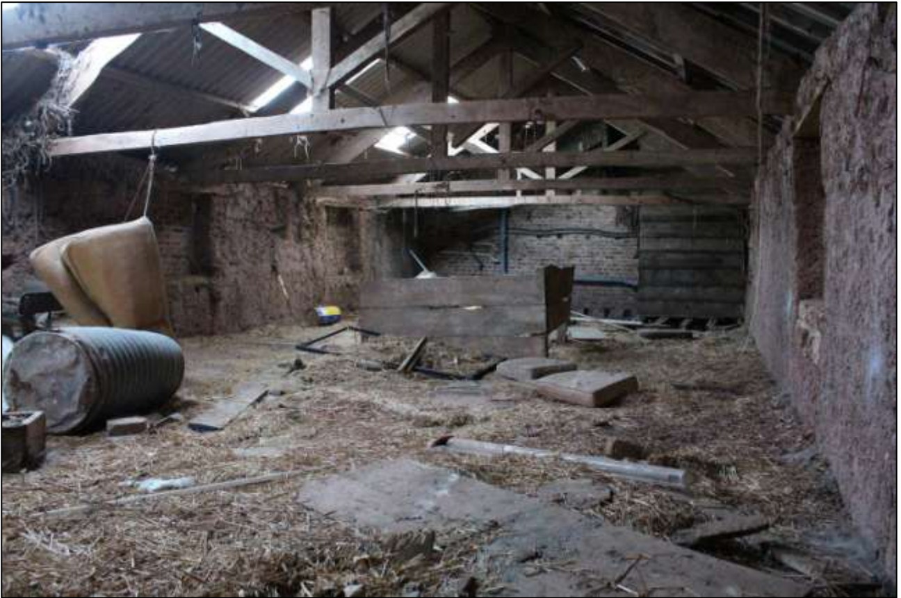
B2 FF INTERIOR; VIEWED FROM THE NNW.
