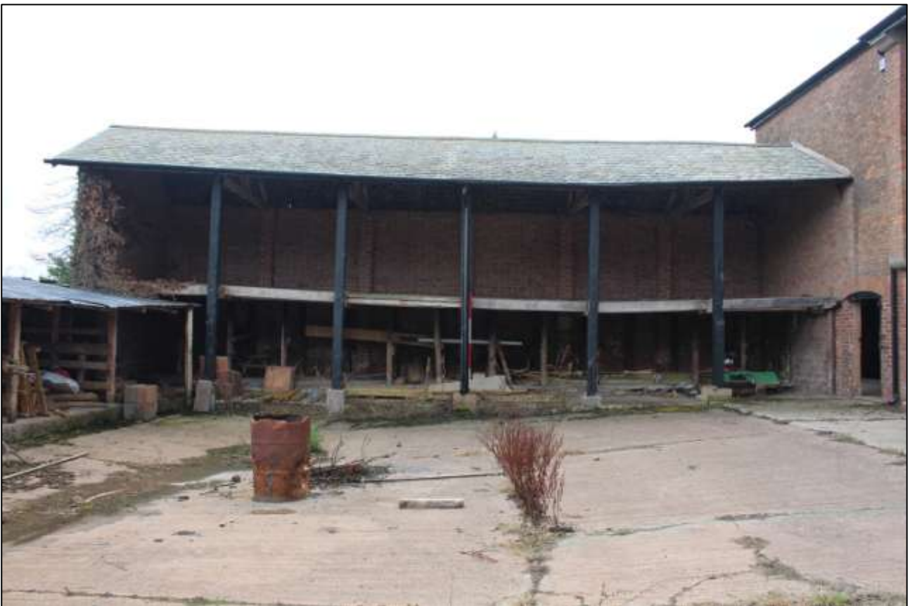
B7 EXTERIOR, NORTH OPEN-FRONTED ELEVATION; VIEWED FROM THE NORTH (SCALE 2M).
