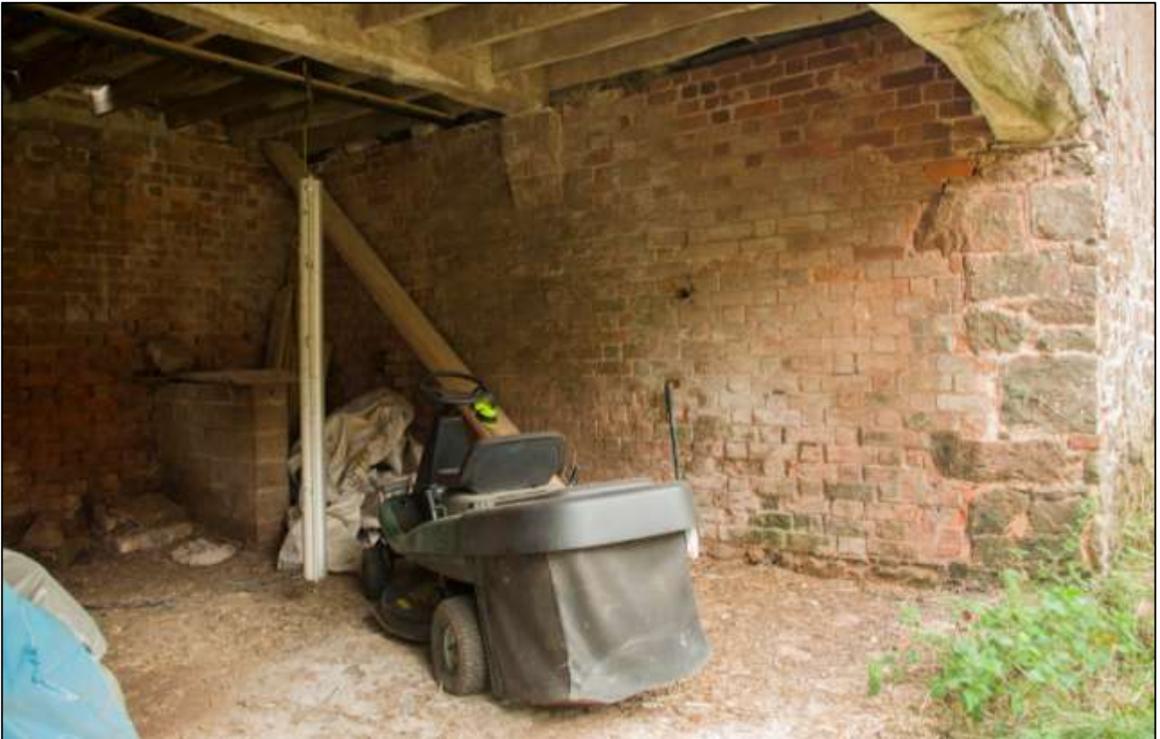
B4B INTERIOR; VIEWED FROM THE NORTH.
