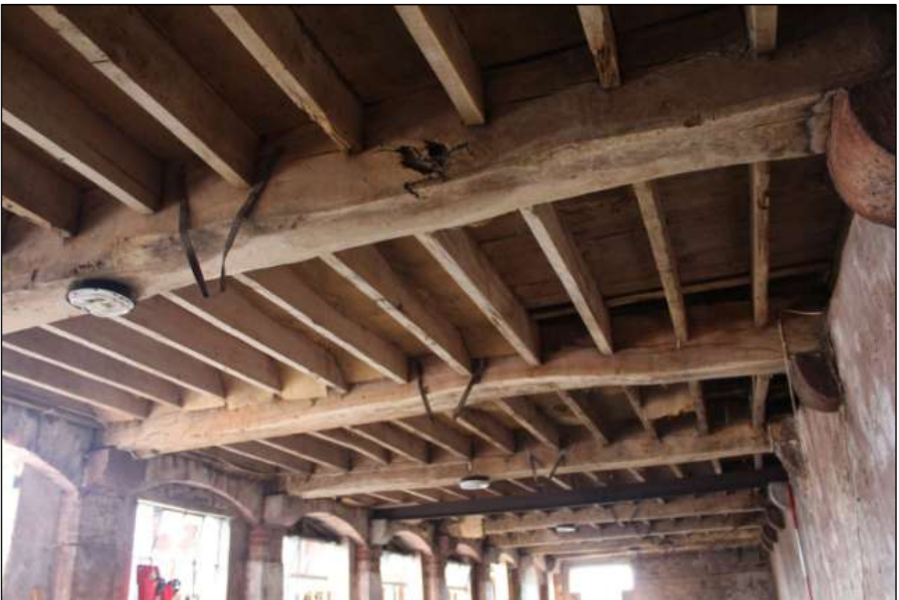
AS ABOVE, WITH DETAIL OF THE ROOF STRUCTURE.
