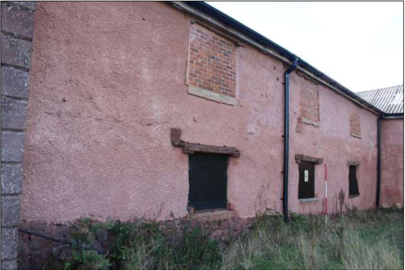
B2 EXTERIOR, EAST ELEVATION; VIEWED FROM THE SOUTH-EAST (SCALE 2M).
