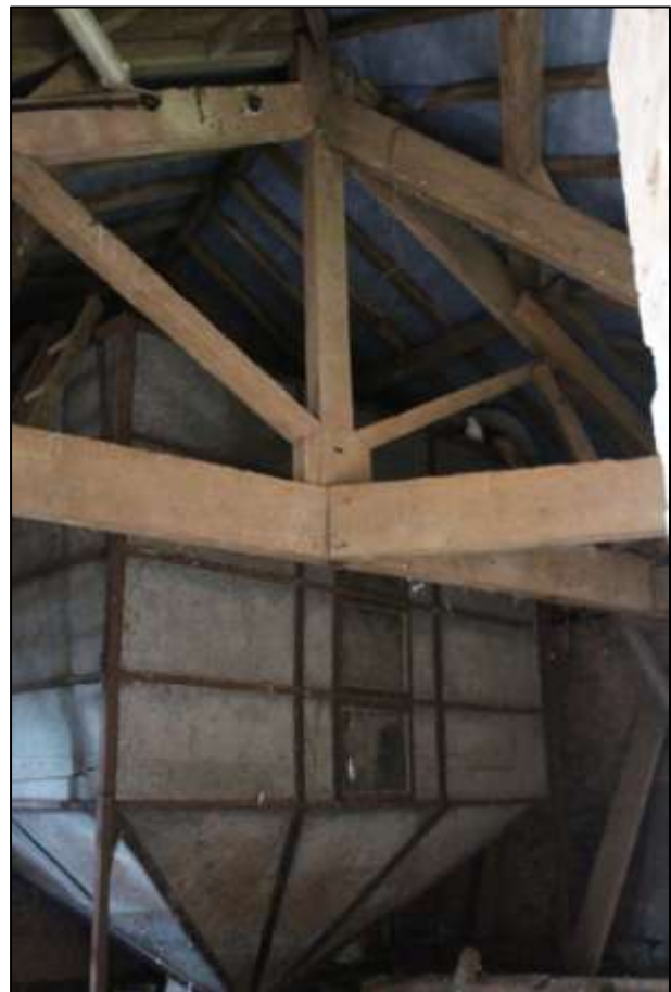
RIGHT: B5 FF INTERIOR, DETAIL OF THE FEED HOPPER AND THE KINGPOST ROOF STRUCTURE; VIEWED FROM THE NORTH-EAST.
