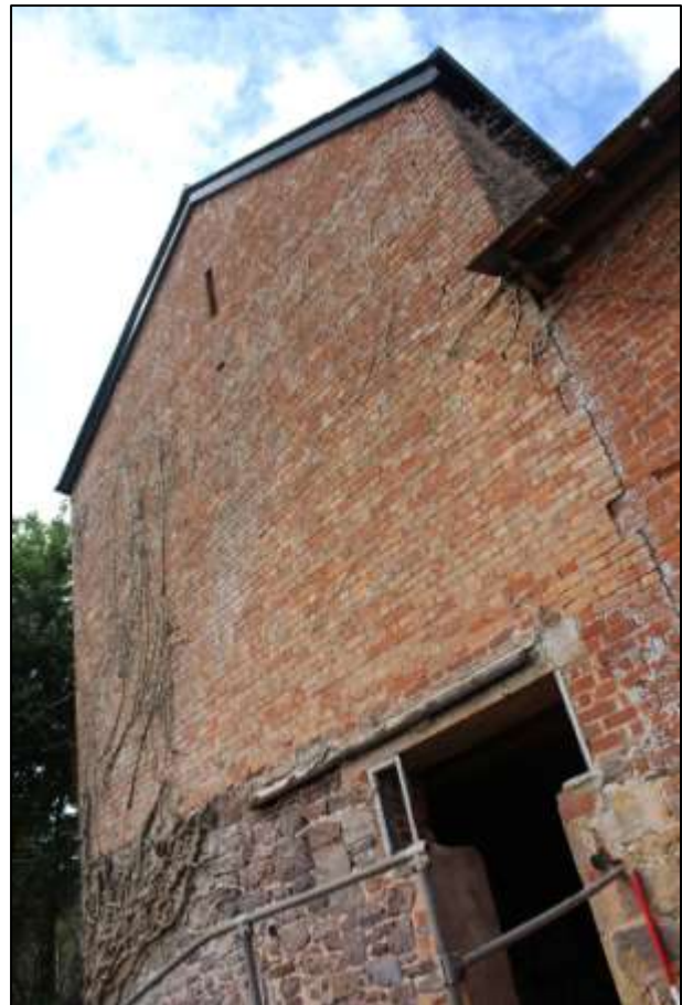
RIGHT: B6 EXTERIOR, SOUTH WALL, SHOWING THE TALL BLIND ELEVATION; VIEWED FROM THE SOUTH-EAST (SCALE 2M).
