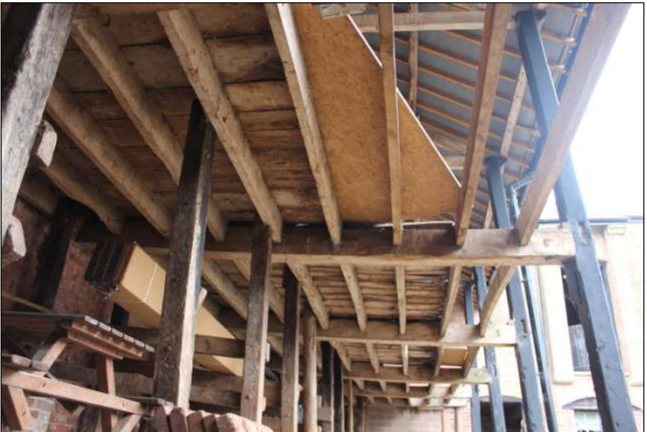
AS ABOVE, SHOWING DETAIL OF THE CEILING.
