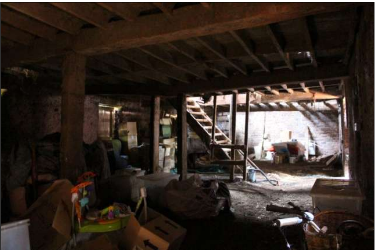
AS ABOVE; VIEWED FROM THE NORTH-WEST.
