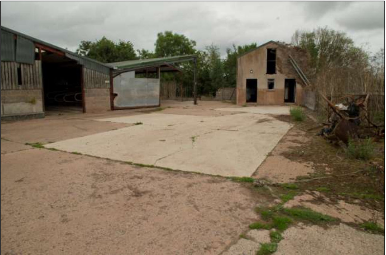
AS ABOVE, SHOWING B12; VIEWED FROM THE SOUTH-WEST.
