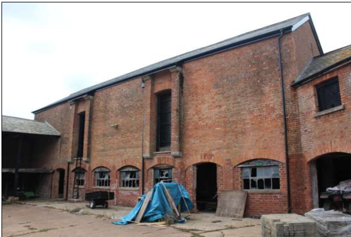
FIGURE 21: THE EAST ELEVATION OF THE B6 THE THRESHING BARN; VIEWED FROM THE NORTH-EAST (SCALE 2M).
