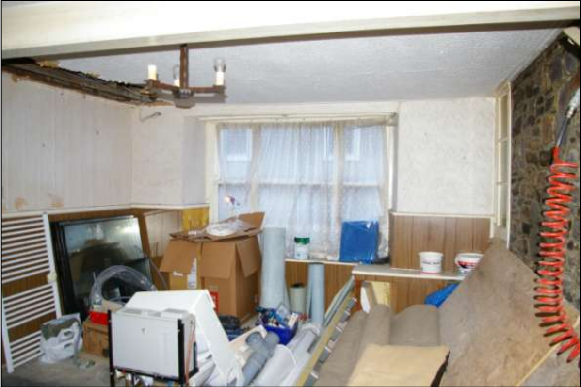
INTERNAL SOUTH WALL OF GR1 SHOWING SASH WINDOW; VIEWED FROM THE NORTH-WEST (NO SCALE).
