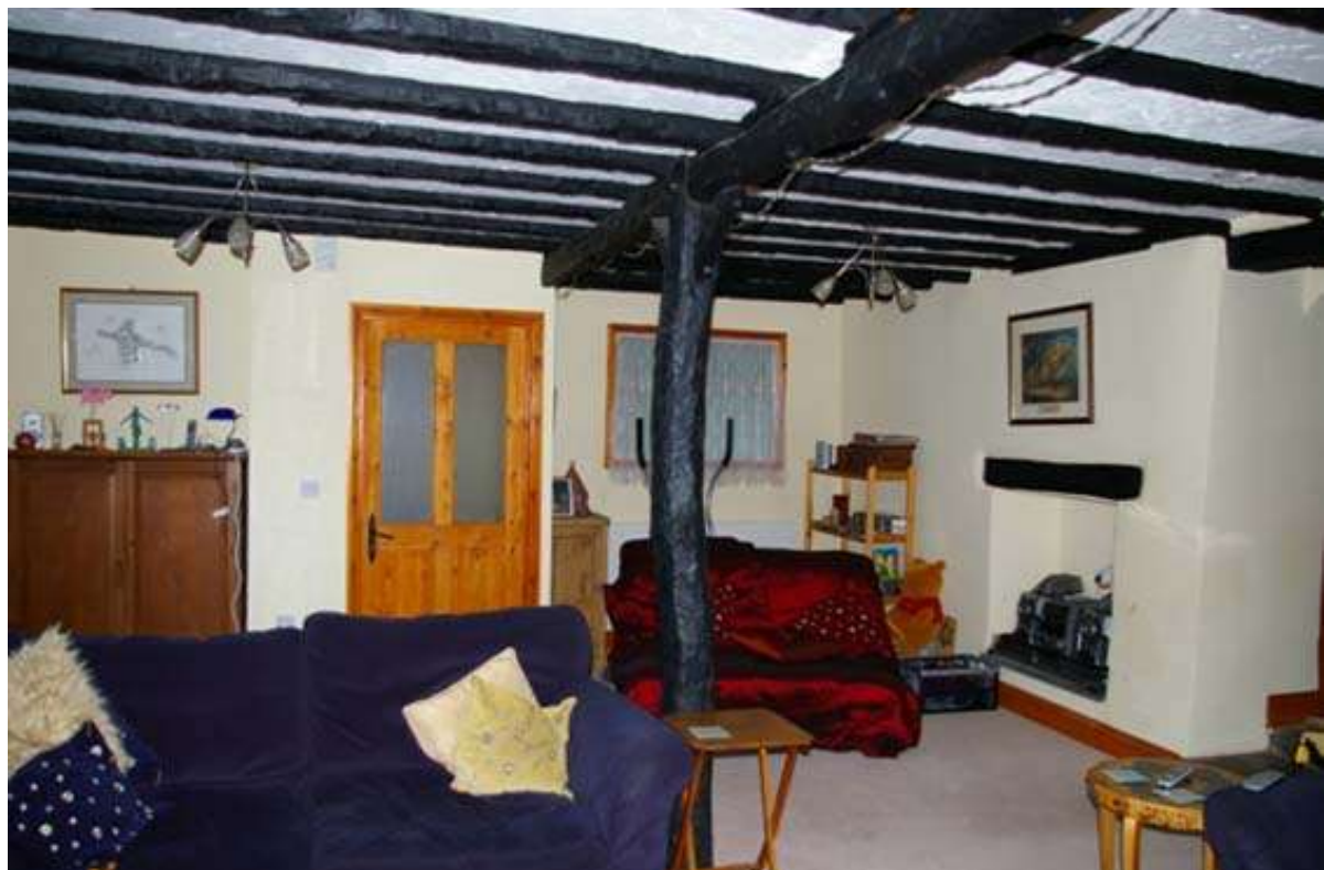
INTERNAL WEST WALL OF GR4; VIEWED FROM THE EAST-SOUTH-EAST (NO SCALE).
