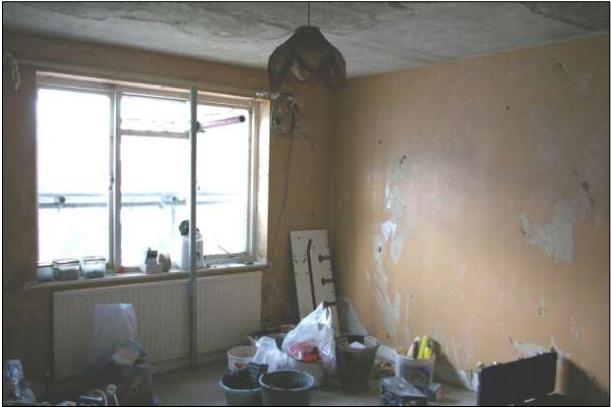
INTERNAL NORTH AND EAST WALLS OF FR4; VIEWED FROM THE SOUTH-WEST (NO SCALE).
