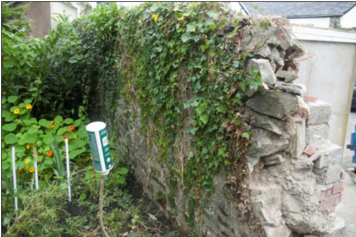
WALL {004}, EAST ELEVATION OBLIQUE;; VIEWED FROM THE NORTH-EAST (NO SCALE).
