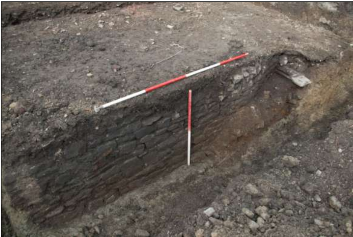
WALL {018}, SOUTH FACING ELEVATION, OBLIQUE; VIEWED FROM THE SOUTH-WEST (1M & 2M SCALES).
