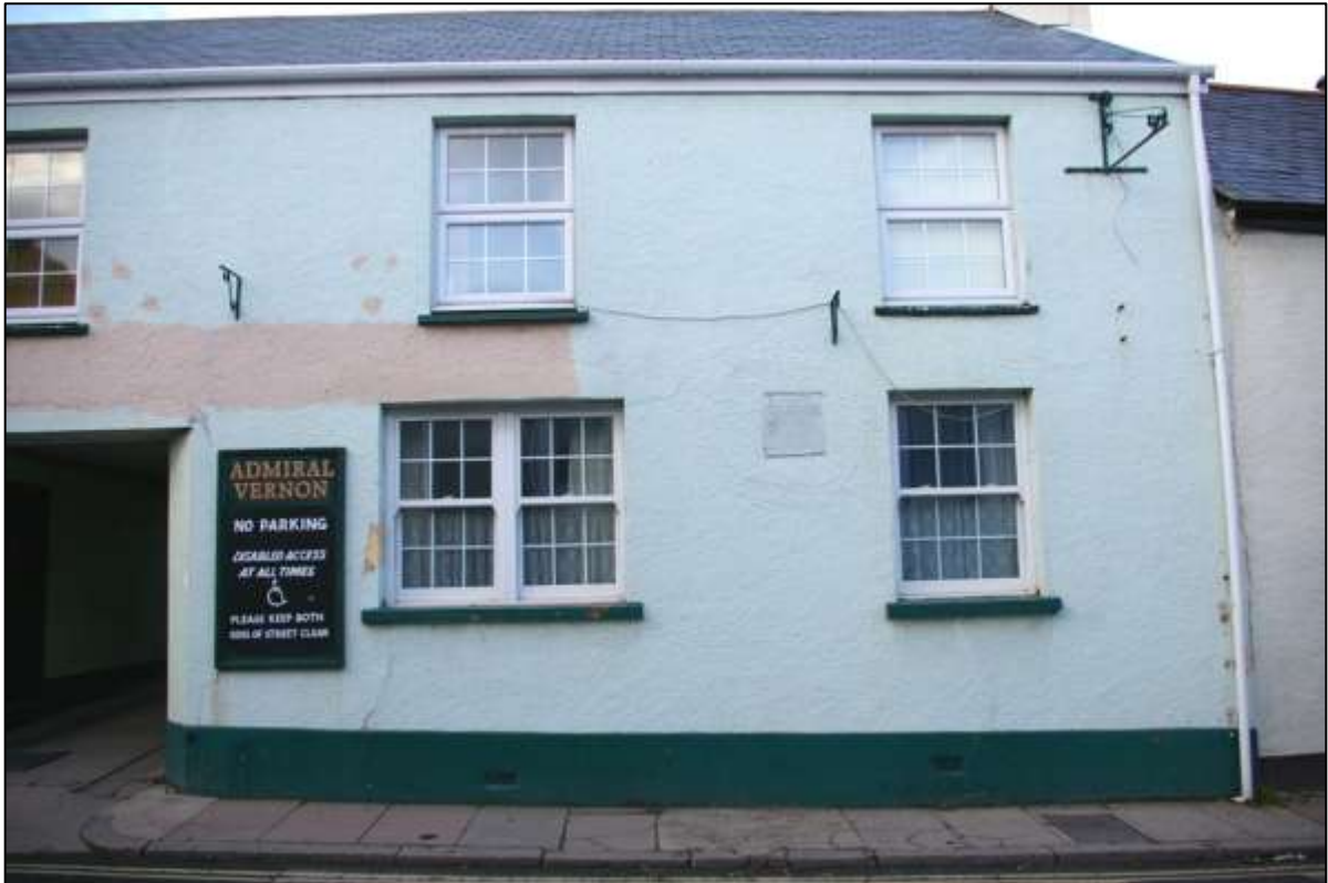
SOUTH ELEVATION, SHOWING MODERN DOUBLE-GLAZED WINDOWS, INCLUDING SASH TO THE GROUND FLOOR; VIEWED FROM THE SOUTH.
