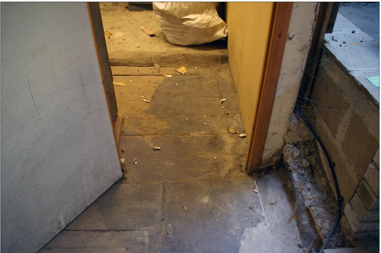
60. B1 FF R1A, VIEW THROUGH D17 INTO R1A SHOWING THE HISTORIC FLOORBOARDS (S5); VIEWED FROM THE EAST.
