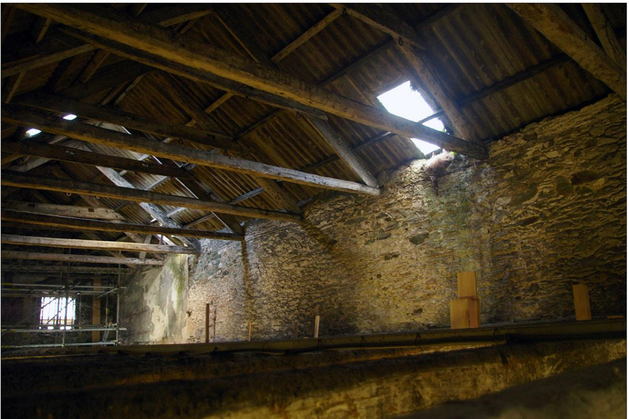
124. AS ABOVE, WITH DETAIL OF THE EAST WALL OF B2; VIEWED FROM THE SOUTH-WEST.
