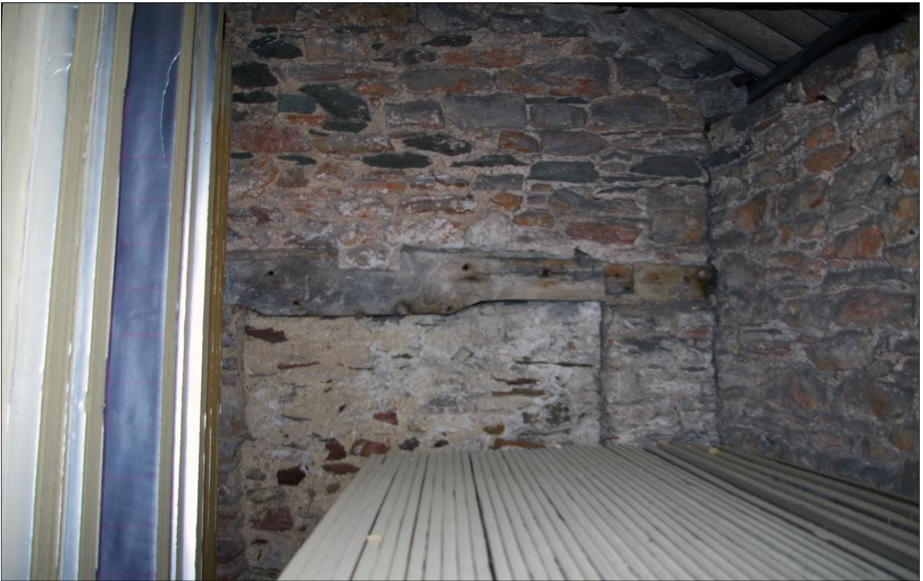
185. B3 FF INTERIOR, THE NORTH WALL SHOWING BO46 WITH UPSIDE-DOWN YOKED LINTEL; VIEWED FROM THE SOUTH.
