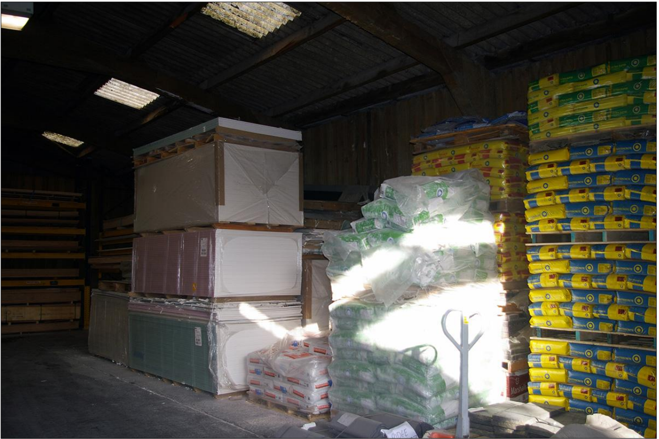
192. AS ABOVE, THE CONCEALED EAST WALL OF B4 (WALL OF THE ADJOINING PROPERTY); VIEWED FROM THE SOUTH-WEST.
