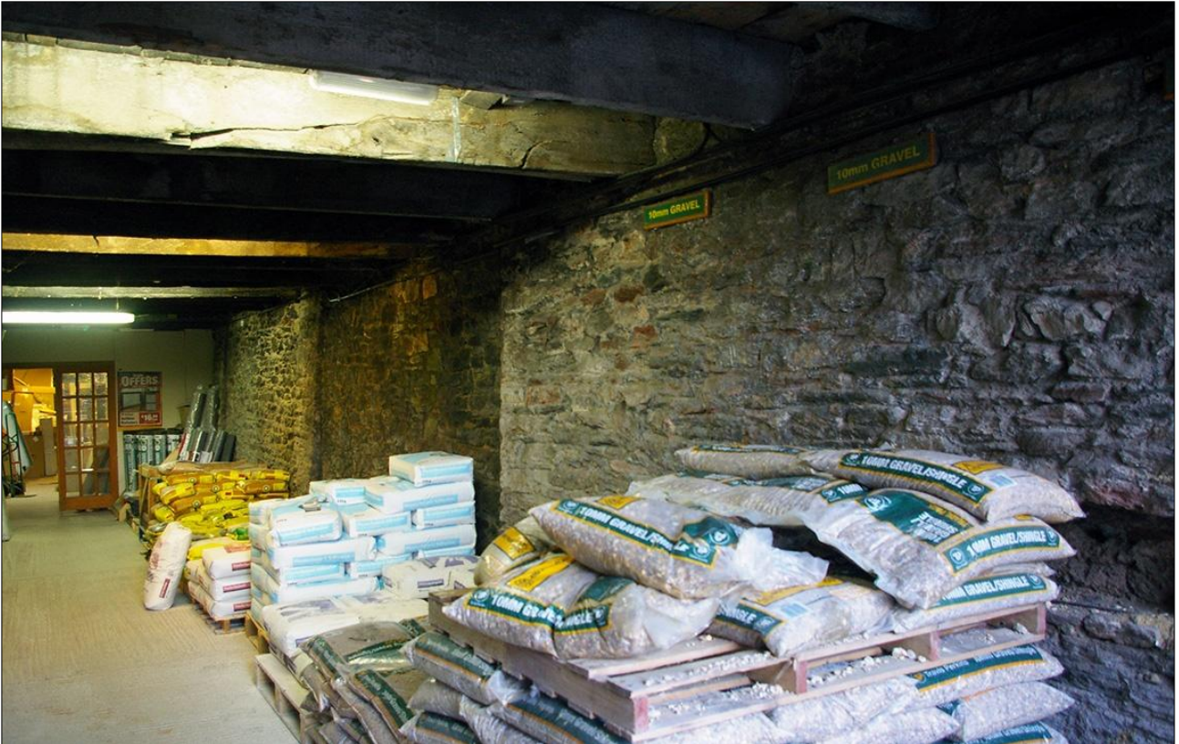
145. B3 GF INTERIOR, THE EAST WALL; VIEWED FROM THE SSW.
