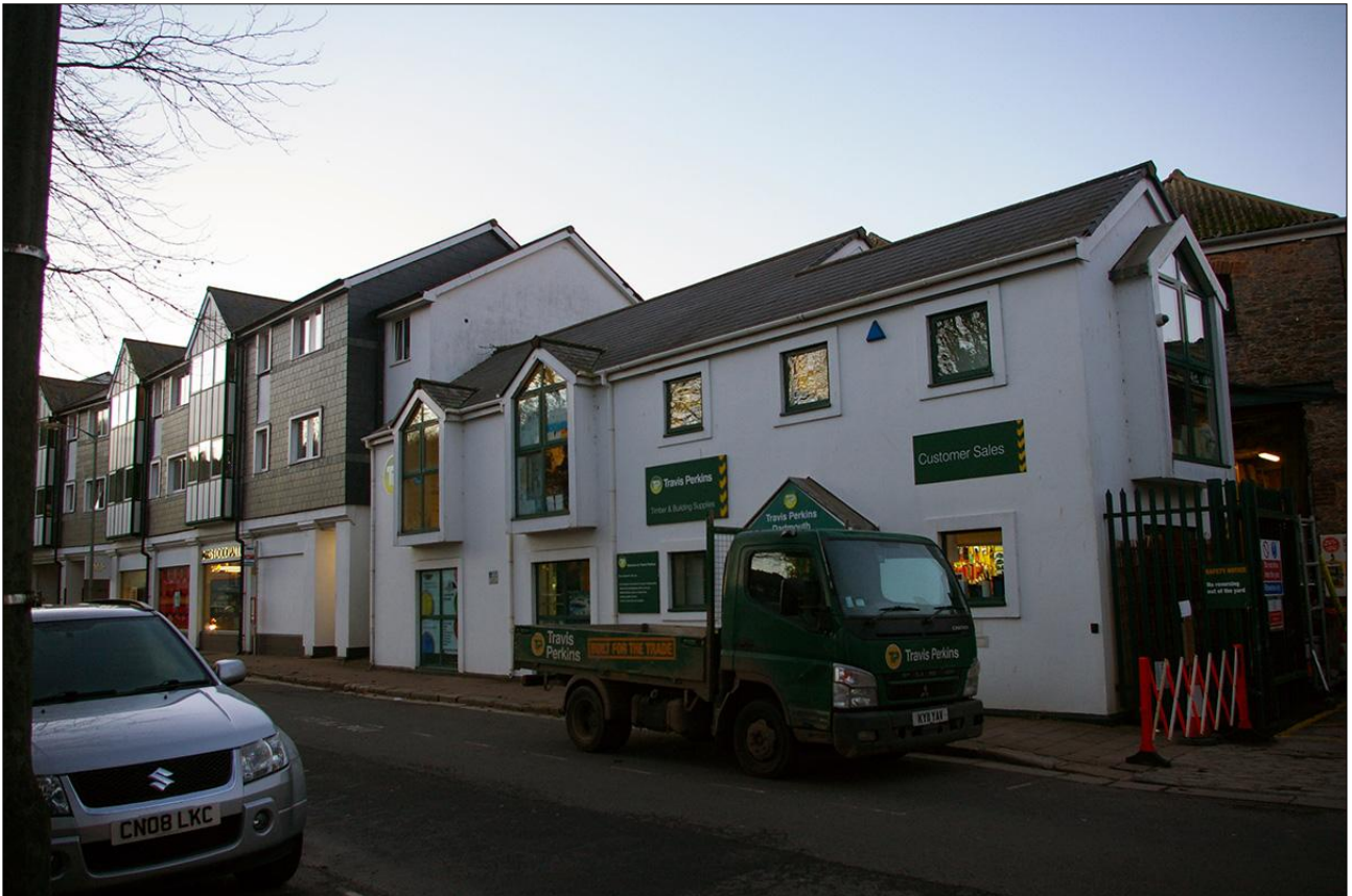
194. THE SOUTH ELEVATION OF THE 1990S TRAVIS PERKINS BUILDING; VIEWED FROM THE SOUTH-EAST.
