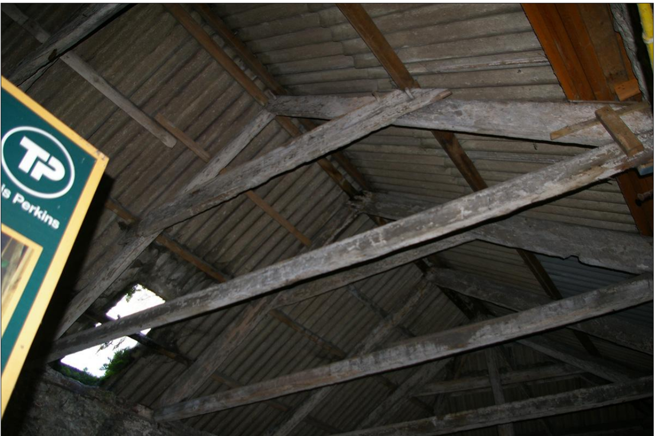
133. AS ABOVE, THE SOUTHERN HALF OF THE ROOF; VIEWED FROM THE NNW.
