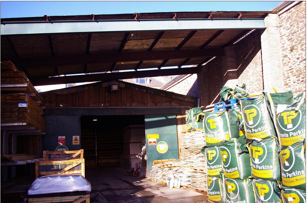
189. B4; VIEWED FROM THE SOUTH.
