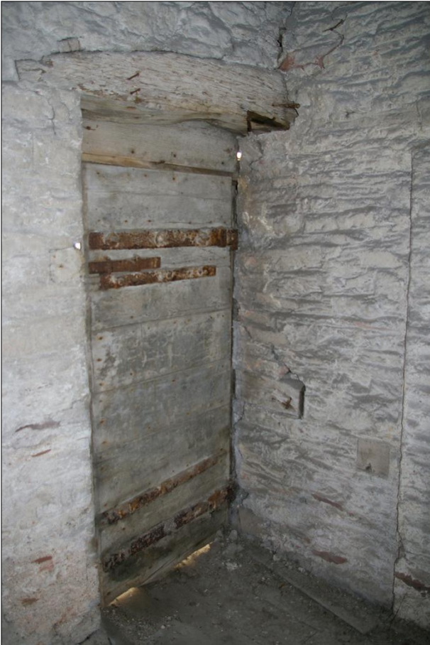
86. B1 FF R3, DETAIL OF D21 SHOWING ITS YOKED LINTEL AND THE RECESS BUILT INTO THE EAST WALL TO TAKE THE DOOR; VIEWED FROM THE SOUTH-WEST.
