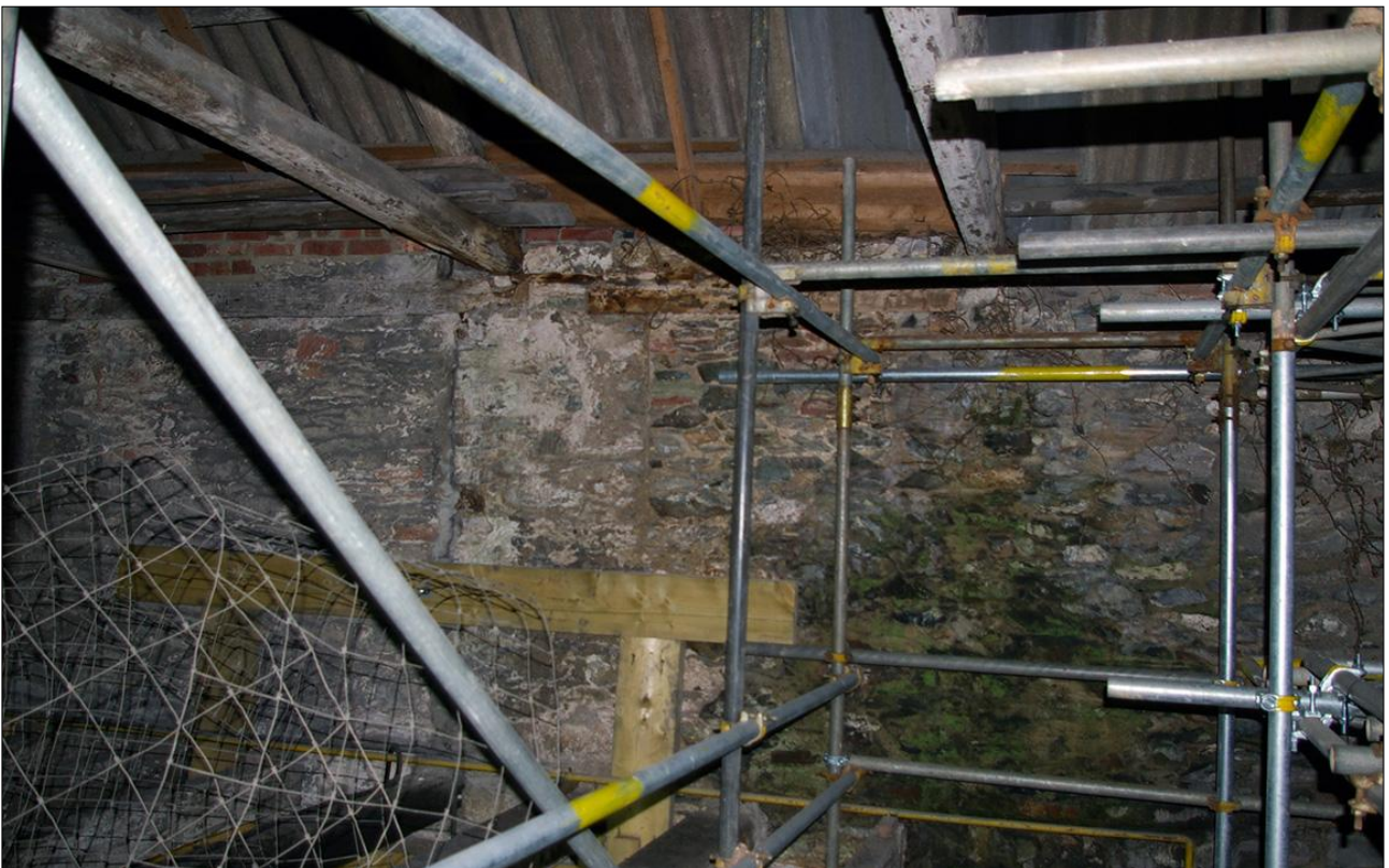
16. THE EAST WALL OF B1 AT ITS NORTHERN END AT SF LEVEL; VIEWED FROM THE WEST.
