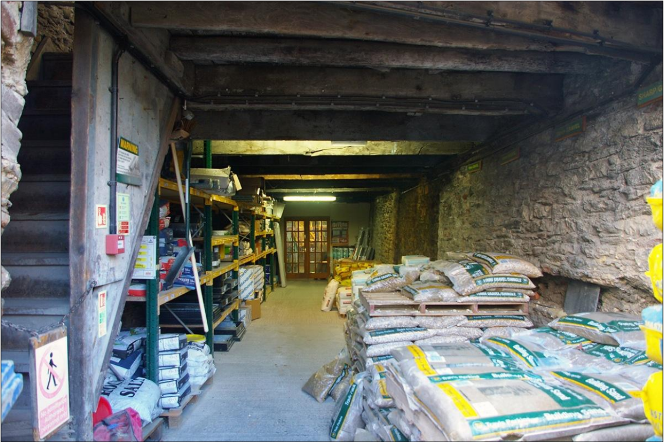
143. THE GF INTERIOR OF B3; VIEWED FROM THE SOUTH.
