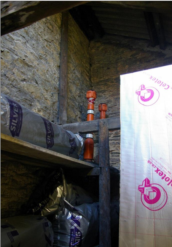
186. LEFT: B3 FF INTERIOR, THE NORTH WALL ABUTTING B2; VIEWED FROM THE SSE.
