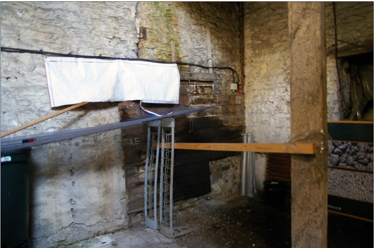
56. AS ABOVE, SHOWING THE REMNANT WOODEN PANELLING (S7) IN THE SOUTH-EAST CORNER; VIEWED FROM THE NORTH-WEST.
