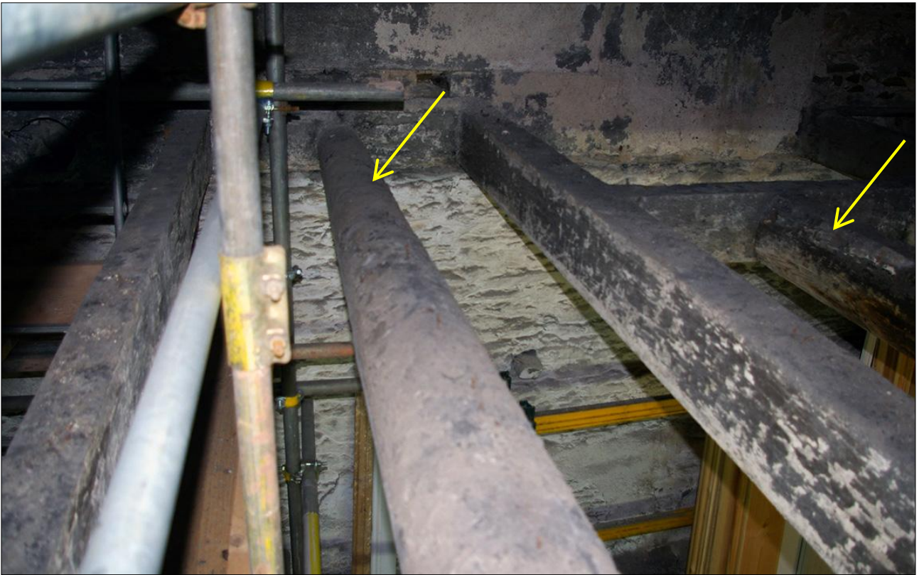
127. B2 SF INTERIOR, SHOWING THE BEAMS AND RE-USED SHIPS TIMBERS S22 (INDICATED); VIEWED FROM THE WEST.
