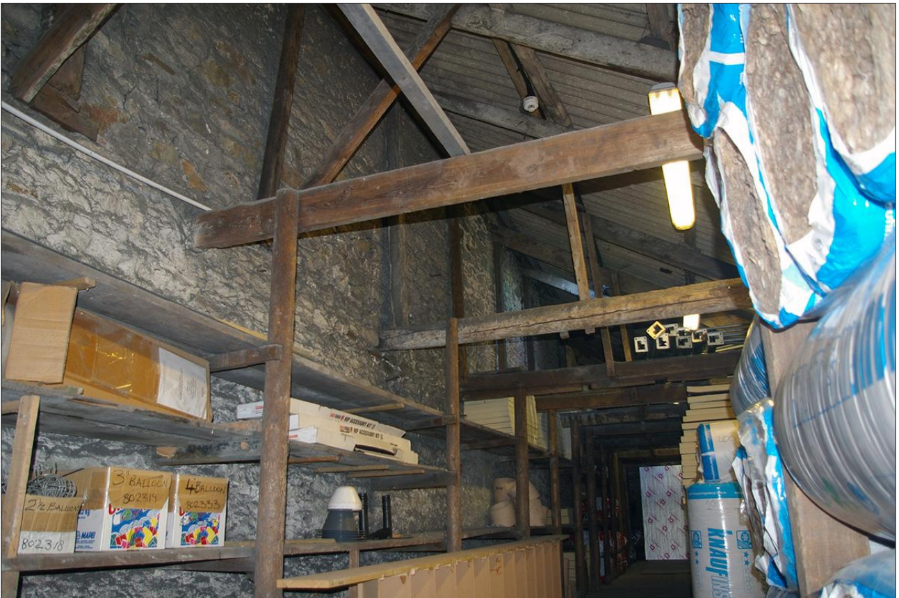
178. B3 FF INTERIOR, SHOWING THE ROOF STRUCTURE; VIEWED FROM THE SSE.
