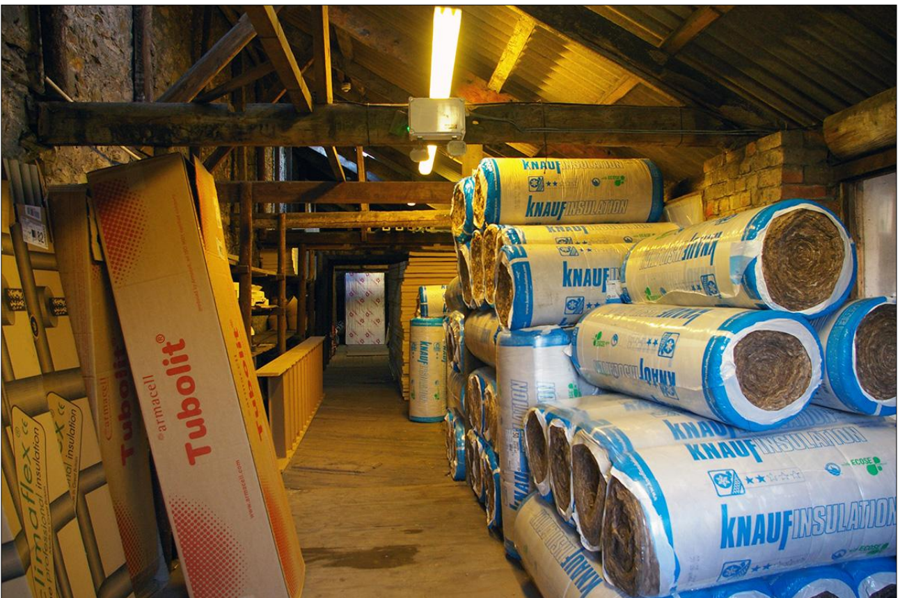
173. B3 FF INTERIOR; VIEWED FROM THE SOUTH.
