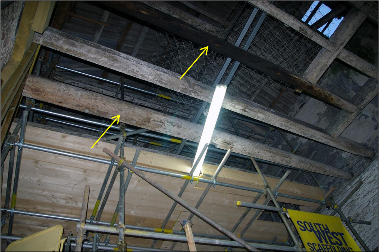
115. B2 FF INTERIOR, SHOWING THE SF BEAMS AND RE-USED SHIPS TIMBERS S22 (INDICATED); VIEWED FROM THE SSW.
