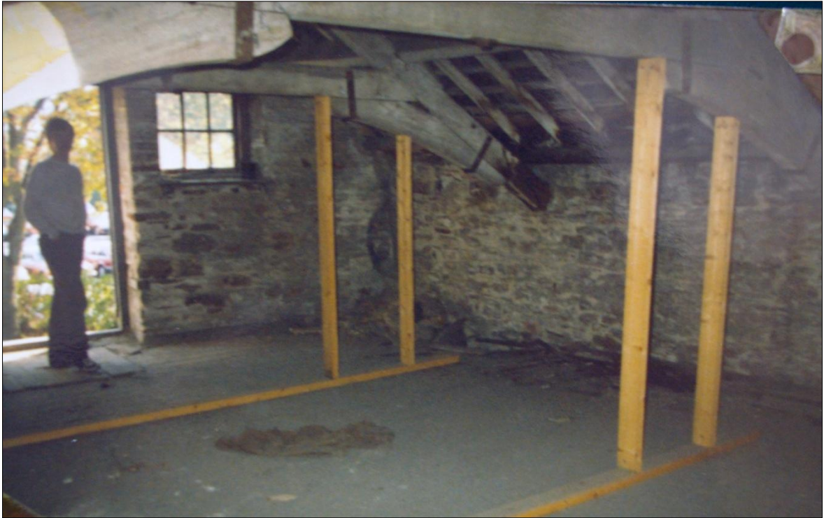
FIGURE 11: THE ROOF SPACE IN THE DEMOLISHED 19 TH CENTURY BUILDING (PRIVATE COLLECTION).
