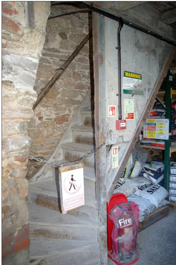
146. B3 GF INTERIOR, THE STAIRS (S3) TO THE FIRST FLOOR; VIEWED FROM THE SOUTH-EAST.
