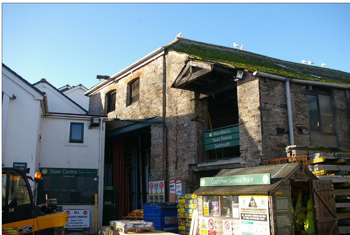
FIGURE 26: THE SOUTH ELEVATION OF B2 AND B3; VIEWED FROM THE SOUTH-EAST.
