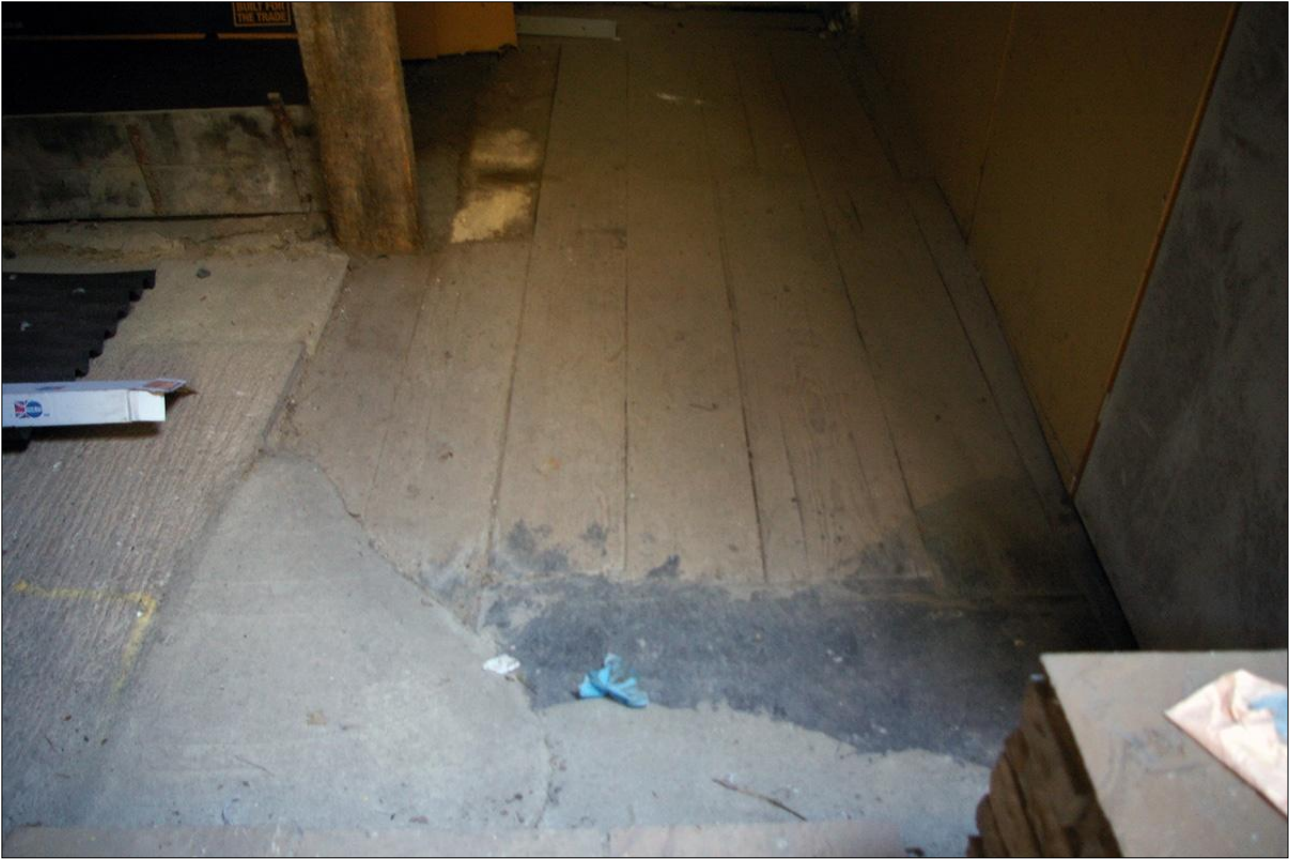
59. B1 FF R1, VIEW OF THE SURVIVING HISTORIC FLOORBOARDS (S5) IN FRONT OF D16; VIEWED FROM THE NORTH.
