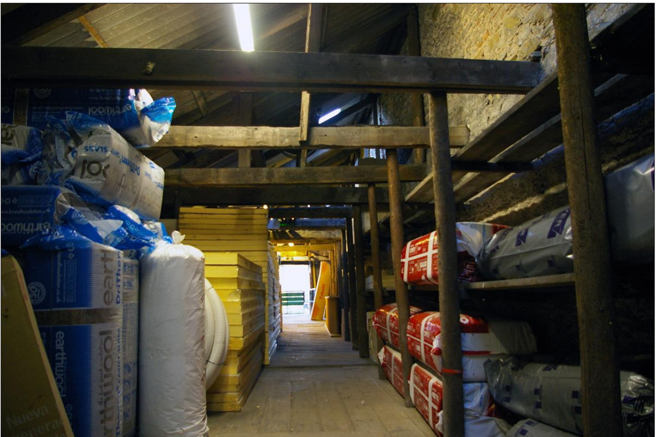
180. B3 FF INTERIOR; VIEWED FROM THE NORTH.
