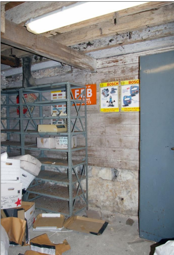
62. B1 FF R1A, SHOWING THE WOODEN PANELLING (S8) IN THIS ROOM; VIEWED FROM THE NORTH-EAST.
