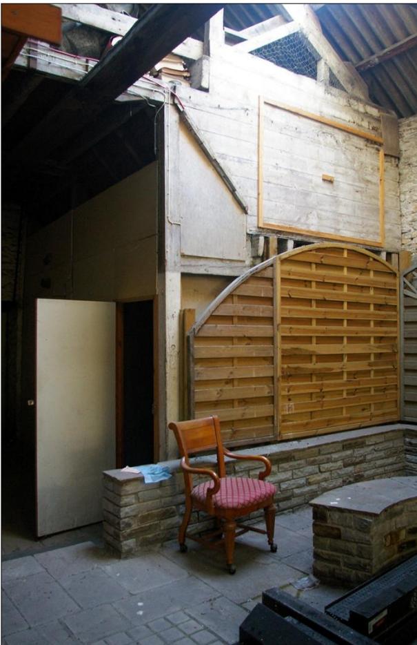
53. LEFT: AS ABOVE; VIEWED FROM THE NORTH-EAST.
