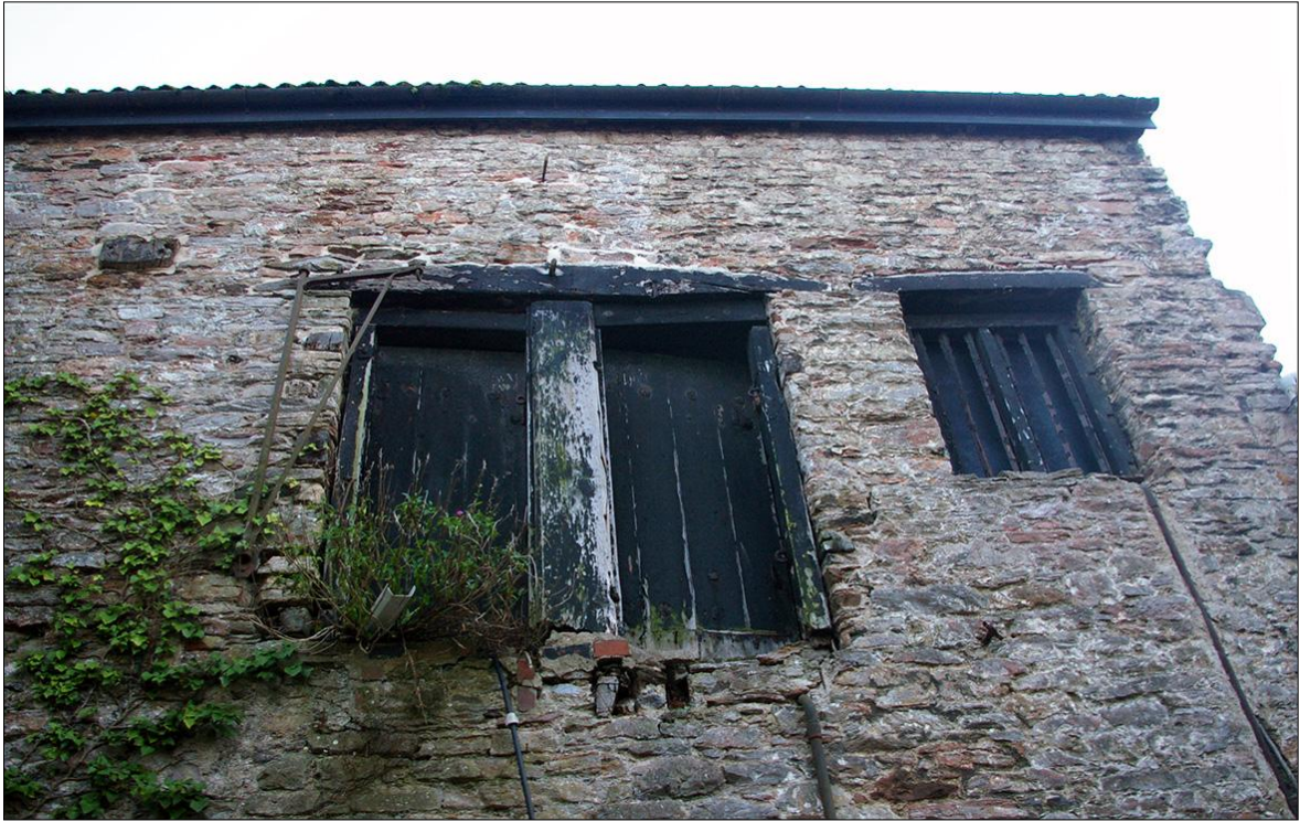
FIGURE 24: THE NORTH ELEVATION OF B1, SHOWING W11 AND DOUBLE-DOOR D21/D22; VIEWED FROM THE NORTH.
