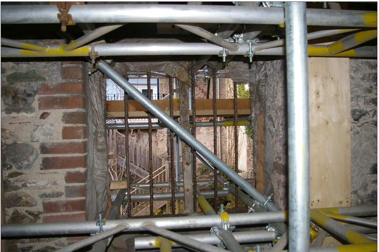
112. B2 FF INTERIOR, NORTH WALL, SHOWING W12; VIEWED FROM THE SOUTH.
