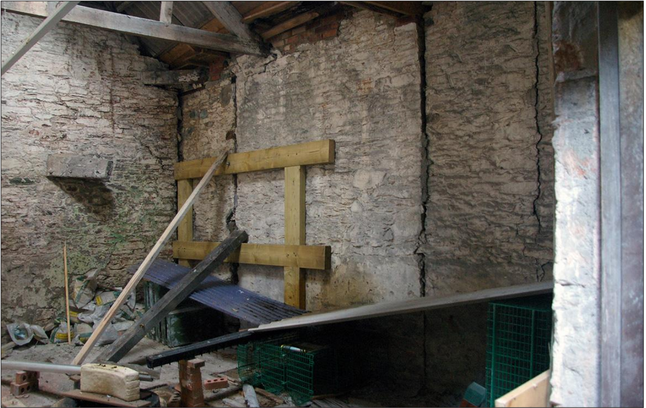
79. B1 FF R2, THE EAST WALL AND ITS BUILD LINES; VIEWED FROM THE SOUTH-EAST.
