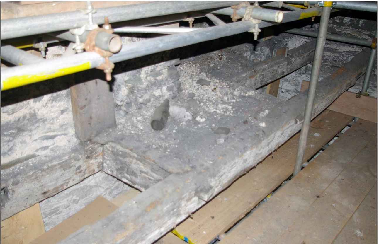
126. AS ABOVE, SHOWING THE REINFORCED BASE FOR FP3; VIEWED FROM THE WSW.
