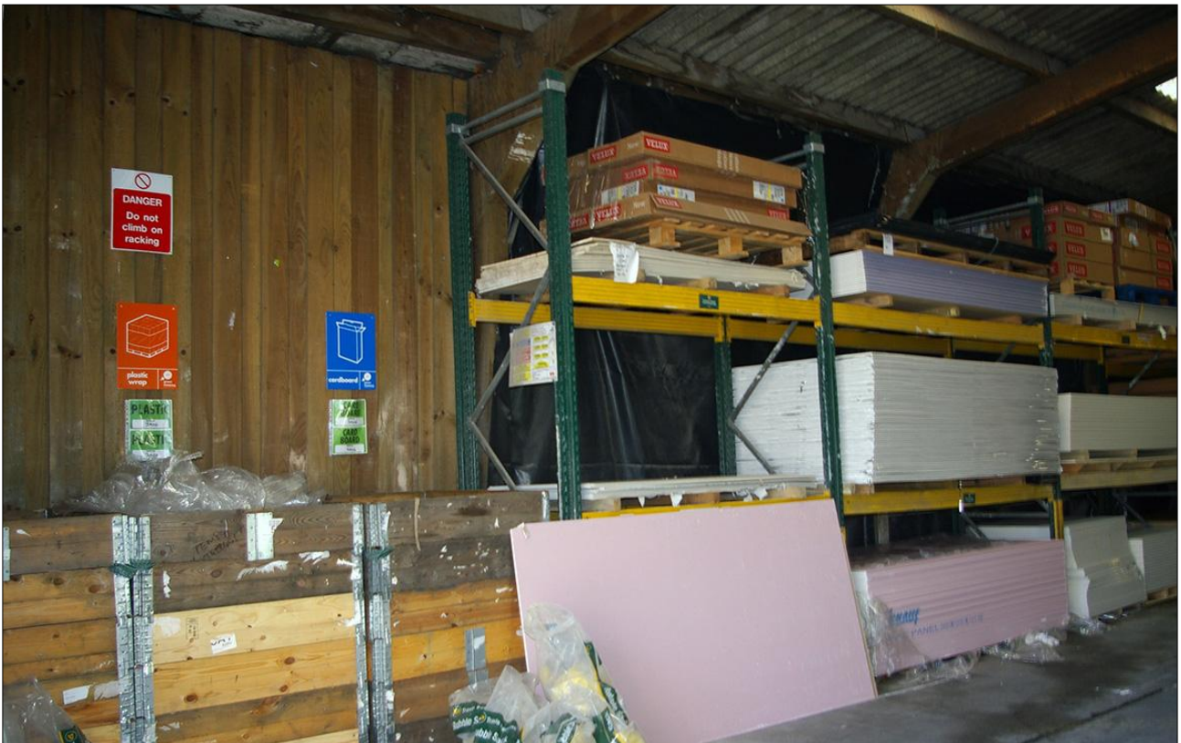
191. AS ABOVE, THE CONCEALED EAST WALL OF B3; VIEWED FROM THE SOUTH-EAST.
