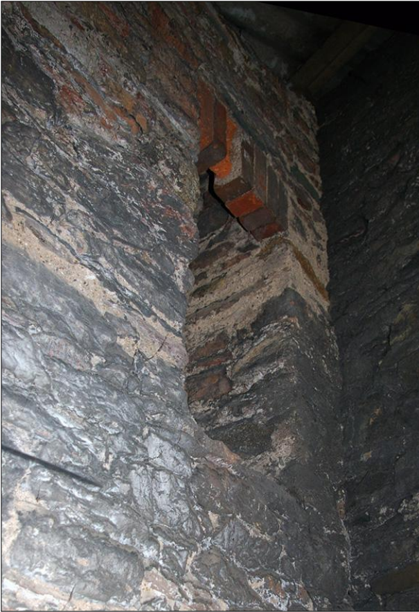
170. B3 SF INTERIOR, DETAIL OF FP4 ABOVE THE STAIRS; VIEWED FROM THE NORTH-EAST.
