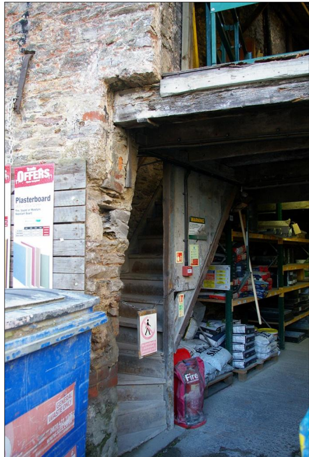
140. RIGHT: THE SOUTH ELEVATION OF B3 SHOWING THE WIDENED DOORWAY D13 WITH STAIRS (S3) BEHIND; VIEWED FROM THE SSE.
