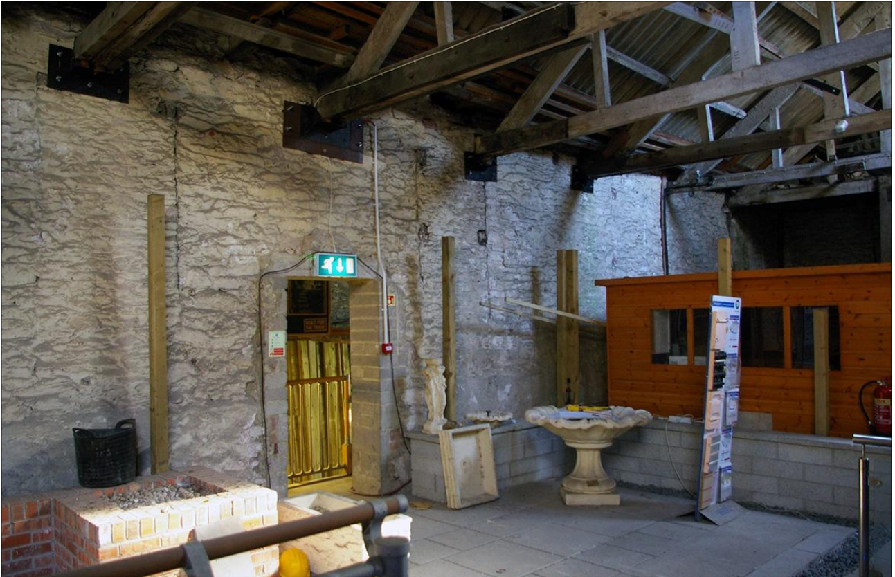
45. AS ABOVE, SHOWING THE STEEL REINFORCED TIE BEAMS ABOVE; VIEWED FROM THE NORTH-WEST.
