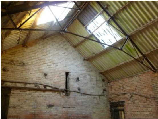
Roof in north extension, with belt slot in wall
