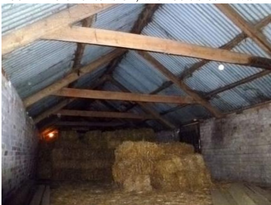
Roof structure over north shippon range
