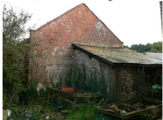
South gable of west range with lean-to shed
