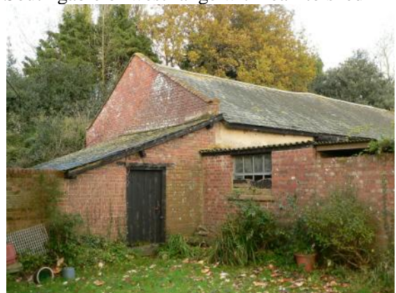
Lean-to shed at south end of west range
