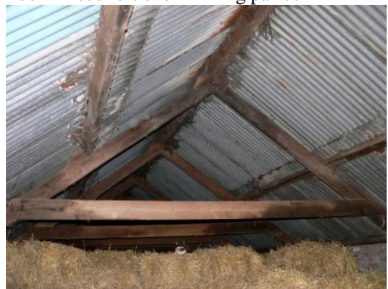
Roof structure over east shippon range
