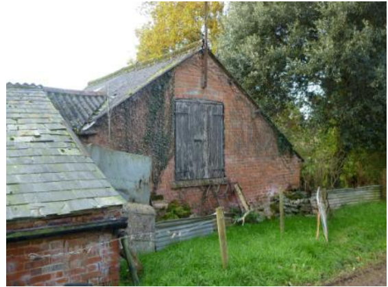
North end of west range, with loading doors
