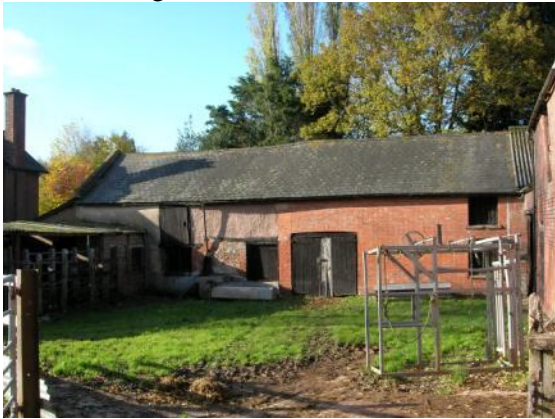
East elevation of west range
