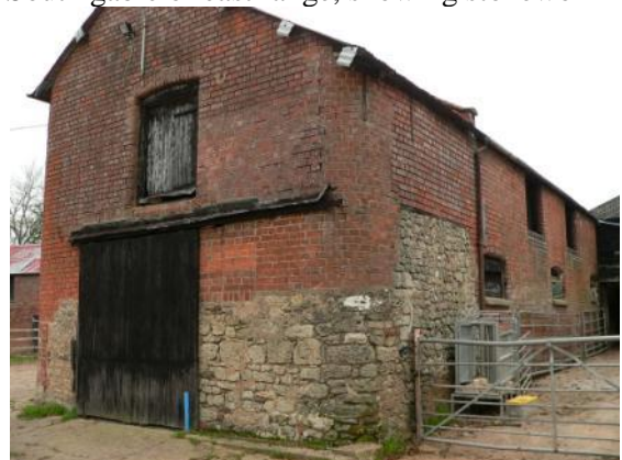
East range, south end and east side
