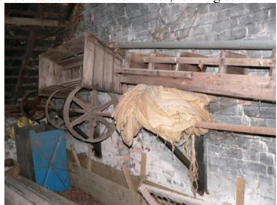
Layshaft along north wall of cider house, driven by belt from engine on floor below
