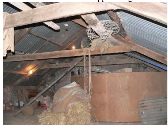
Grain silo, north end of east shippon range
