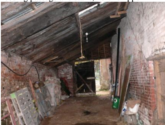
Lean-to shed, north shippon back wall to right
