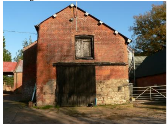
South gable of east range, showing stonework
