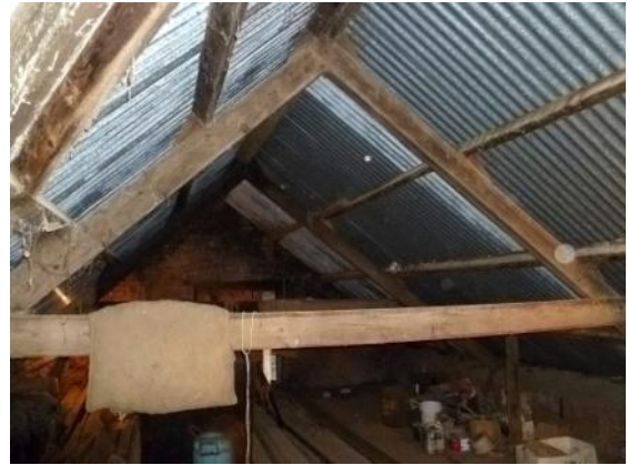
Roof in feed loft over milking parlour
