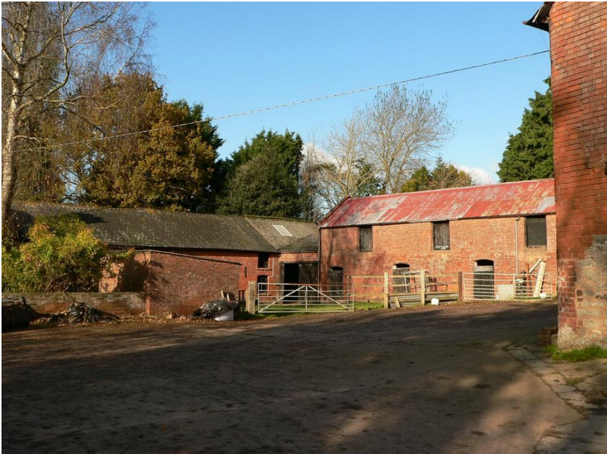
Farm buildings at Peradon, Clyst Hydon. from the south
