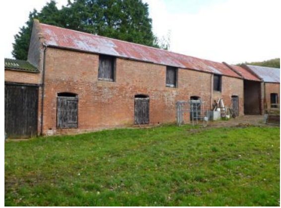
South elevation of north range
