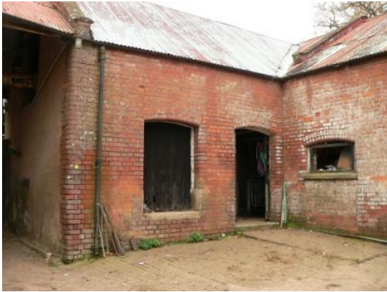
North range, dairy and milking parlour
