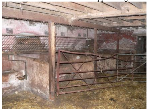
Stalls and steel supports in east shippon
