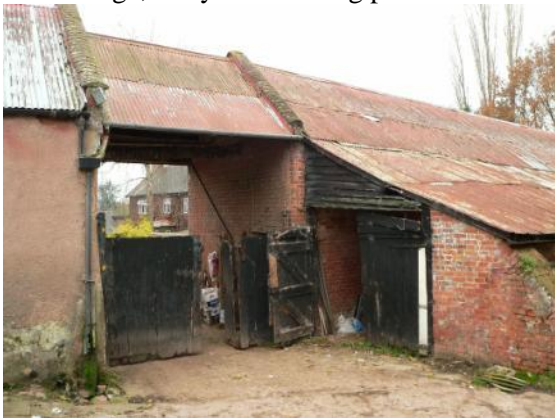
North side of passageway, north range
