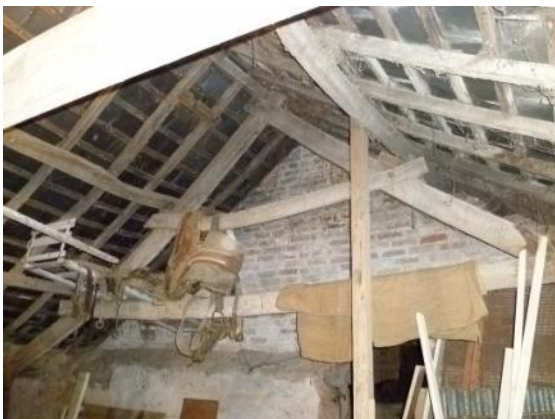
Roof truss, north end of granary, west range
