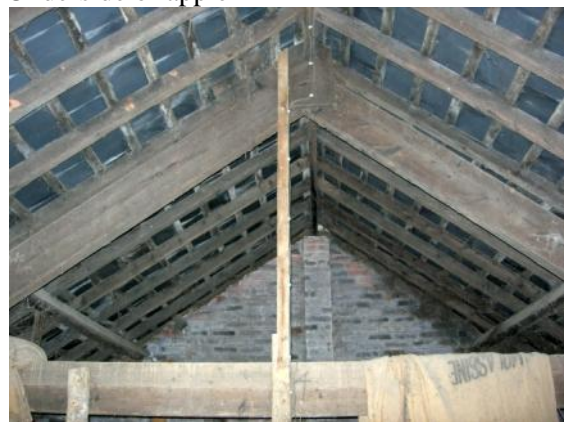
Roof structure in cider house, looking south
