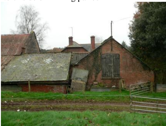
Lean-to roofed shed and north end of west range
