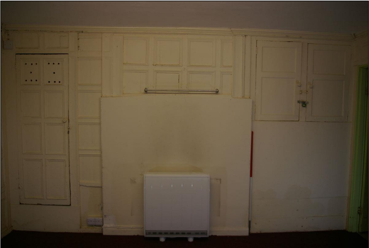
65. THE WEST WALL, WITH 1M SCALE, WITH CUPBOARD, BLOCKED FIREPLACE AND CUPBOARD TO NORTH; FROM THE EAST.
