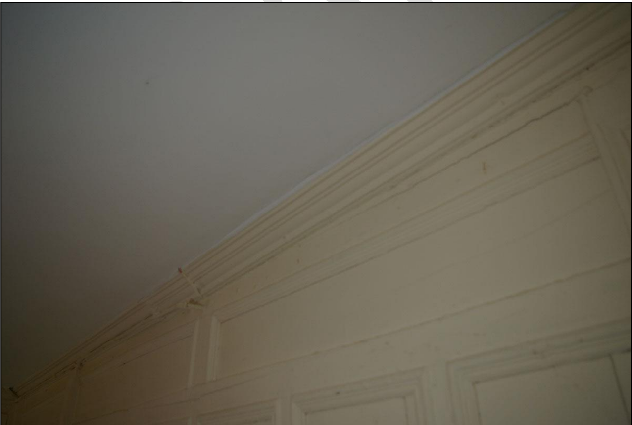
68. THE WOODEN CORNICE TO THE NORTH WALL; FROM THE EAST-SOUTH-EAST.
