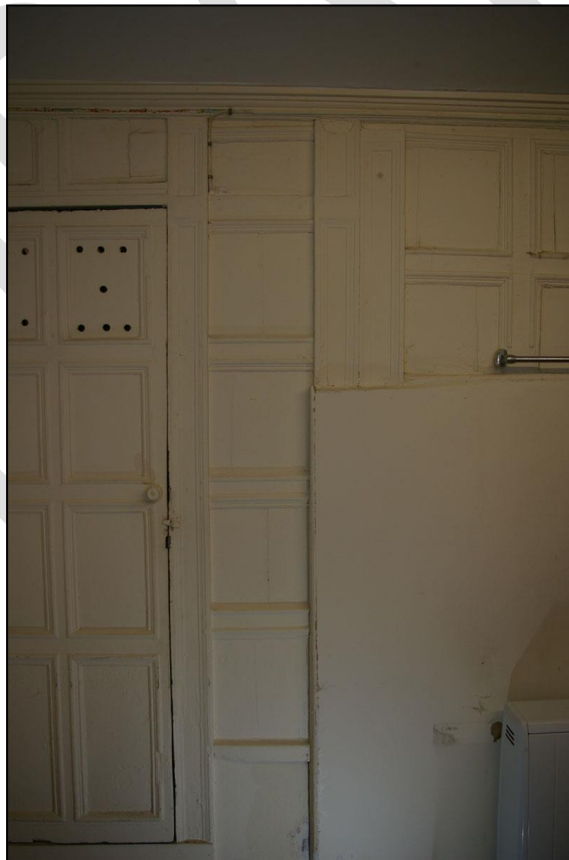
95. THE CUT AND RESET PANELLING AND PILASTERS TO THE SOUTH OF THE BLOCKED FIREPLACE; FROM THE EAST.
