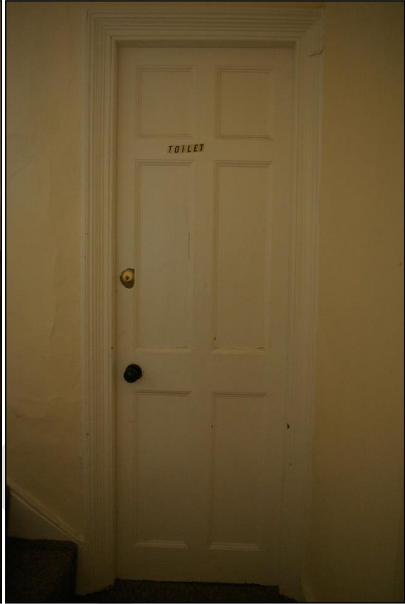
27. LEFT: THE THIRD FLIGHT OF STAIRS, SHOWING THE MOULDED HANDRAIL AND TURNED BALUSTERS; FROM THE SOUTH-WEST. 28. RIGHT: R11 AND THE DOOR TO THE LONG-DROP TOILET WHICH PROJECTS OFF THE BACK OF THE BUILDING. THE DOOR IS A SIX PANEL WITH DEEPLY REEDED FRAME; FROM THE SOUTH.
