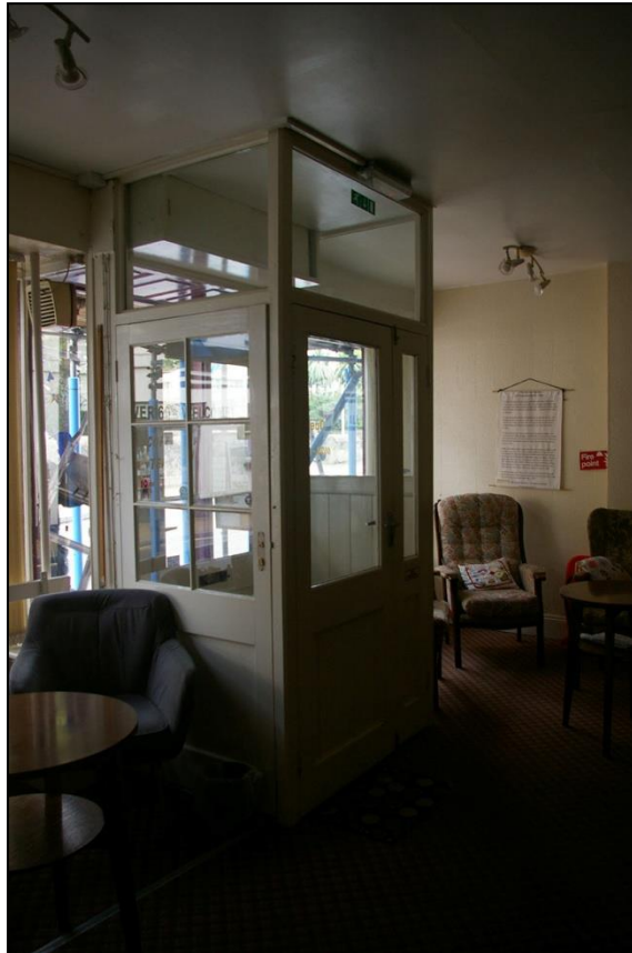
17. THE MODERN PLATE GLASS FACIA OF R2, WITH A RECYCLED COMBINATION OF DOORS AND FRAMEWORK FORMING A SMALL LOBBY; FROM THE EAST-NORTH-EAST.
