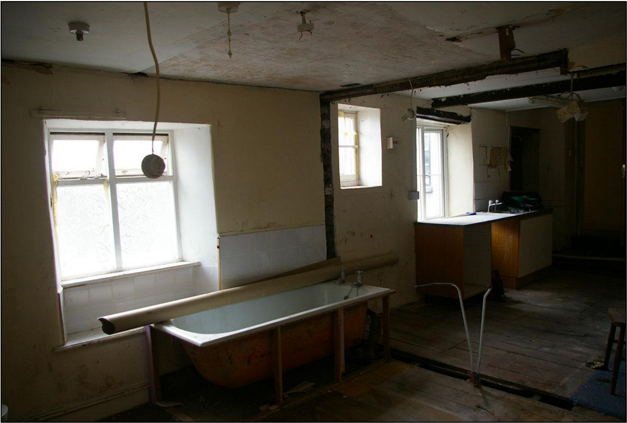
51. LONG VIEW DOWN THE EAST WALL OF ROOM 20; FROM THE NORTH-WEST.
