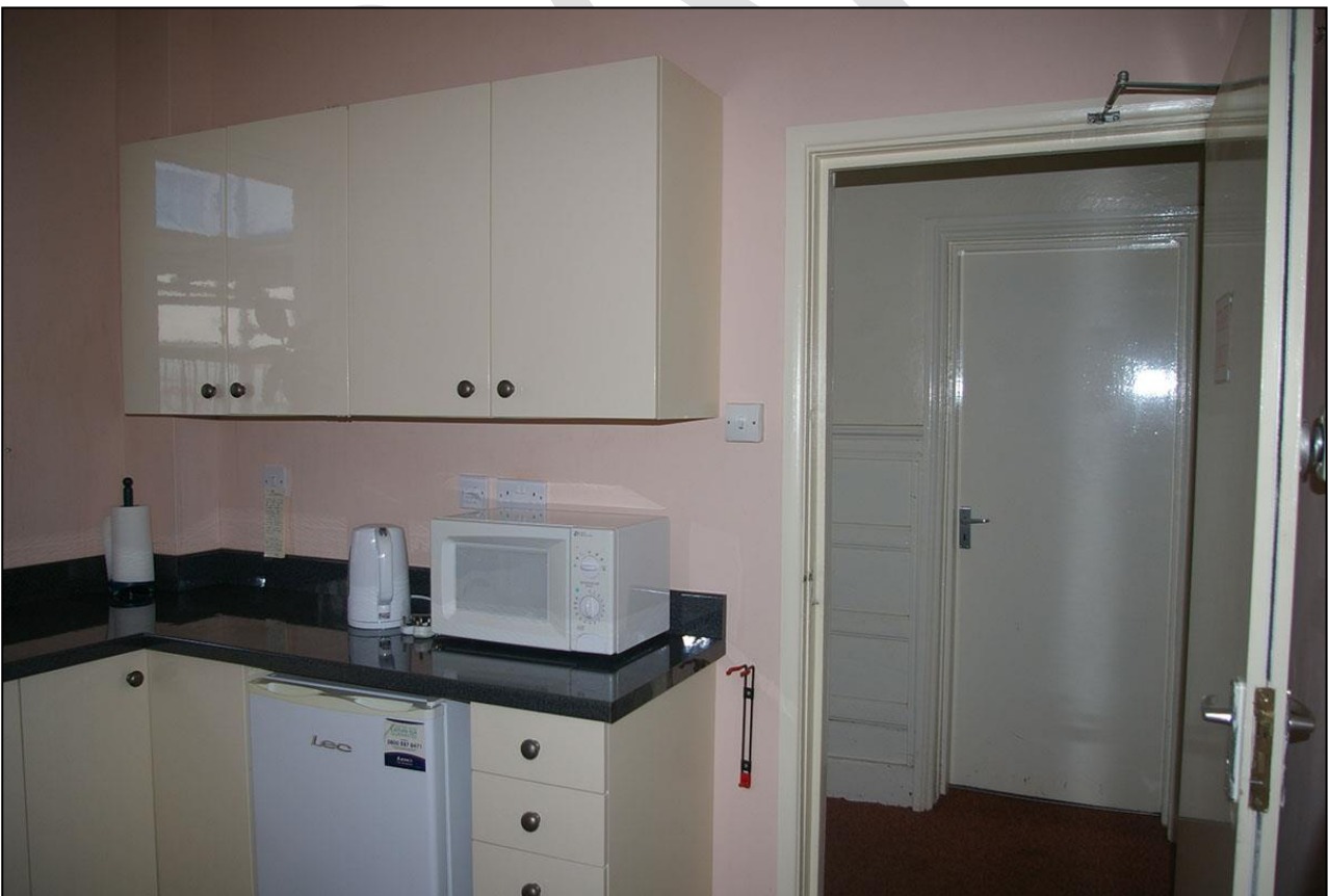
16. VIEW FROM THE OFFICE OUT OF THE DOOR TO THE MODERN DOOR OPPOSITE, LEADING TO R2; FROM THE EAST, NORTH-EAST.
