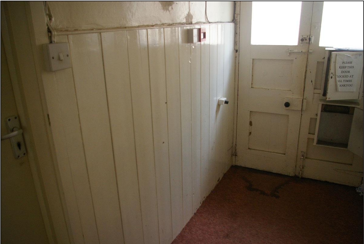
11. THE PLAIN BEADED PLANK PANELLING, 1803, TO THE EAST OF THE CORRIDOR; FROM THE NORTH-WEST. 12.
