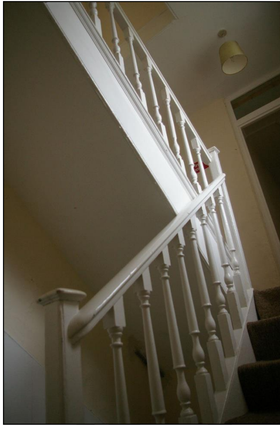
22. THE MOULDED HANDRAIL ATTACHED TO THE NEWEL POST, THE BANISTERS AND DETAILED VIEW OF THE TURNED BALUSTERS; FROM THE EAST-NORTH-EAST.
