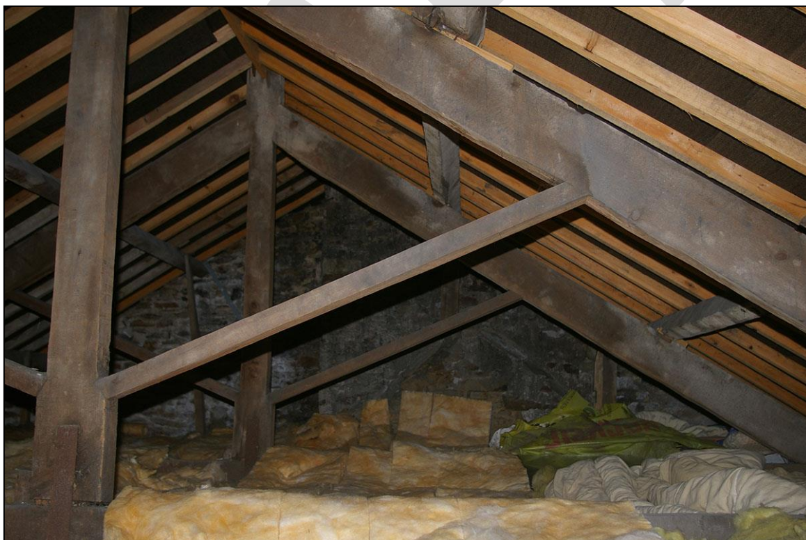
FIGURE 5: VIEW TO THE WEST PARTY WALL OF THE BUILDING, AND 19 TH CENTURY KING POST TRUSSES OF BUILDING 1; FROM THE EAST.
