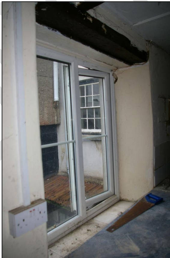
54. W17, SHOWING MODERN DOUBLE GLAZING IN DEEP OPENING, WITH WINDOW SEAT BELOW AND CHUNKY TIMBER LINTEL; FROM THE NORTH-WEST
