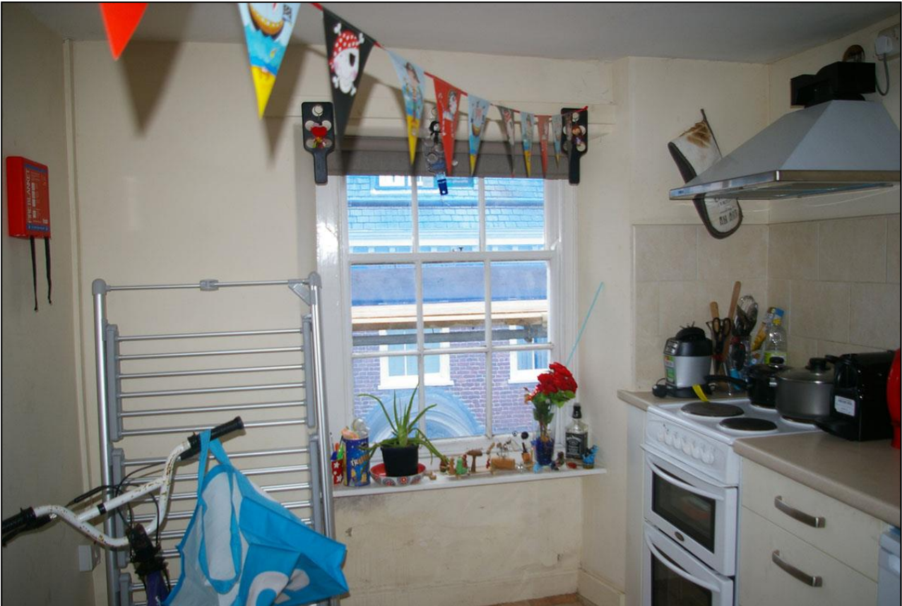
33. THE LATER HORNED SASH WINDOW WHICH LIGHTS THE KITCHEN, R14. ALSO SHOWING AN AWKWARD STEP IN THE WALL, THICKER TO THE WEST AND MAY SUGGEST INFILL BETWEEN BUILDINGS, FURTHER PHASING; FROM THE NORTH.
