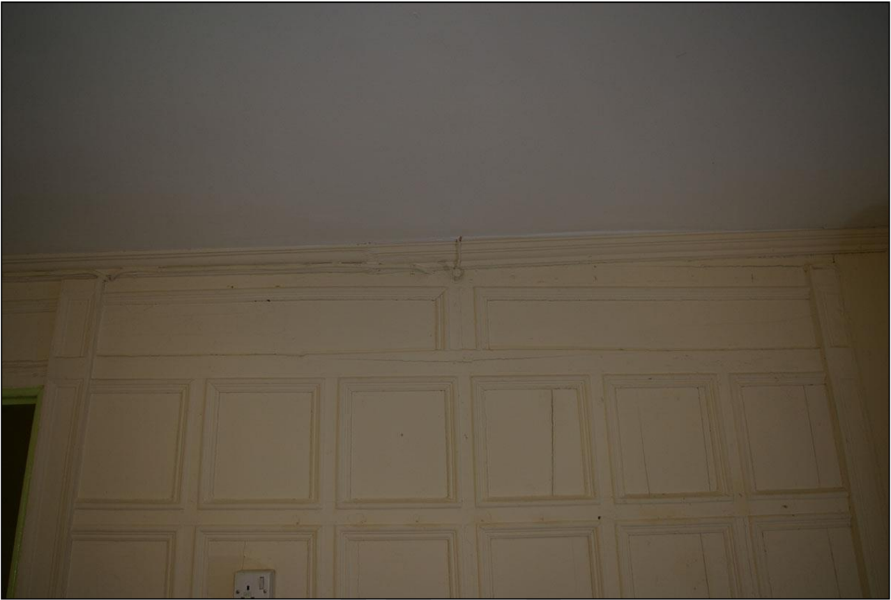
69. THE TYPE 8 TOP PANELS ON THE NORTH WALL; FROM THE SOUTH.
