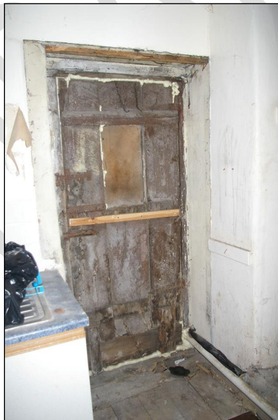
50. GOOD LATER 18 TH OR EARLY 19 TH CENTURY DOOR, D30, NAILED SHUT IN BOARDED OVER OPENING IN THE EAST WALL OF ROOM 20; FROM THE WEST-NORTH-WEST (WITH FLASH).
