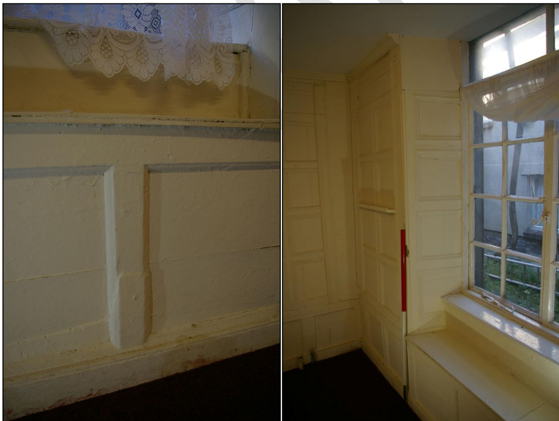
78. LEFT: THE CHUNKY BEAD MOULDING UNDER THE WINDOW SEAT, ON THE EAST WALL; FROM THE NORTH-WEST.
