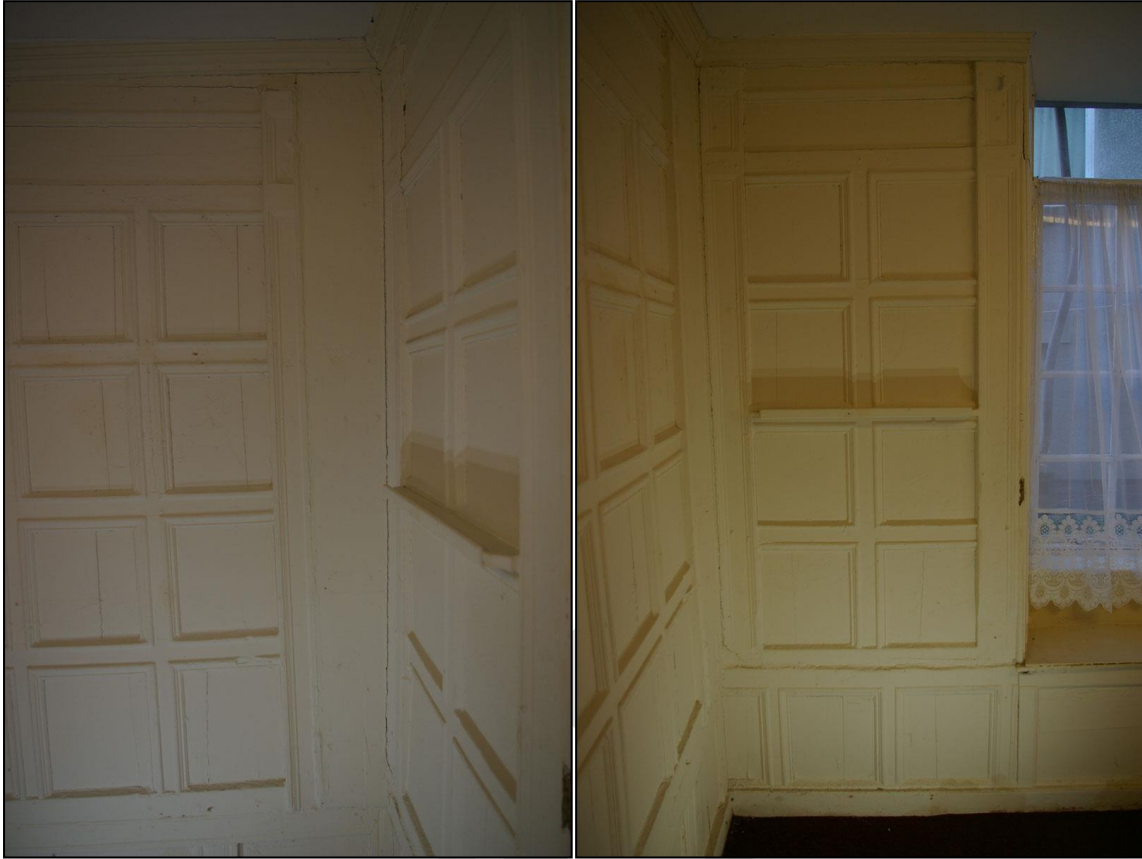
74. LEFT: THE END PILASTER OF THE NORTH WALL TO THE EAST, TYPE 5, WITH PLAIN PLANKS IN THE CORNERS; FROM THE SOUTH.
