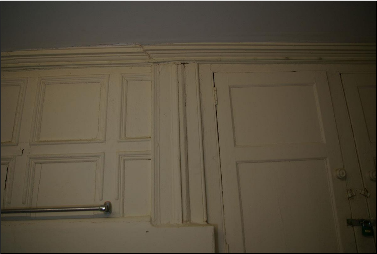
98. THE CUT AND RESET PILASTERS BETWEEN THE PANELLING AND CUPBOARD TO THE NORTH OF THE FIREPLACE; FROM THE EAST.
