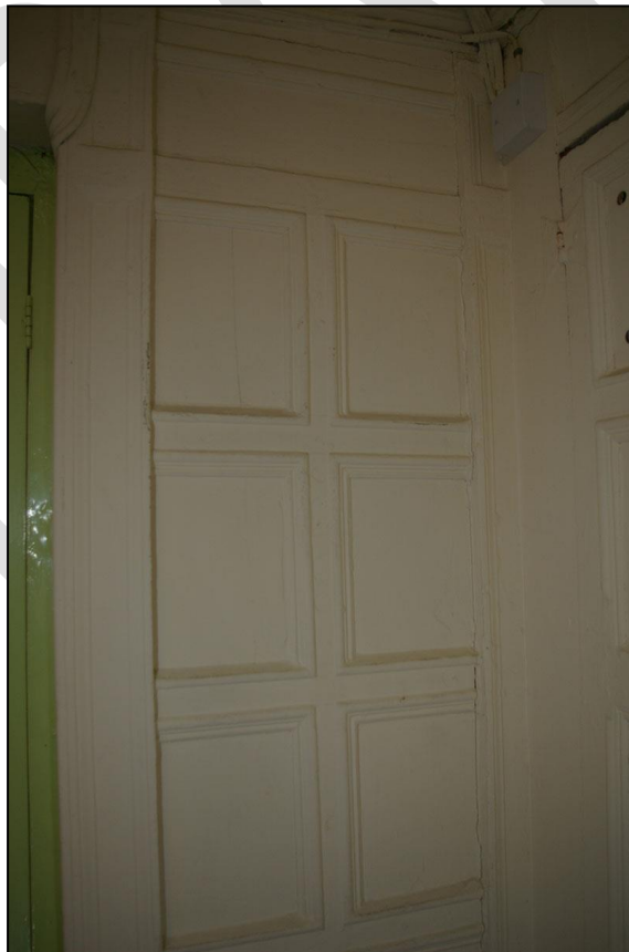
90. THE SOUTH-WEST CORNER, WITH PILASTERS AND TYPE 3 PANELLING; FROM THE NORTH-EAST
