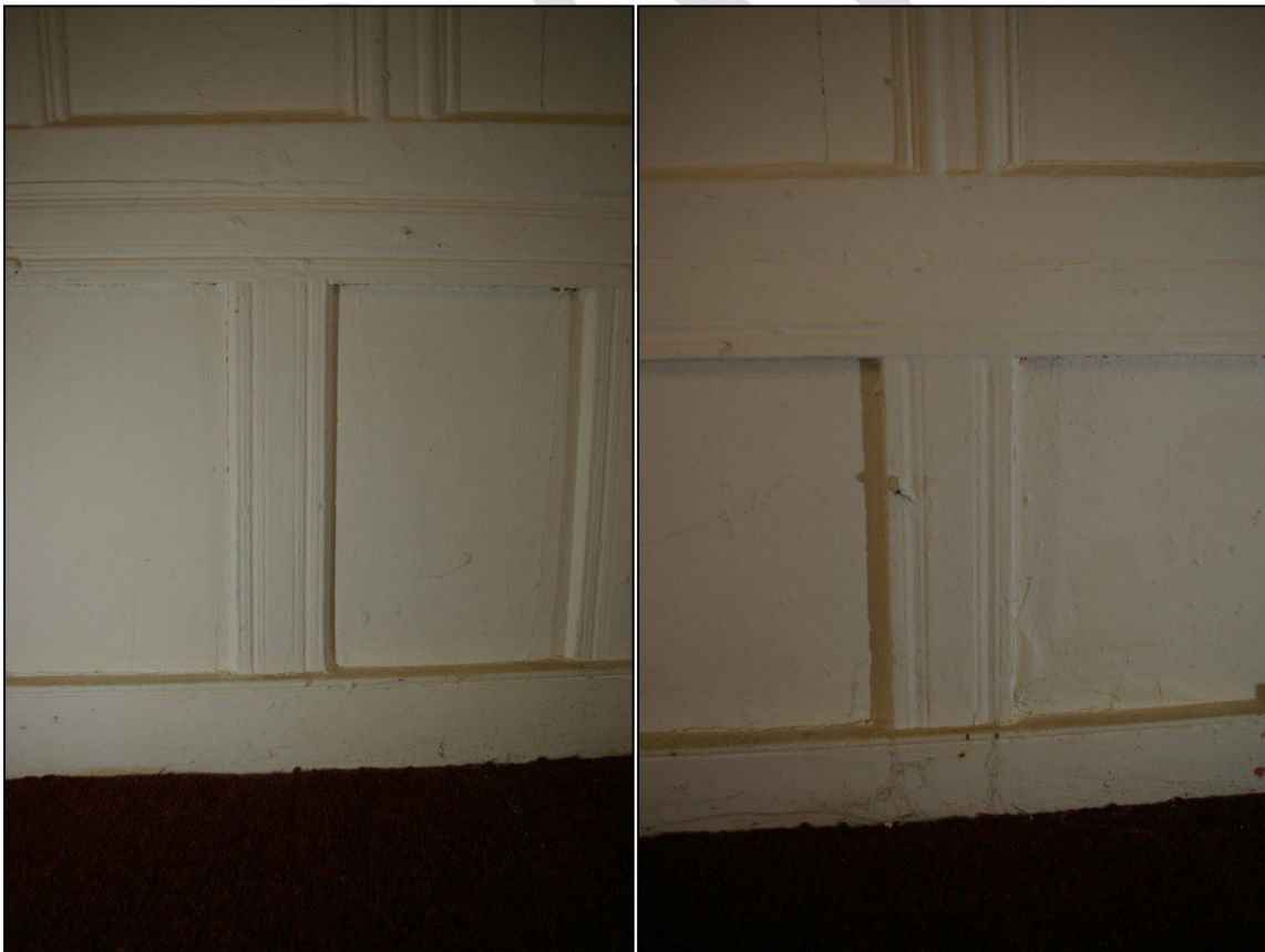
72. LEFT: THE SCRATCH MOULDED PANELS; FROM THE SOUTH.
