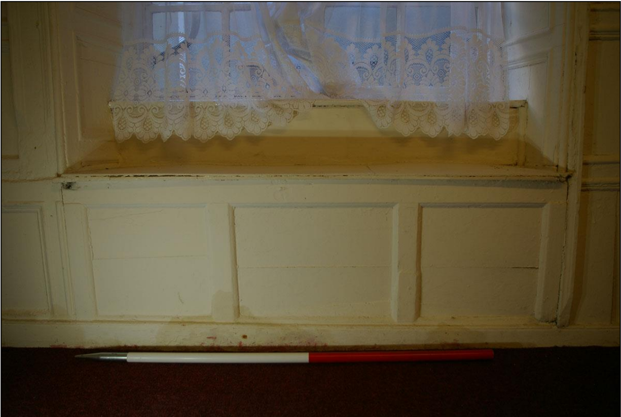
77. THE PANEL UNDER THE WINDOW SEAT AND W13, WITH 1M SCALE, THIS TYPE 9 PANEL IS LIKELY 19 TH CENTURY; FROM THE WEST.
