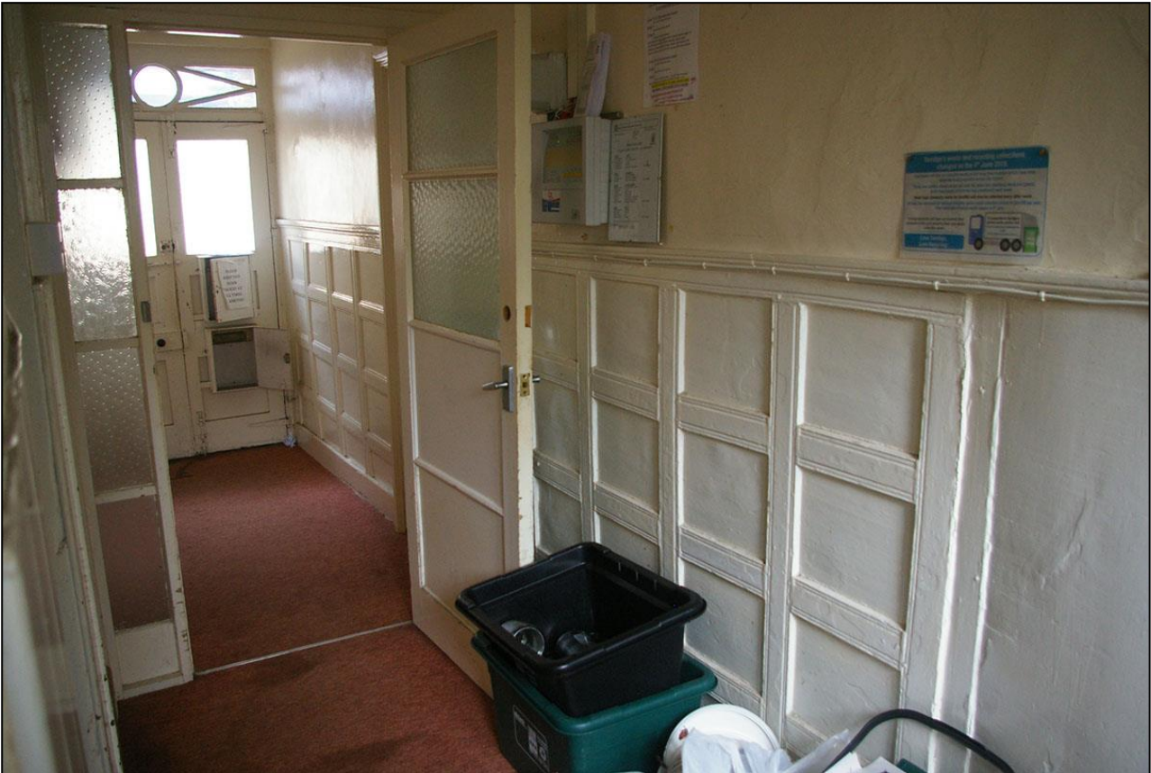
9. VIEW ALONG THE WEST WALL OF R1 AND R1A, SHOWING TWO PHASES OF PANELLING; FROM THE NORTH-EAST.
