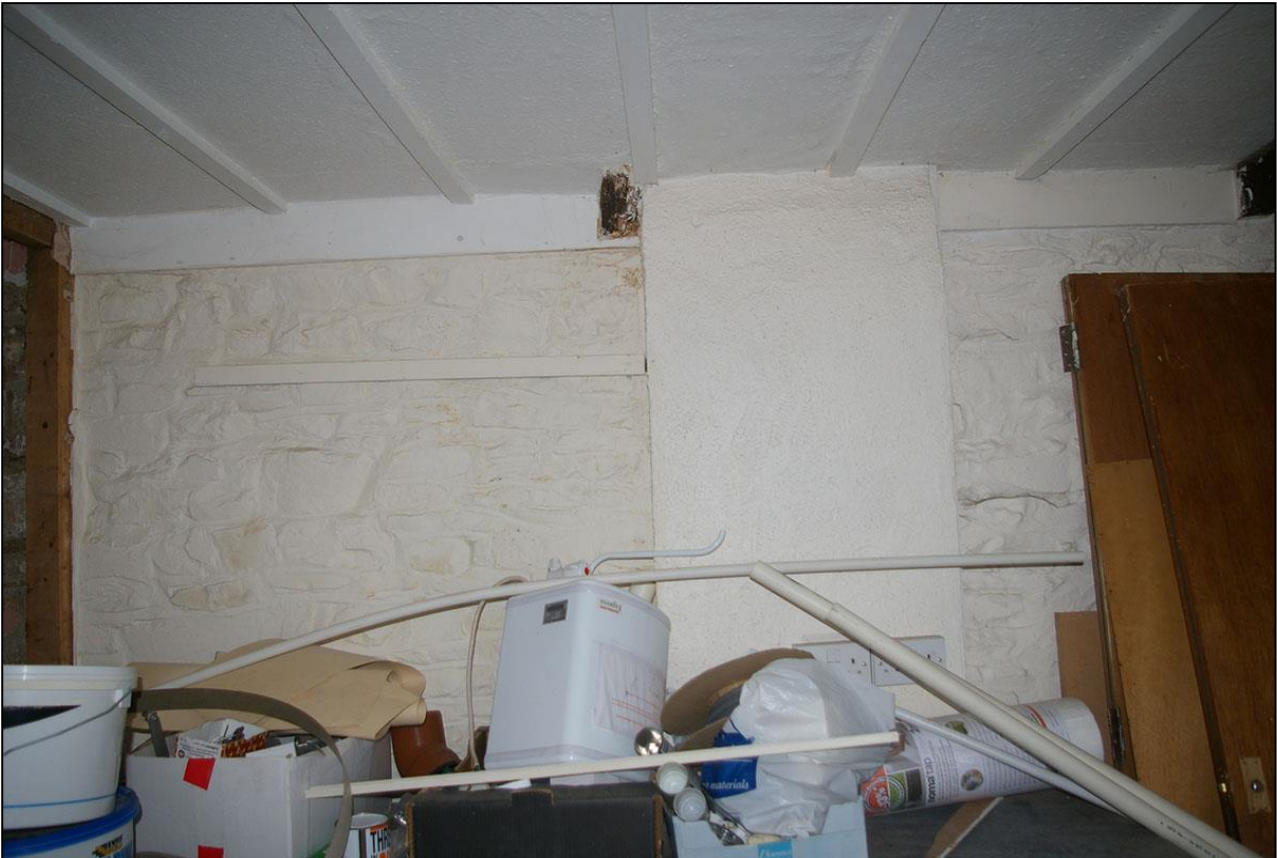
55. THE NARROW BRICK RENDERED STACK BUILT ONTO THE EARLIER HEAVY STONE RUBBLE WEST WALL OF ROOM 20; FROM THE EAST.
