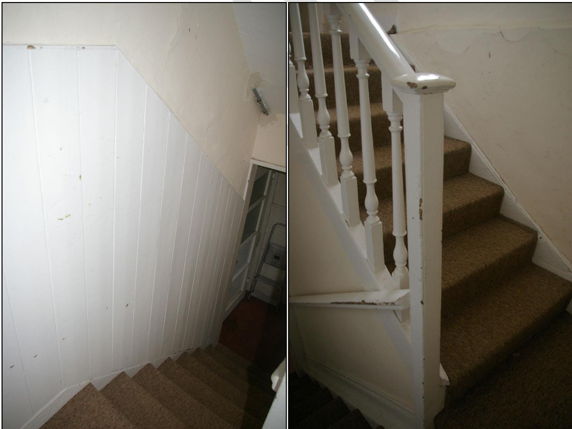
20. LEFT: THE BEADED PLANK PANELLING ON THE PARTITION WALL BETWEEN R5 AND R3; FROM THE NORTH-EAST.
