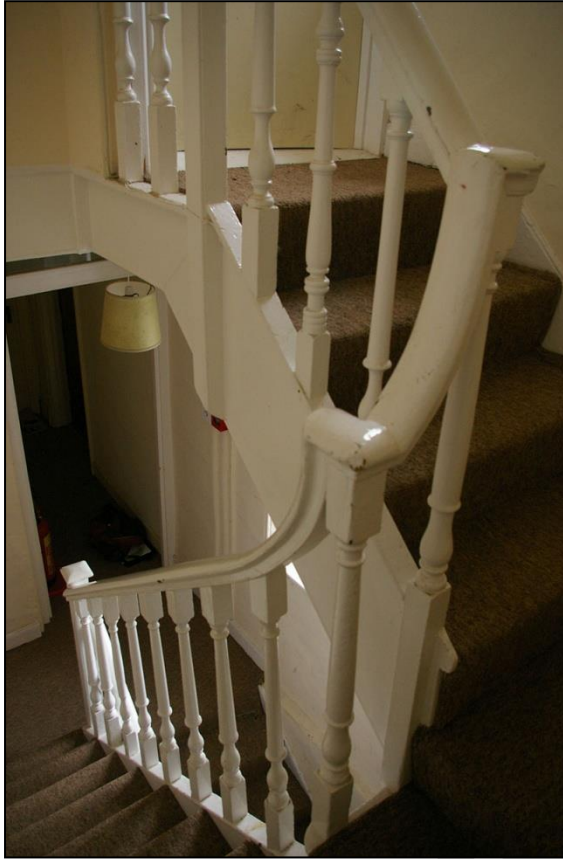
27. LEFT: THE THIRD FLIGHT OF STAIRS, SHOWING THE MOULDED HANDRAIL AND TURNED BALUSTERS; FROM THE SOUTH-WEST. 28. RIGHT: R11 AND THE DOOR TO THE LONG-DROP TOILET WHICH PROJECTS OFF THE BACK OF THE BUILDING. THE DOOR IS A SIX PANEL WITH DEEPLY REEDED FRAME; FROM THE SOUTH.
