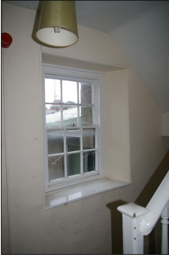
24. LEFT: THE SASH WINDOW IN R6, THE FIRST FLOOR LANDING, A HORNLESS SASH, IN A CHUNKY MOULDED SASH BOX; FROM THE SOUTH-WEST.
