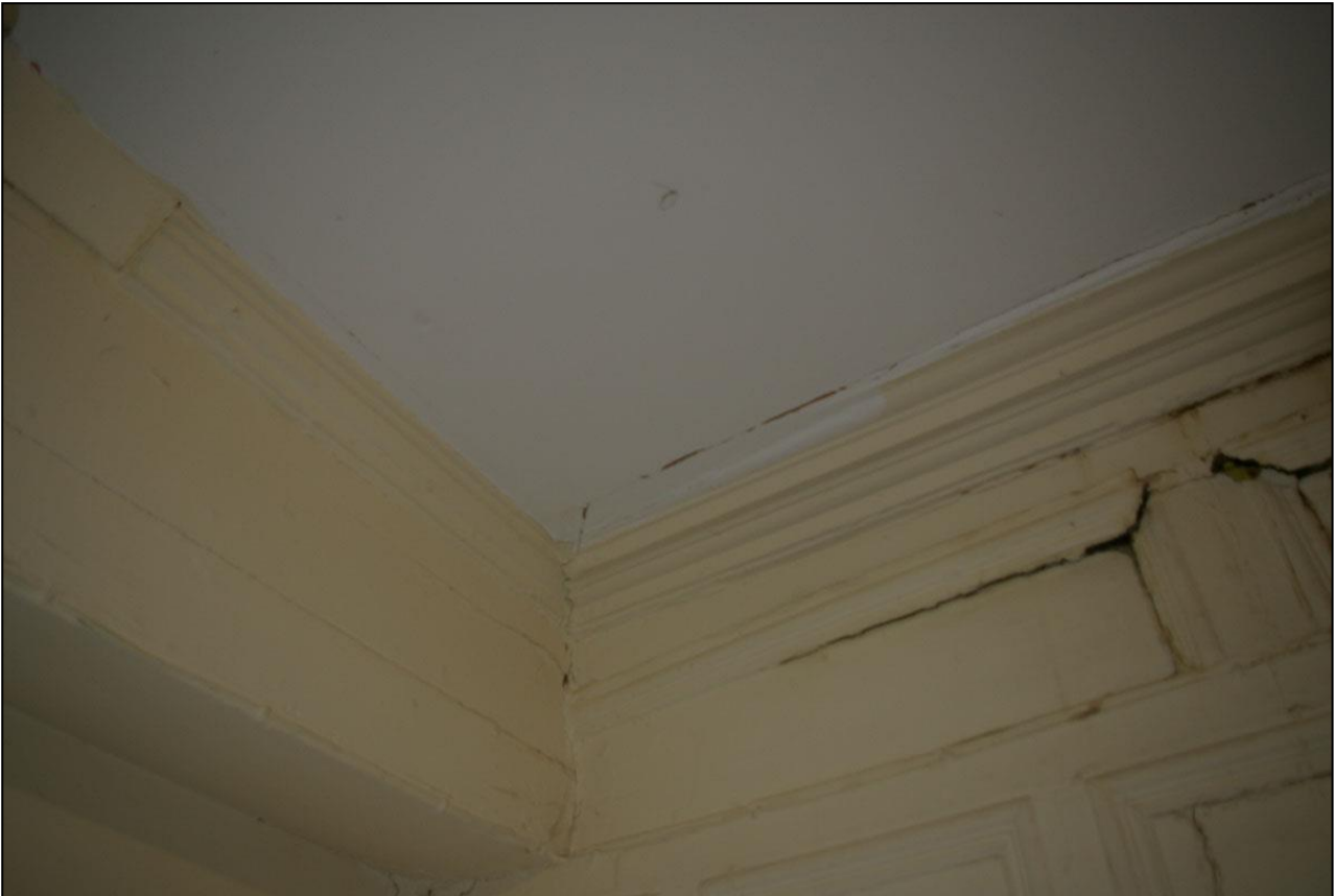
83. THE DIFFERENT WOODEN CORNICES MEETING IN THE SOUTH-EAST CORNER OF THE ROOM; FROM THE NORTH-WEST.
