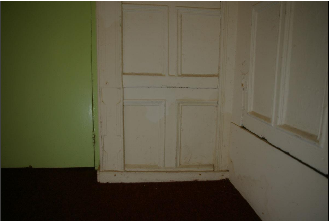
91. THE CUT AND RESET PANNELLING IN THE SOUTH-WEST CORNER; FROM THE NORTH.
