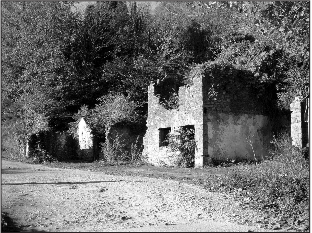
Plate 4 The stable and coach house, viewed looking north-west, November 2005.
