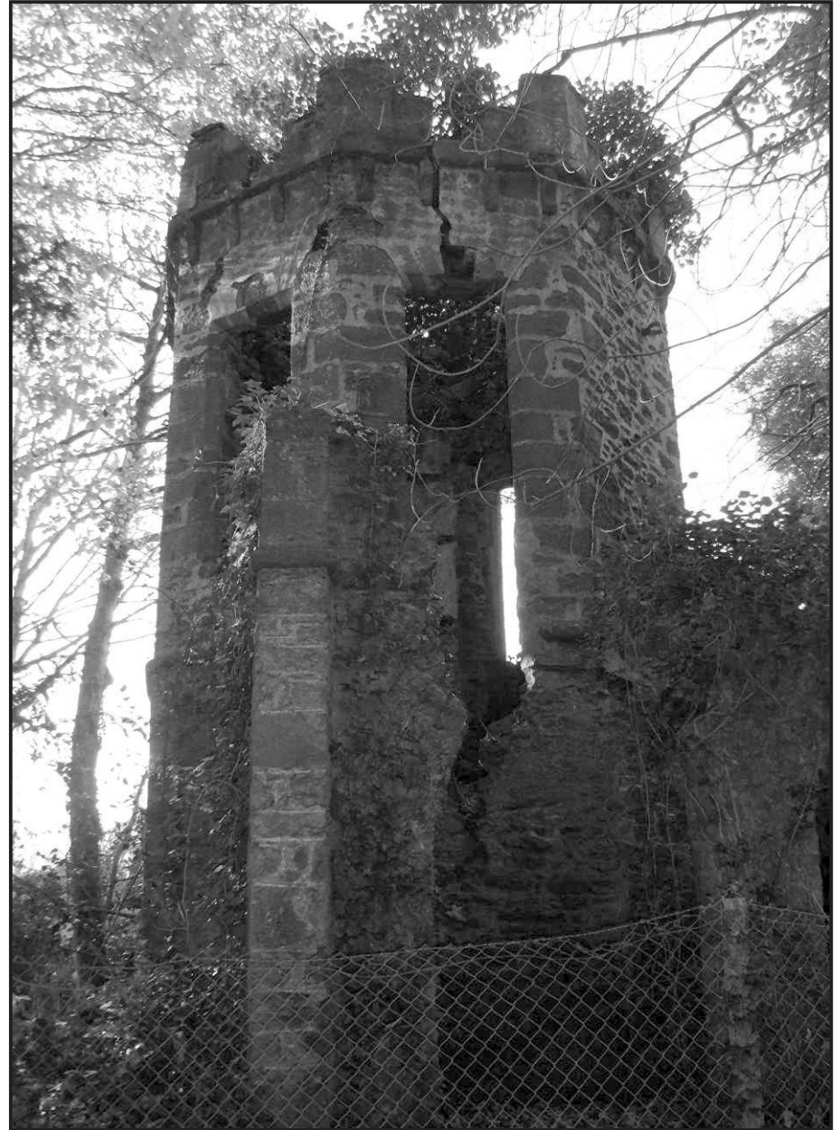
Plate 3 The gazebo or folly, looking south, also showing one of the collapsed arches of the annex, November 2005.
