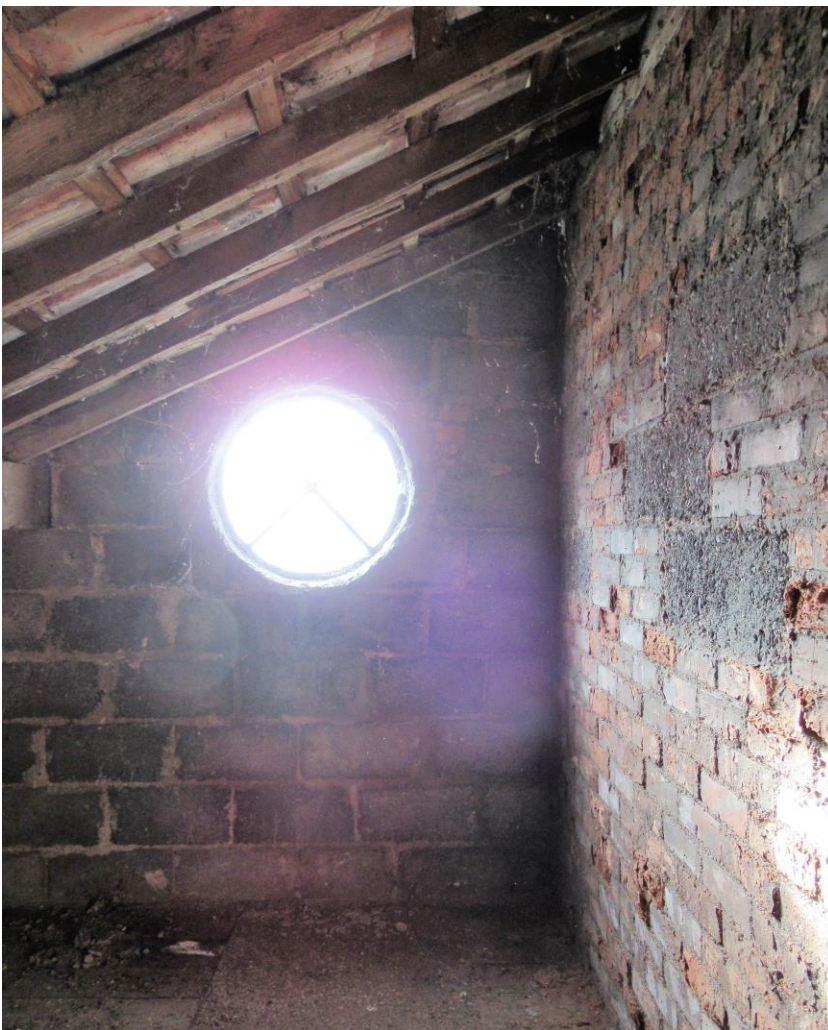
Plate 17: South wall of first floor
