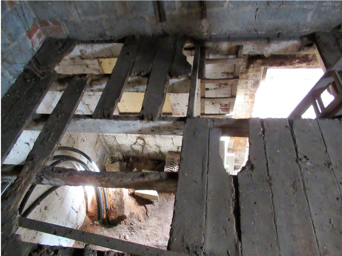
Plate 14: First floor structure from above
