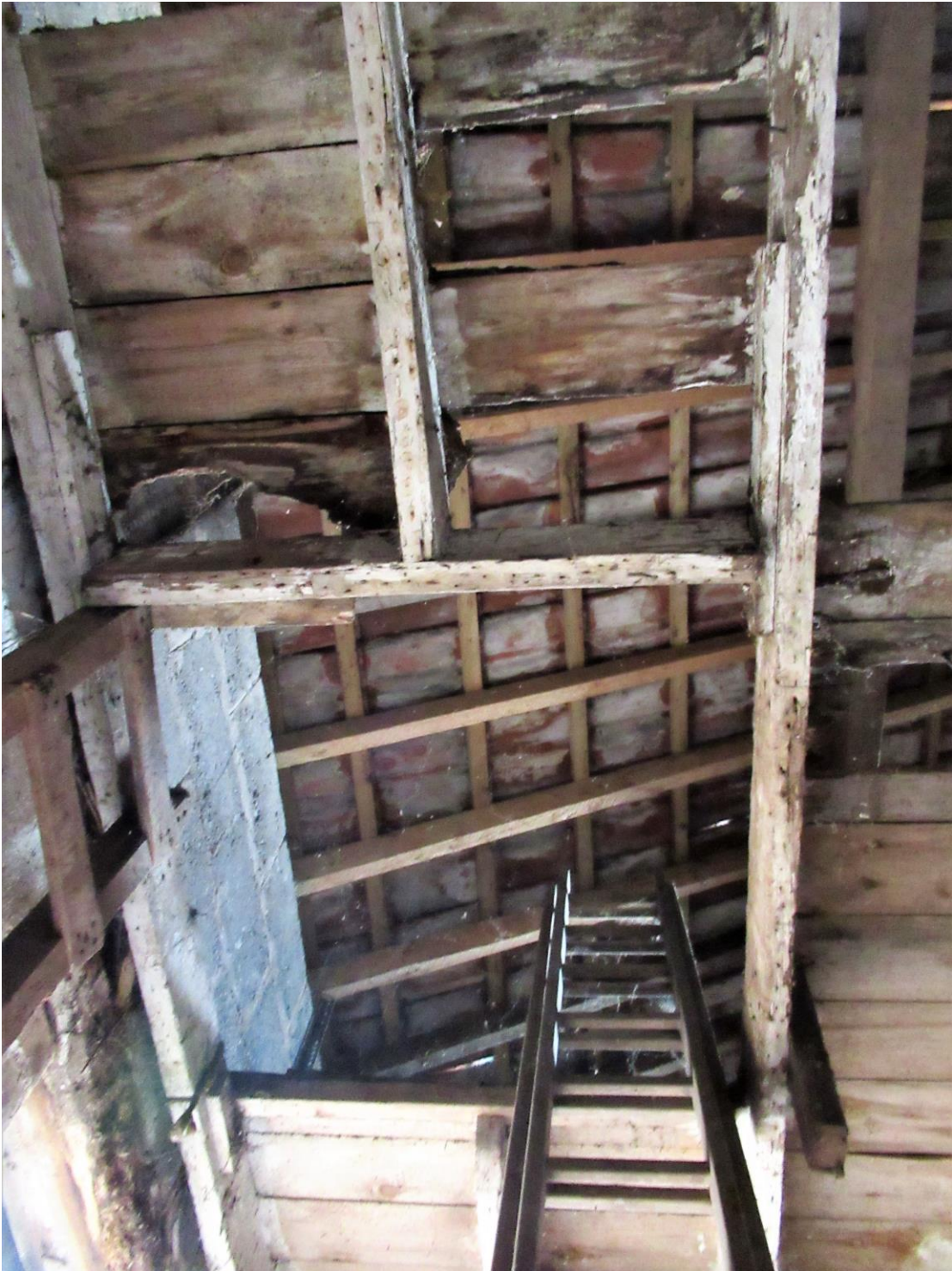
Plate 13: Underside of ceiling showing opening and underside of roof structure above
