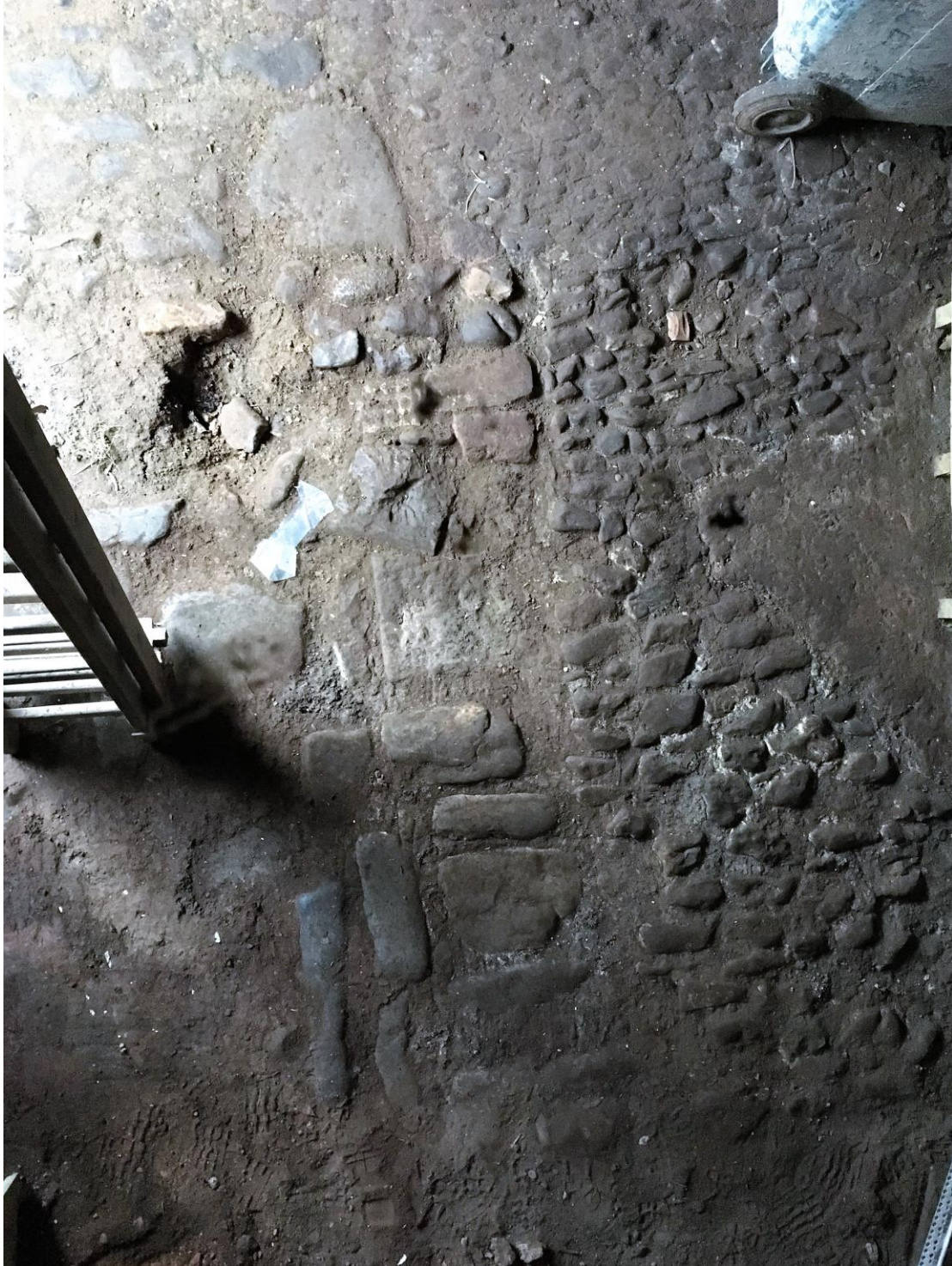
Plate 12: Cobbled floor on ground floor and larger paving stones around doorway and ladder
