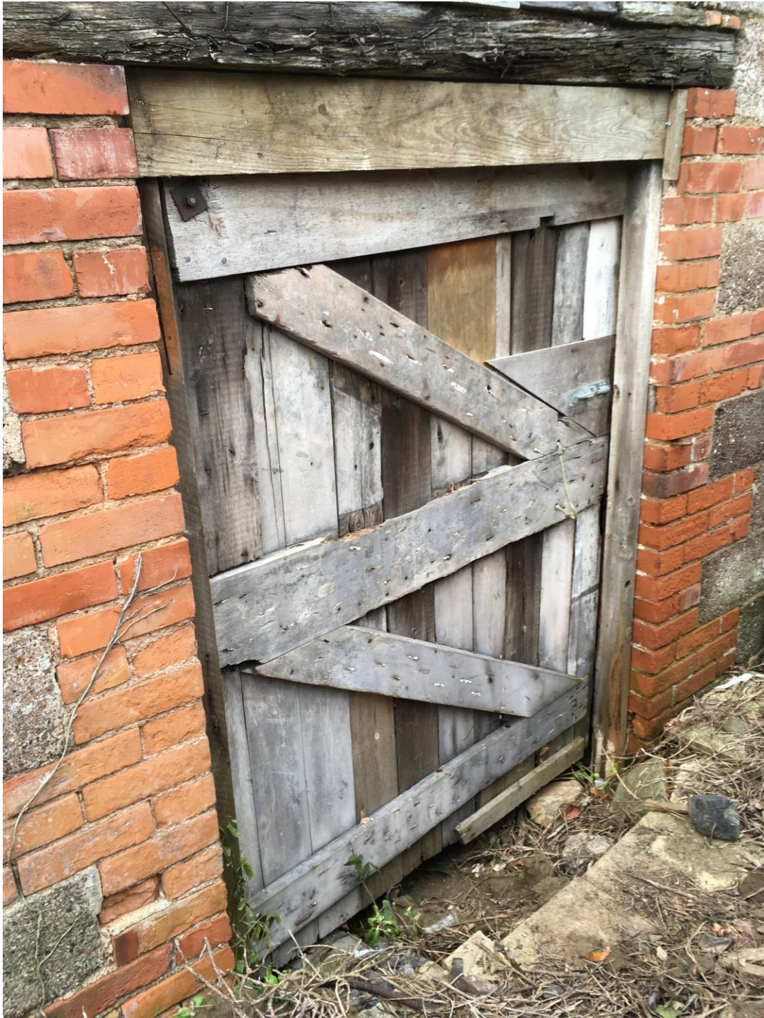
Plate 7: Ledged and braced plank door on east wall
