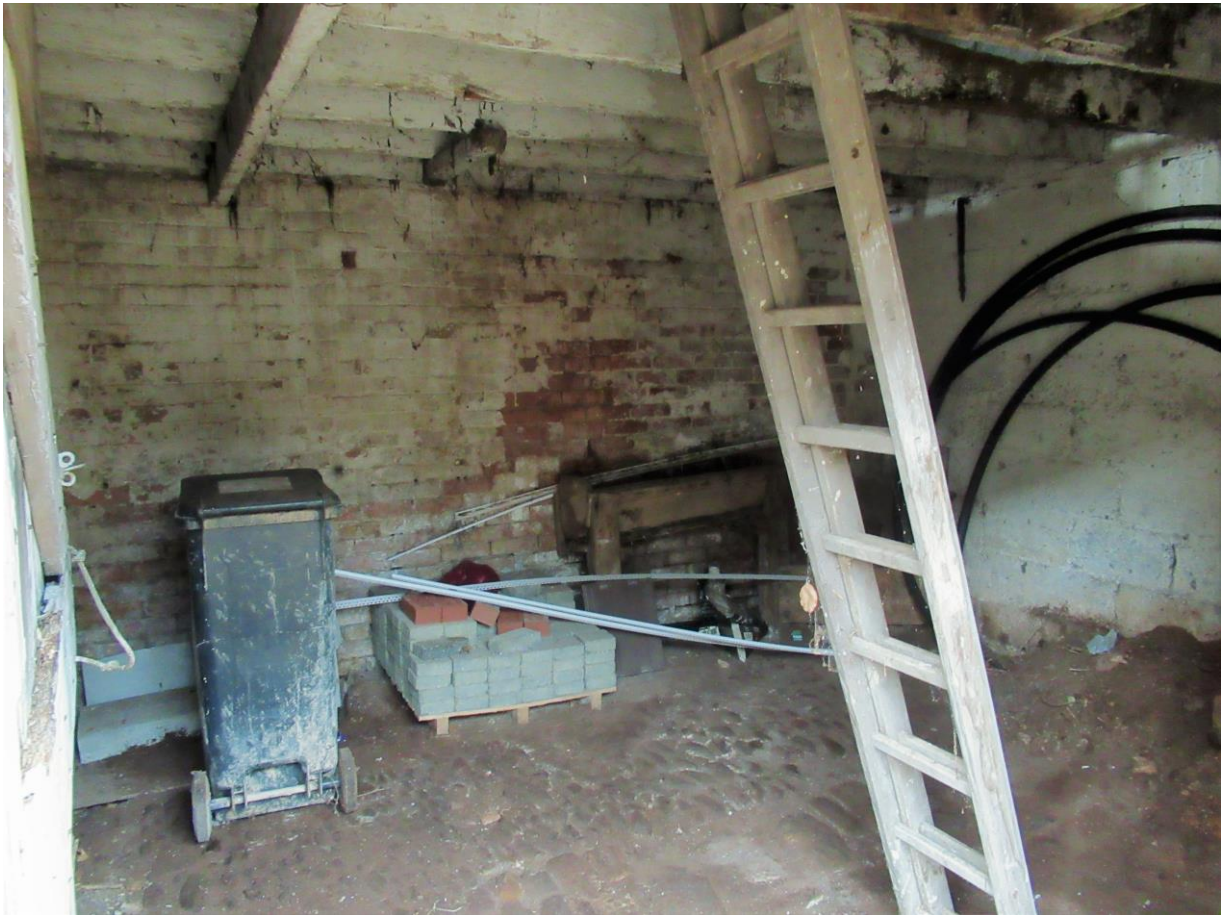
Plate 10: Interior of ground floor viewed from doorway
