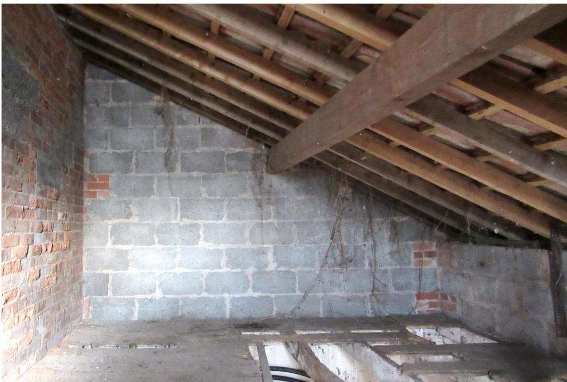
Plate 15: First floor looking north
