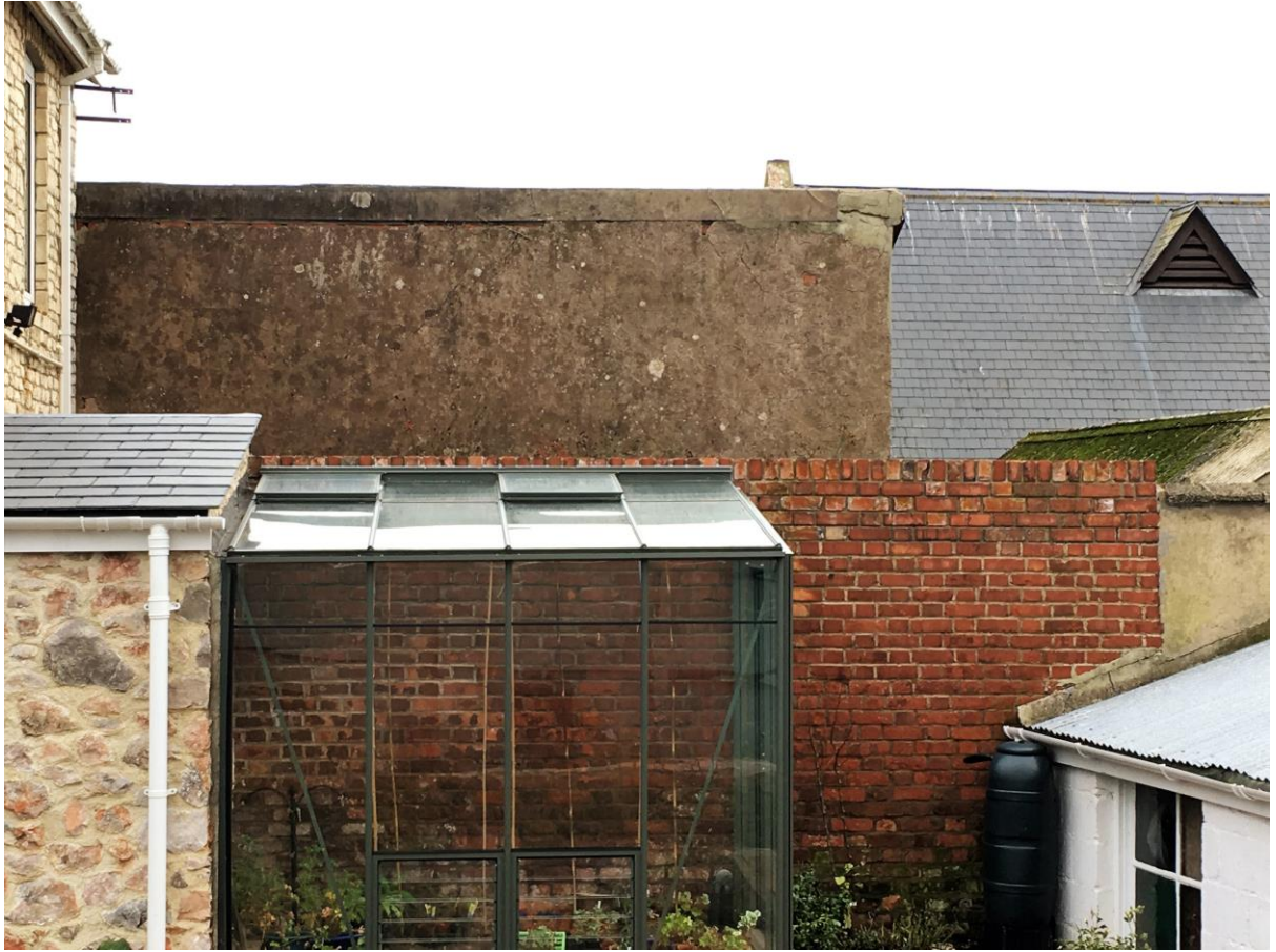
Plate 6: Rendered west elevation of stable visible above brick party wall
