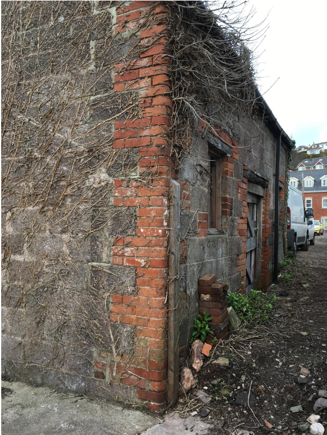
Plate 4: South-eastern corner of the stable showing bull-nosed brick quoins
