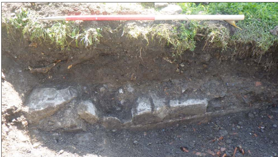
Plate 3: Trench 2, modern wall footing S203, looking south (1m scale)
