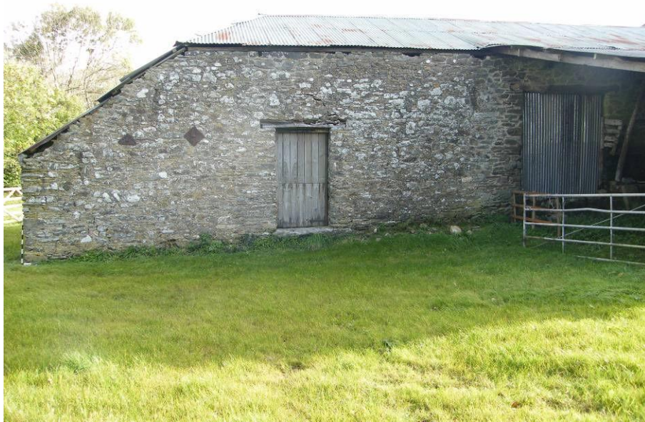
Plate 5: Southwest elevation of the threshing barn and shippon, viewed looking northeast
