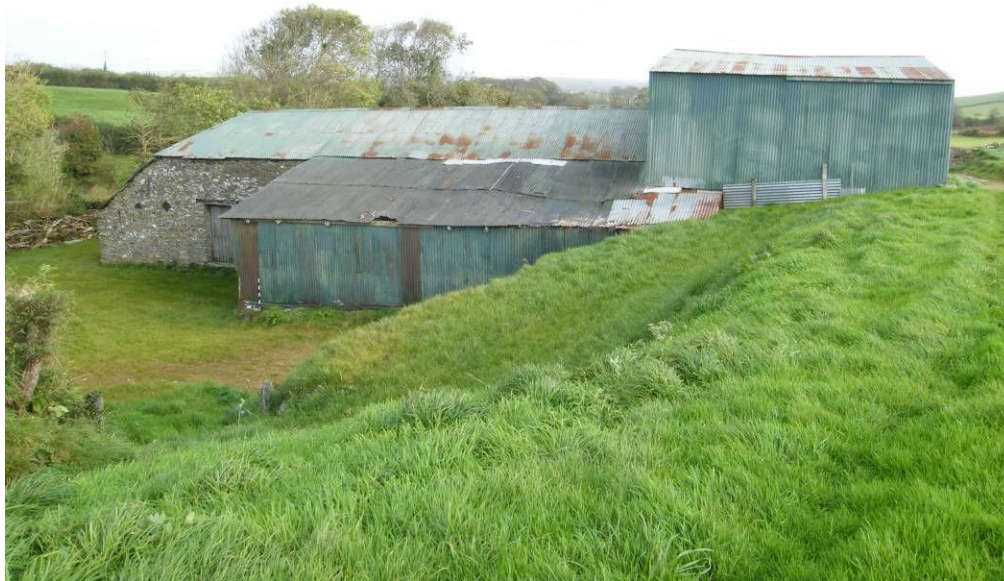
Plate 1: General view of the barn, viewed looking north northeast
