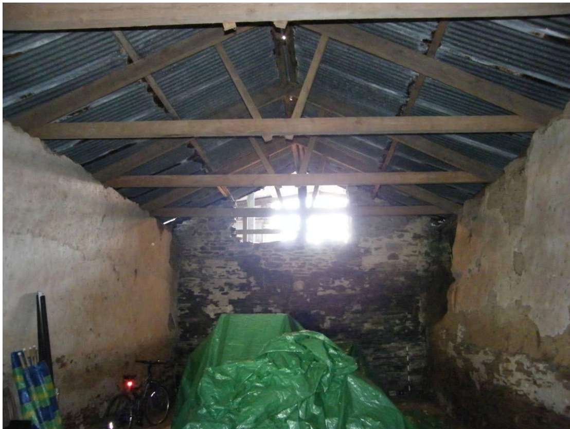
Plate 10: General view of the barns interior, viewed looking southeast
