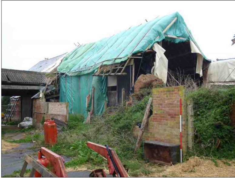
Plate 10: The threshing barn, looking northwest (2m scale)
