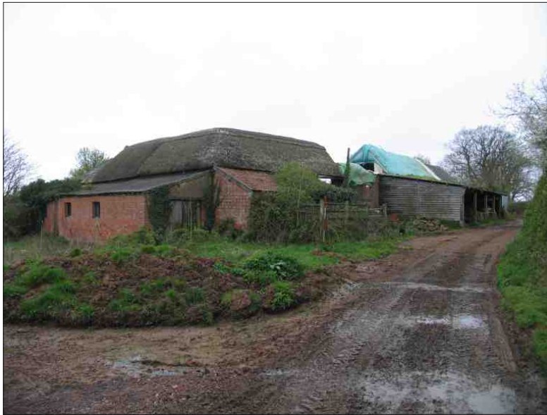
Plate 1: The dairy with attached root store (centre and left) and threshing barn with attached lean-to beyond to the right, looking southwest (2m scale)
