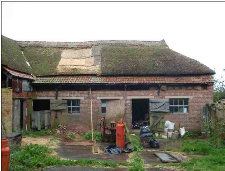
Plate 2: The dairy, looking east (2m scale)
