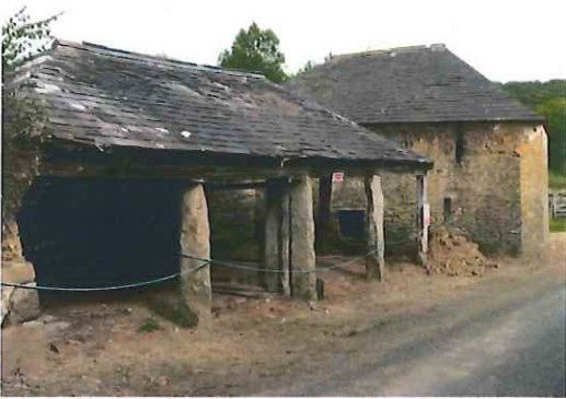
Cart shed and south-east corner of mill
