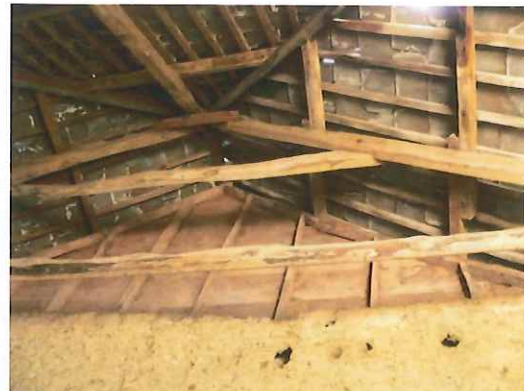
Mill roof: general construction, looking east
