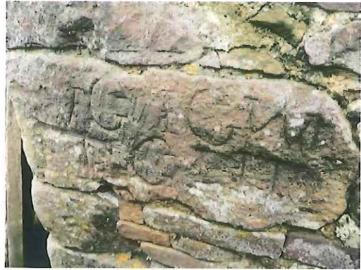
Carved stone by mill door, north elevation
