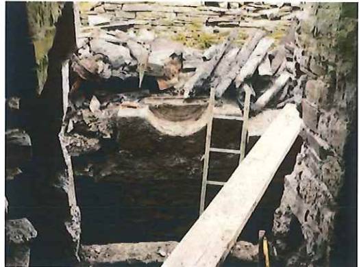
Looking west across wheelpit to bearing block
