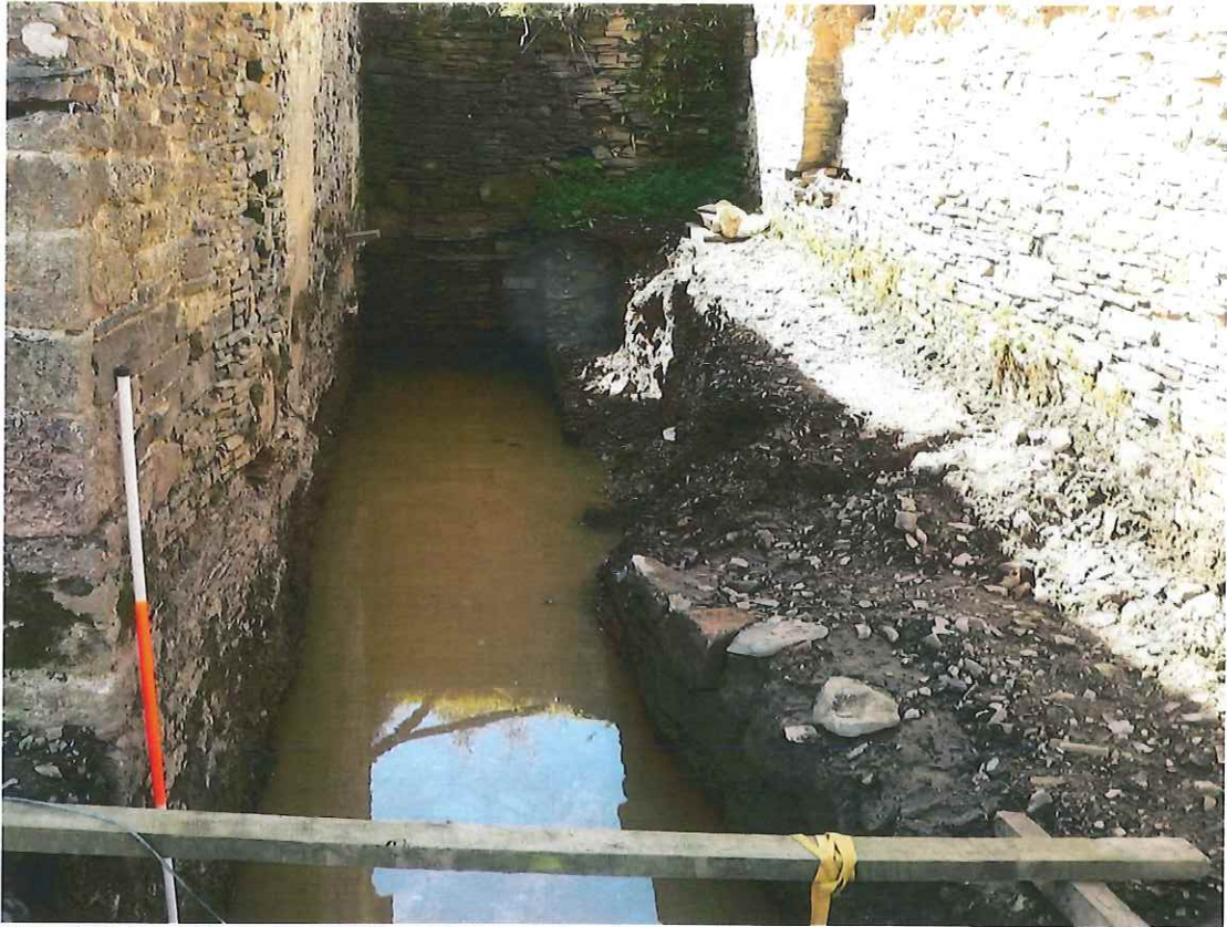
Wheelpit from downstream after clearance, showing standing ground water. August 2011
