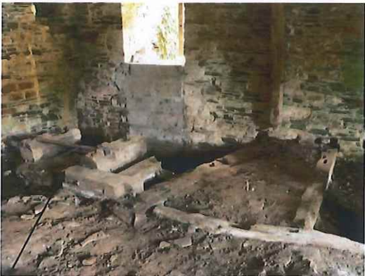
Bearing block and south cog pit
