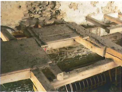
1st floor, remains of sack traps
