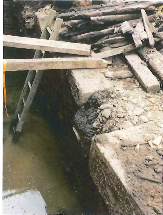
Granite blocks on west side of wheelpit
