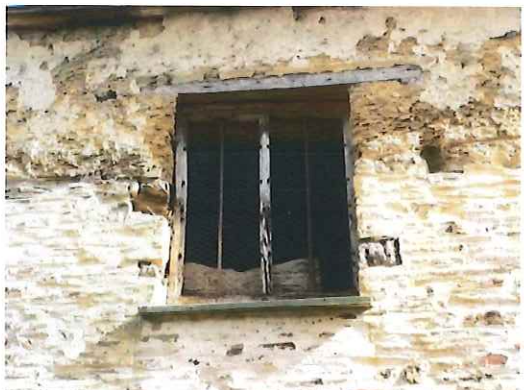
1st floor window, west elevation (south)
