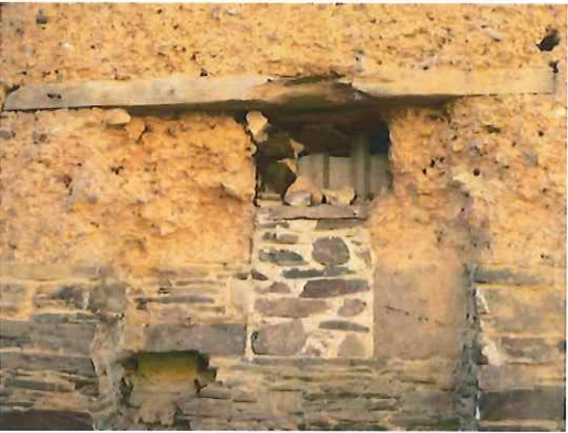
Position of mechanical drive into cider barn
