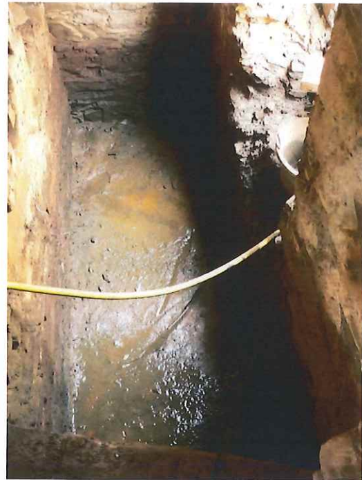
Internal cog pit after clearance
