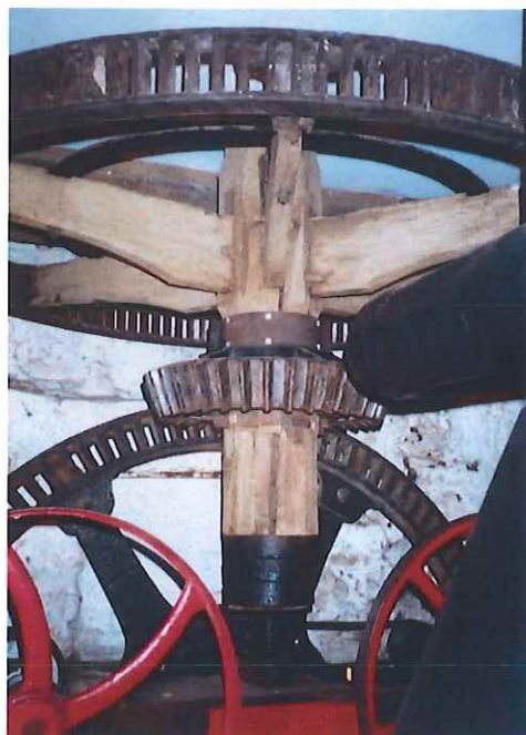
Iron gearing and timber upright shaft in Town Mill, Okehampton, Devon, probably that from Lew Mill 30 October 1993 Martin Watts
