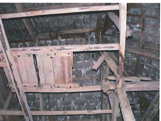
Remains of hoist and sack platform in roof
