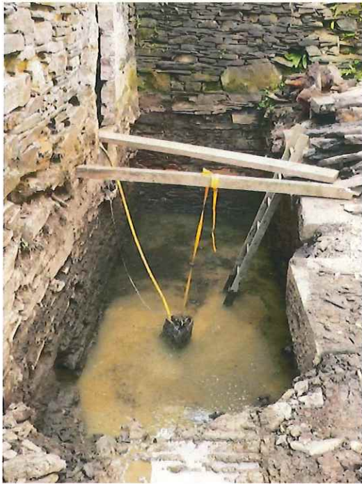
Upstream end of wheelpit during excavation July 2011
