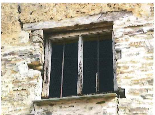
1st floor window, west elevation (north)
