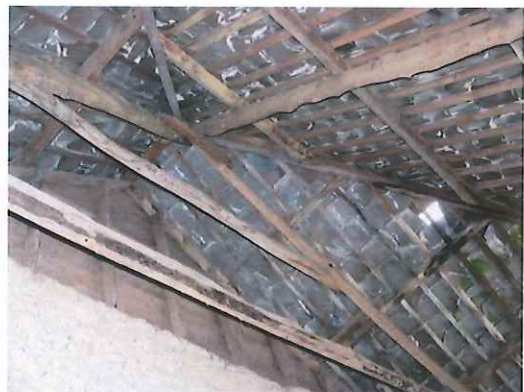
Mill east wall and roof from north-west
