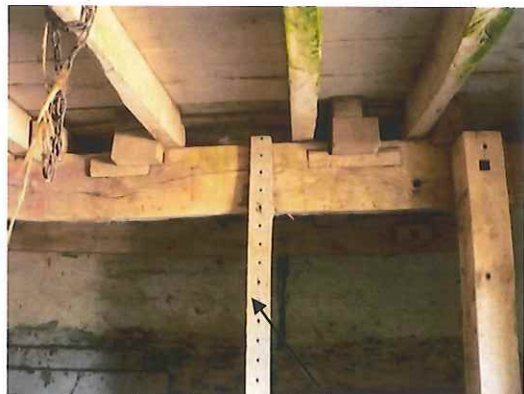
Hurst, north end. Possible tenter beam reused
