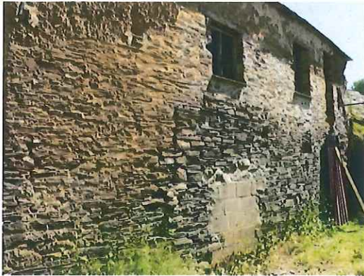
Wheelpit area prior to excavation, June 2010
