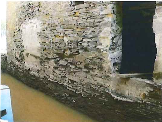
West wall and excavated wheelpit, flooded, August 2011
