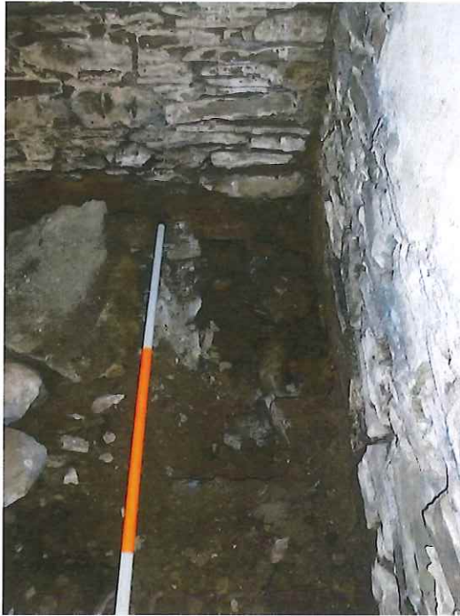
Drain in south-east corner, mill ground floor
