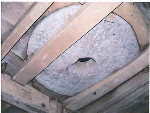
Beams supporting conglomerate millstone
