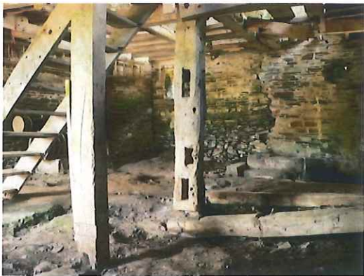
Mill, ground floor looking south, under hurst
