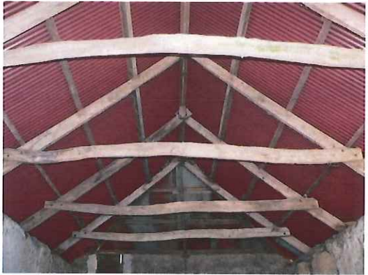
Roof of cider barn, looking south
