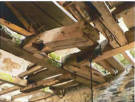
Bearing point for upright shaft
