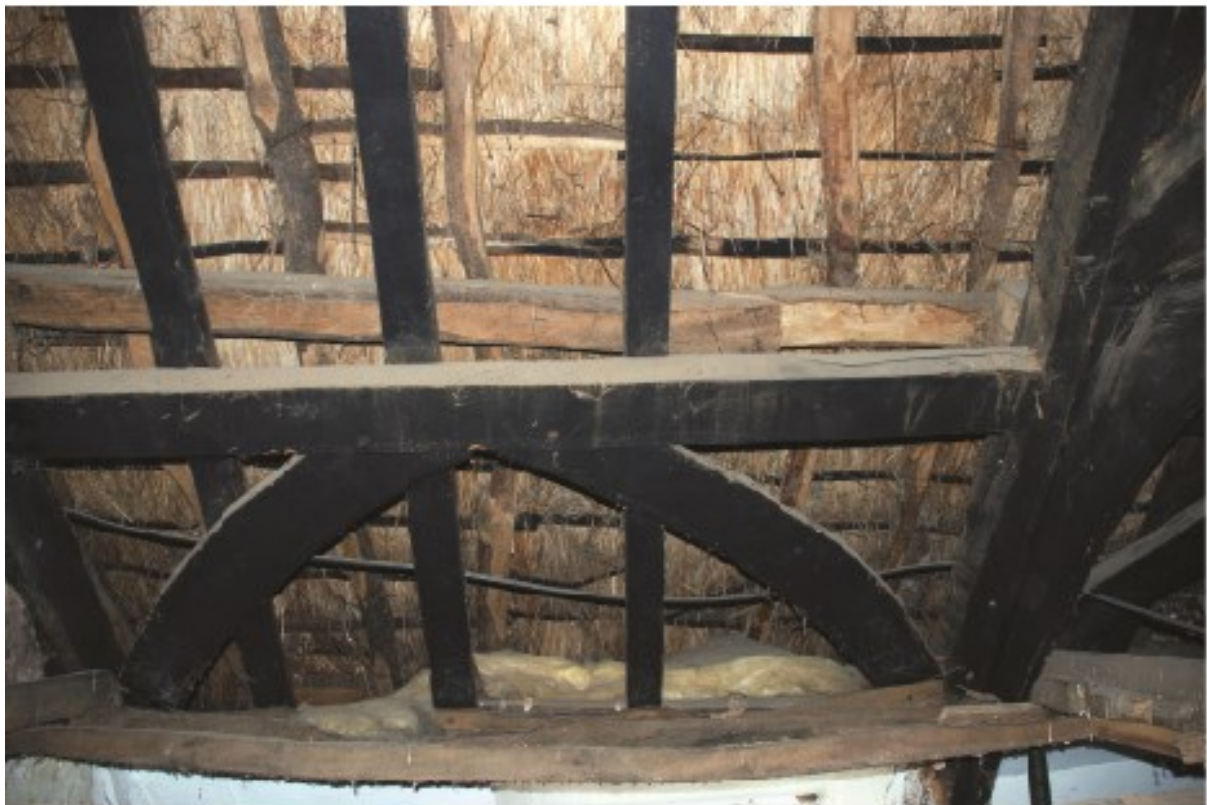
Plate 8 Windbraces beneath lower purlin, looking south.
