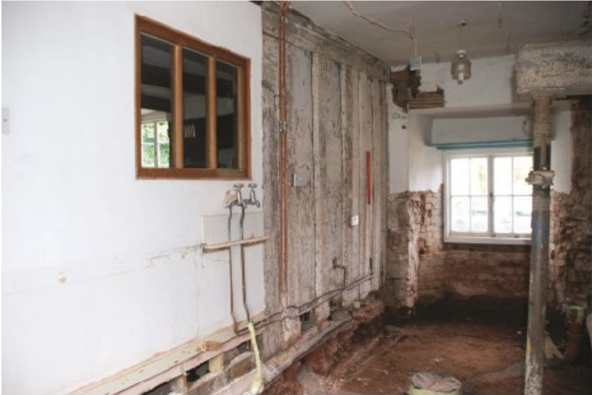
Plate 19 The screen on the upper, hall side of the passage, looking northwest.
