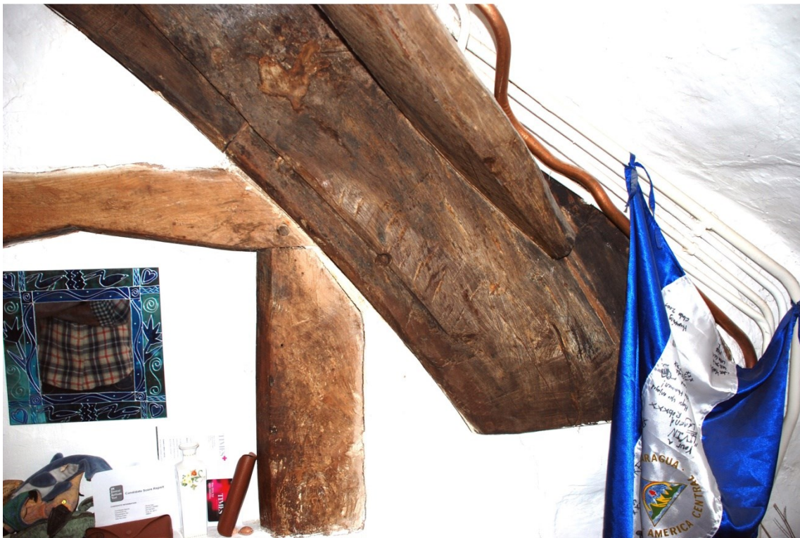
Plate 4 Elbow of probable true cruck truss over former hall, looking west.
