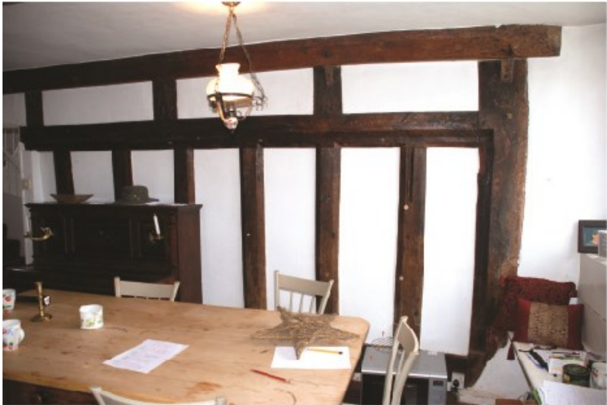
Plate 11 Screen at the bottom of the full height partition between hall and inner room, showing pegged joint to truss (to right), looking southwest.
