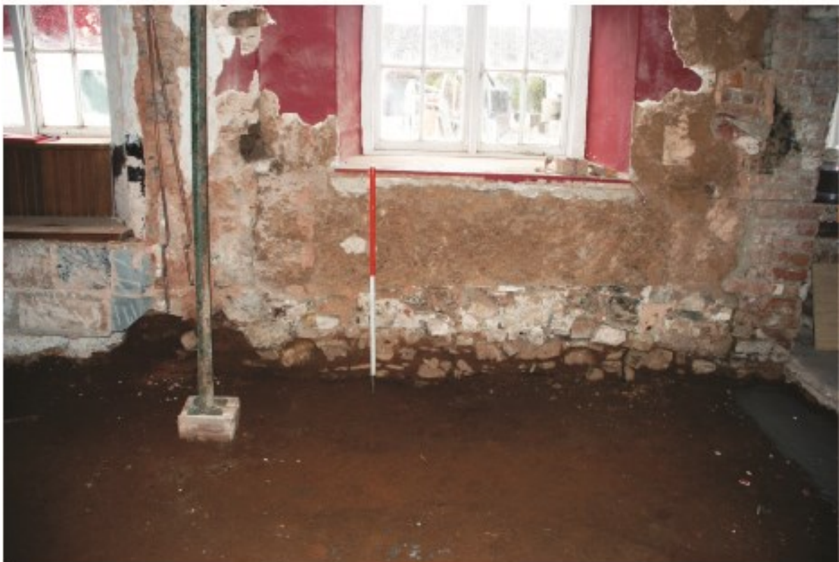
Plate 14 Trench-dug stone rubble footings exposed beneath the north wall, looking north.
