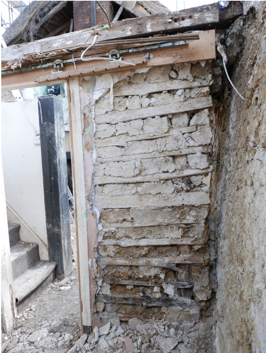
Lath and daub partition wall in Number 2.
