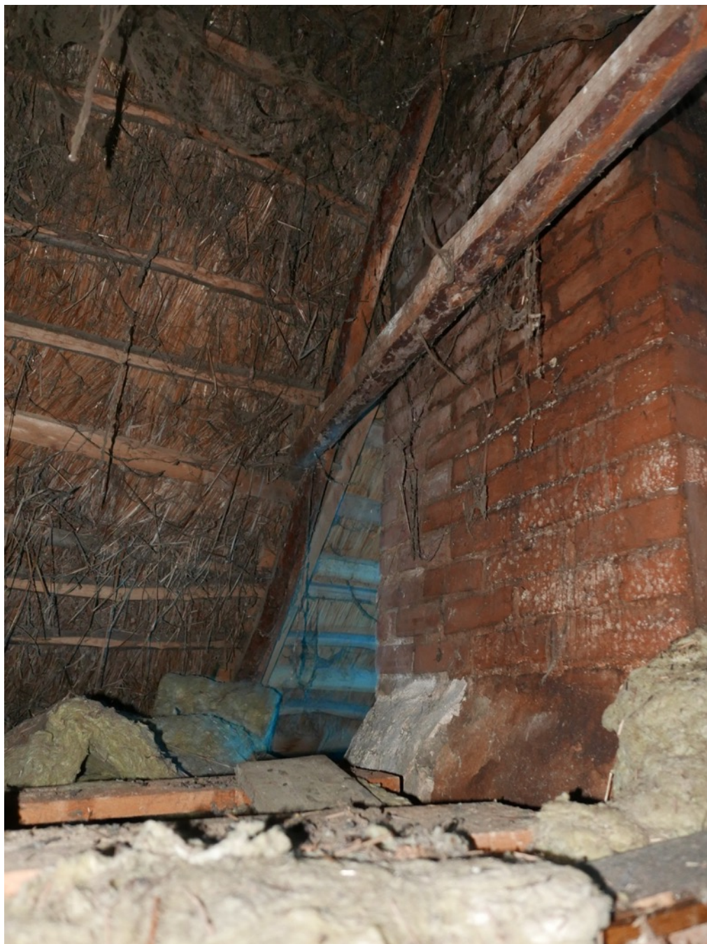
Chimney of Number 1 from within loft space.
