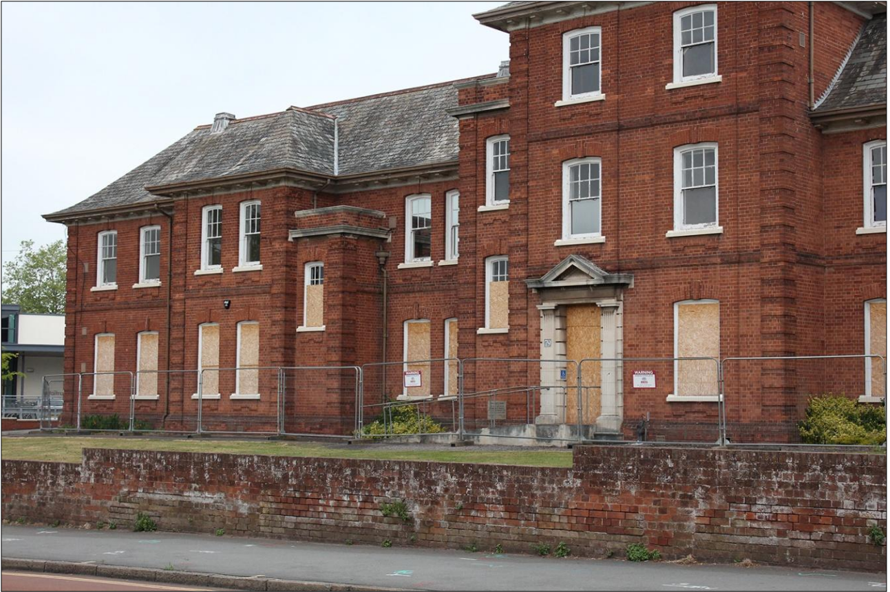
3. FRONT (SOUTH-WEST) EXTERNAL ELEVATION OF BUILDING, WEST END; VIEWED FROM THE SOUTH-EAST.
