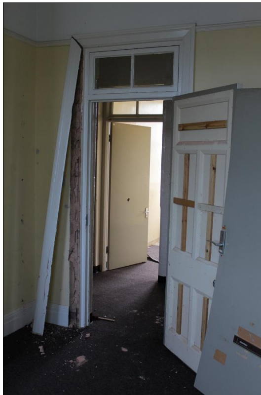
66. VIEW OF THE DOOR IN THE NORTH-EAST WALL OF ROOM F25, DEMONSTRATING IT TO BE A 1913 ORIGINAL; VIEWED FROM THE SOUTH-EAST.
