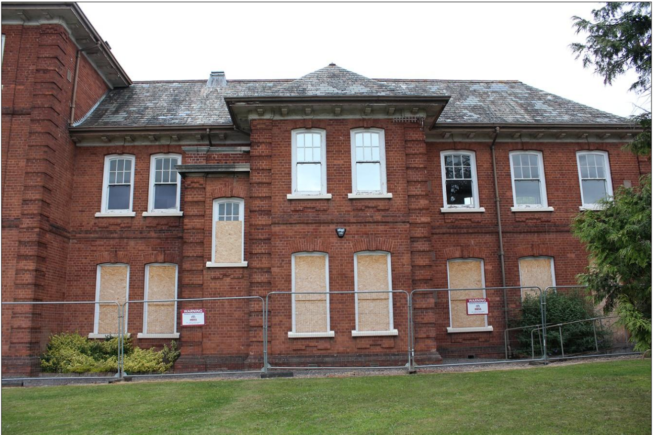
27. FRONT (SOUTH-WEST) EXTERNAL ELEVATION OF BUILDING, EAST END; VIEWED FROM THE SOUTH-WEST.
