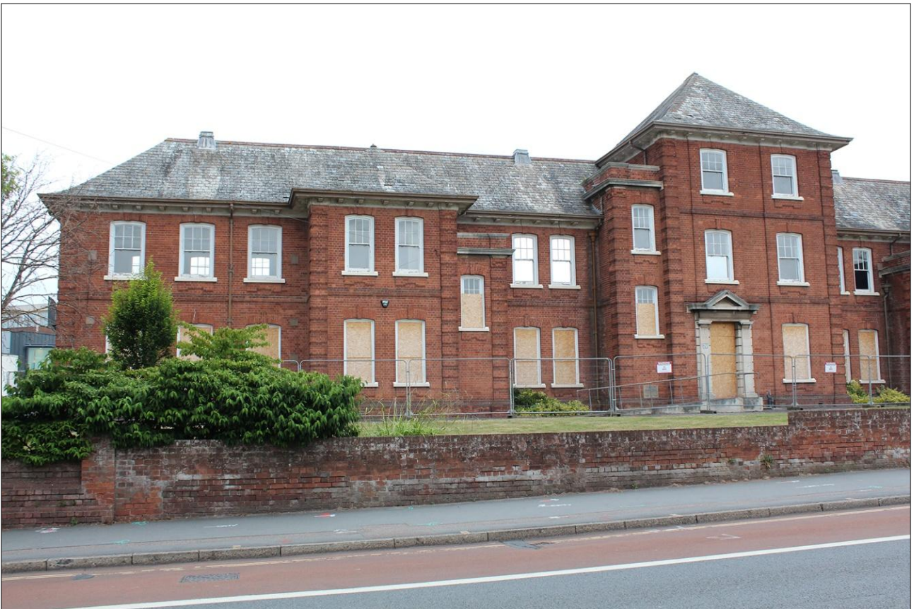
2. FRONT (SOUTH-WEST) EXTERNAL ELEVATION OF BUILDING, WEST END; VIEWED FROM THE SOUTH-WEST.
