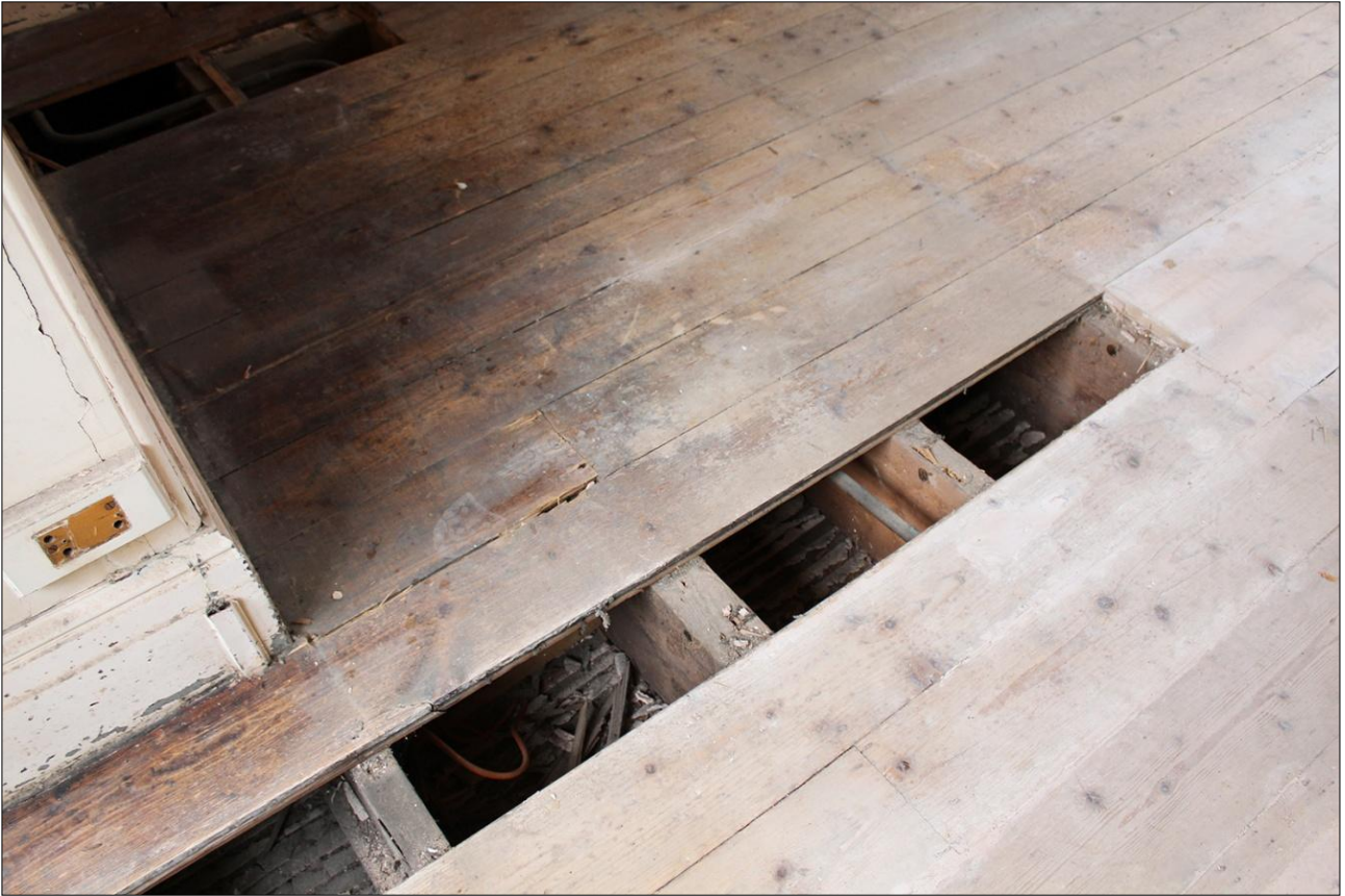
101. DETAIL OF THE FLOORBOARDS IN ROOM S7; VIEWED FROM THE SOUTH-WEST.
