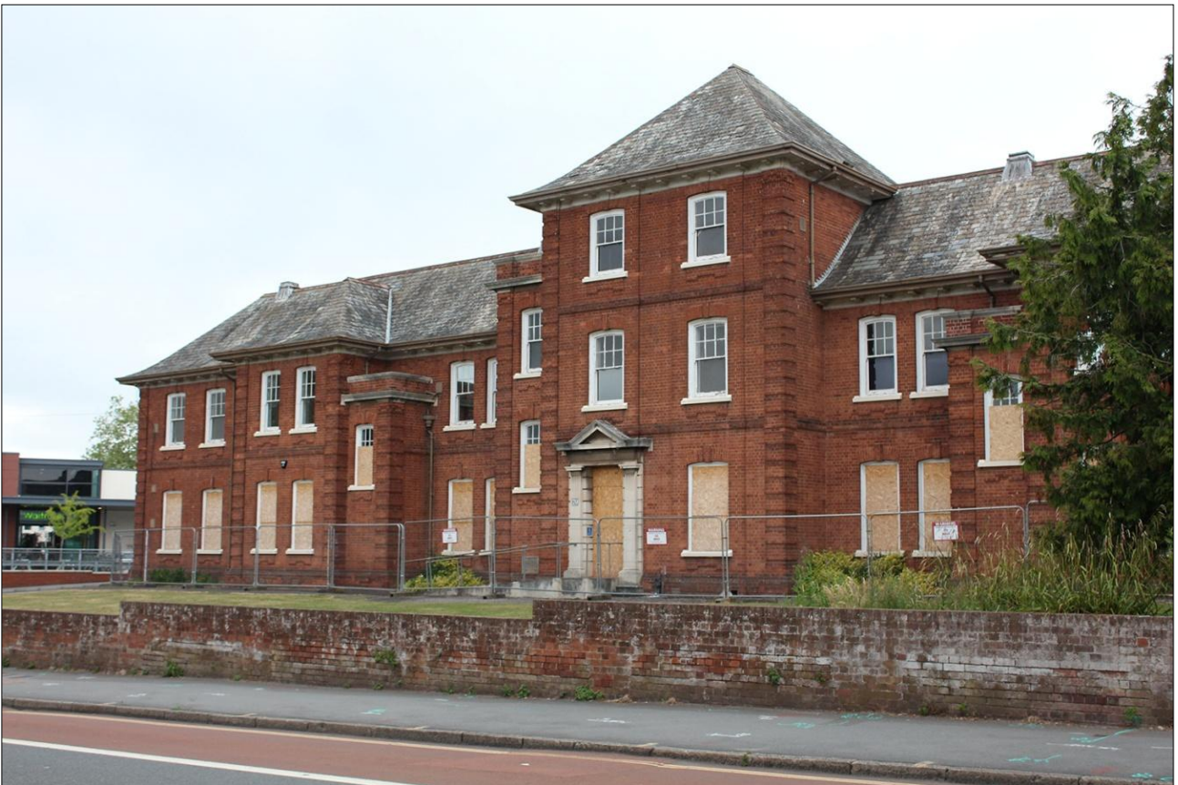
4. FRONT (SOUTH-WEST) EXTERNAL ELEVATION OF BUILDING; VIEWED FROM THE SOUTH-WEST.
