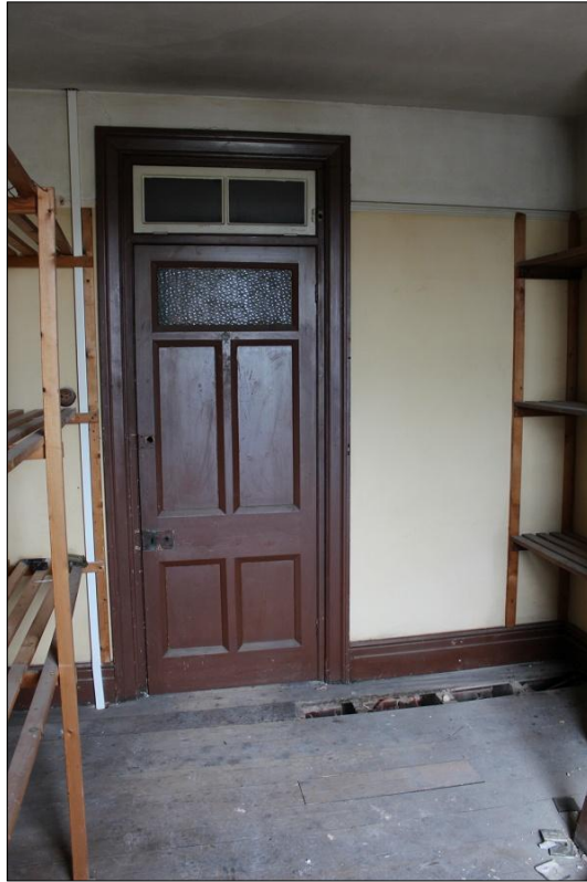
80. VIEW OF ROOM S6 SHOWING THE DOOR IN THE NORTH-EAST WALL; VIEWED FROM THE SOUTH-WEST.
