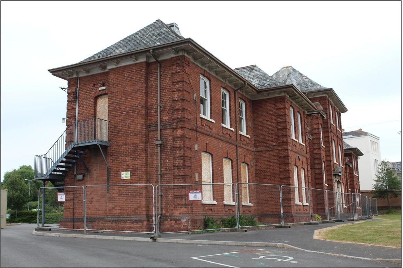
21. NORTH-WEST AND FRONT (SOUTH-EAST) EXTERNAL ELEVATIONS OF BUILDING; VIEWED FROM THE WEST.
