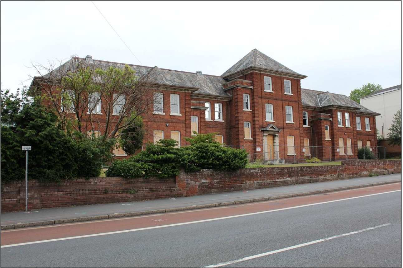
1. FRONT (SOUTH-WEST) EXTERNAL ELEVATION OF BUILDING; VIEWED FROM THE SOUTH-WEST.
