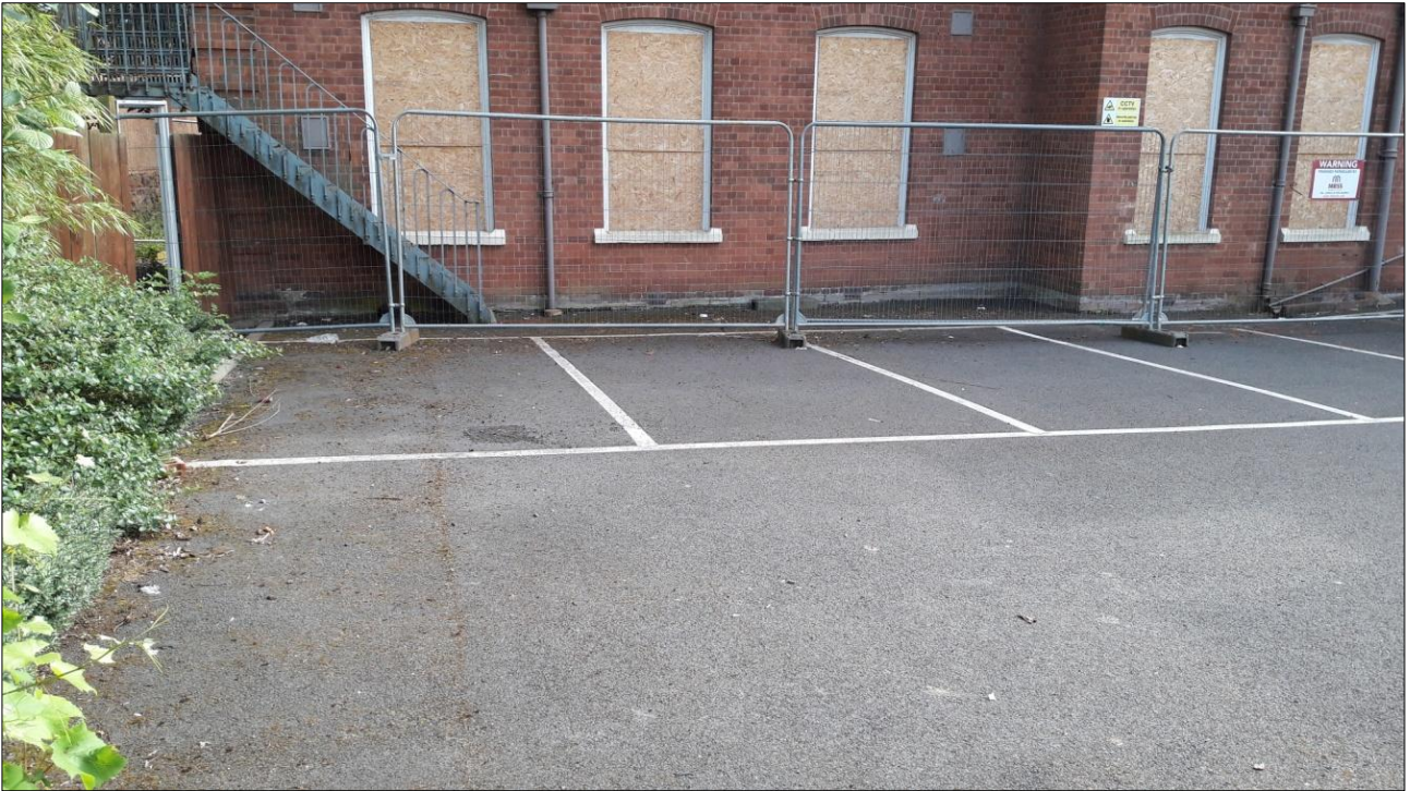
1. CAR PARK AREA TO REAR (NORTH) OF BUILDING, EAST END; VIEWED FROM THE NORTH-EAST (NO SCALE).
