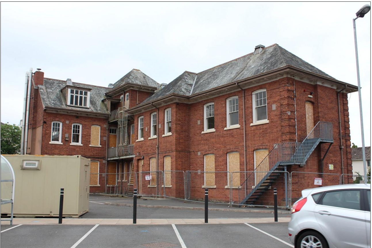
18. REAR (NORTH-EAST) EXTERNAL ELEVATION OF BUILDING, WEST END; VIEWED FROM THE NORTH-WEST.
