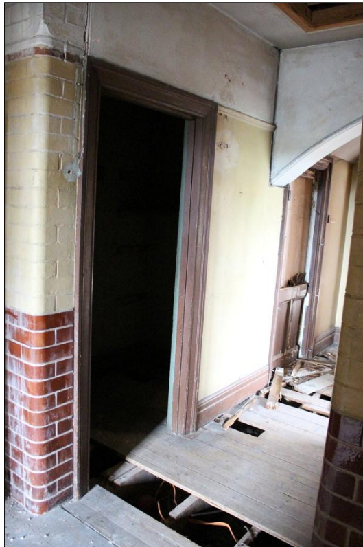
91. DETAIL OF THE DOOR OPENINGS IN THE NORTH-WEST WALL OF CORRIDOR S8; VIEWED FROM THE SOUTH-EAST.
