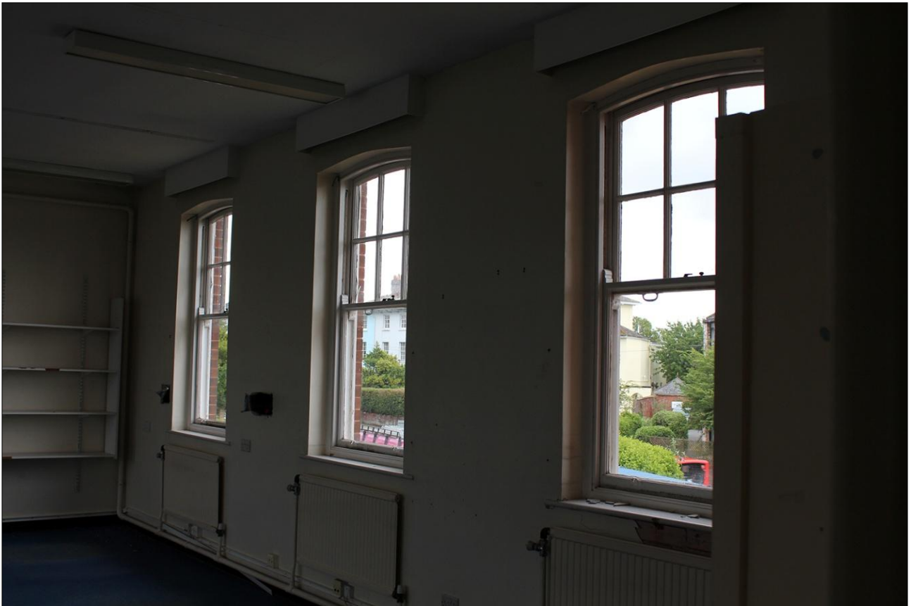
67. DETAIL OF WINDOW OPENINGS IN THE SOUTH-WEST WALL OF ROOM F26; VIEWED FROM THE NORTH-WEST.
