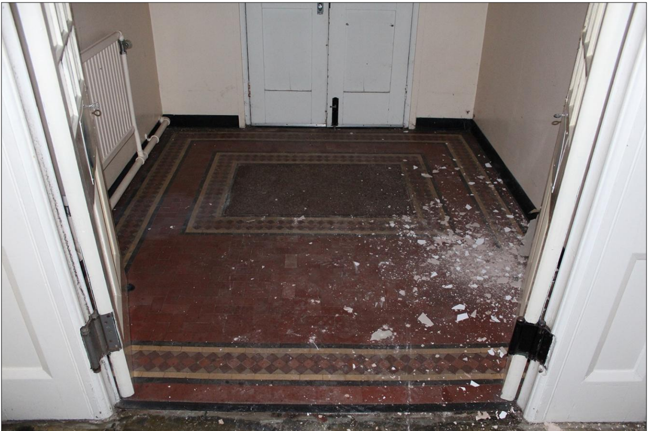
42. DETAIL OF FLOOR IN ROOM 22; VIEWED FROM THE NORTH-EAST.
