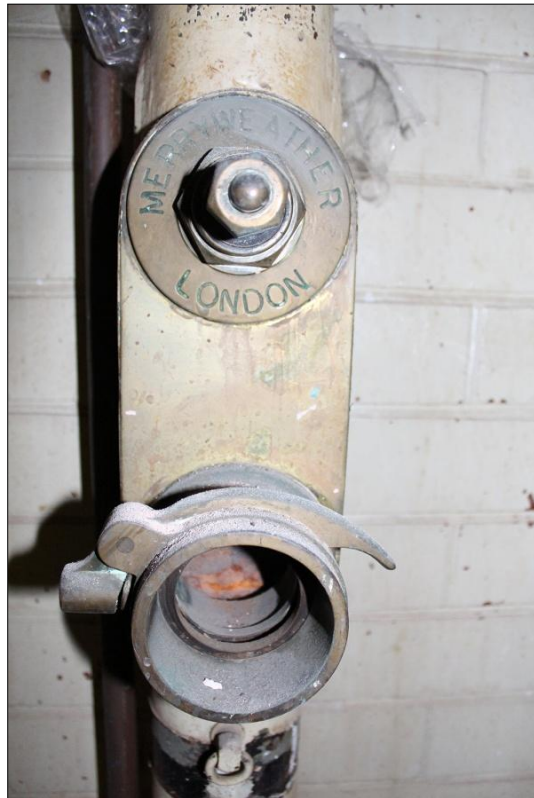
LEFT: 75. THE FIRE HYDRANT IN ROOM S3; VIEWED FROM THE WEST.
