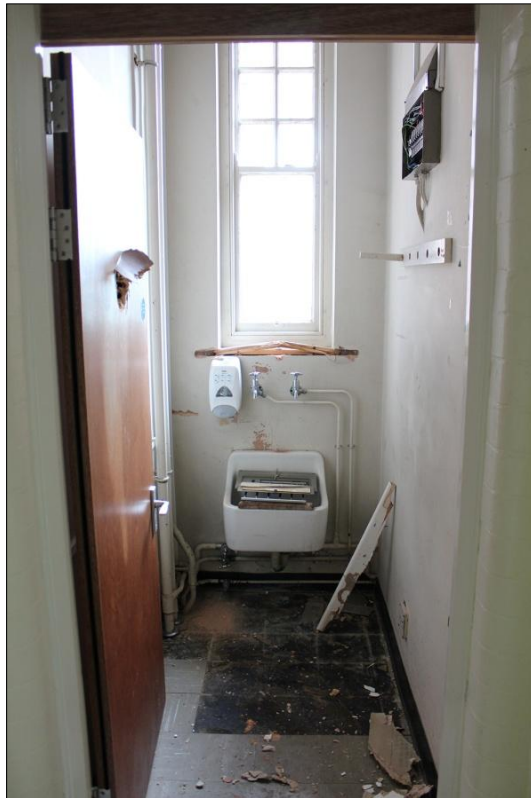
63. DETAIL OF F15 SHOWING INDICATING FORMER FUNCTION AS BATHROOM; VIEWED FROM THE SOUTH-WEST.
