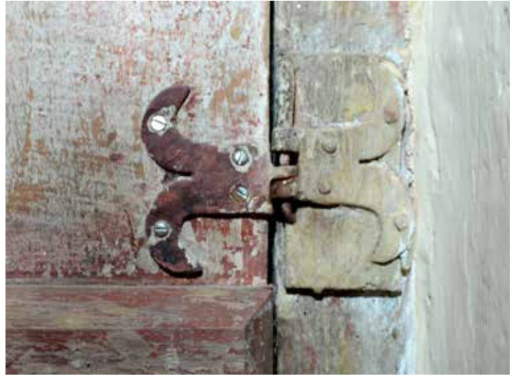
23. (Left) The double doorway to the eastern closets off the Great Chamber.
