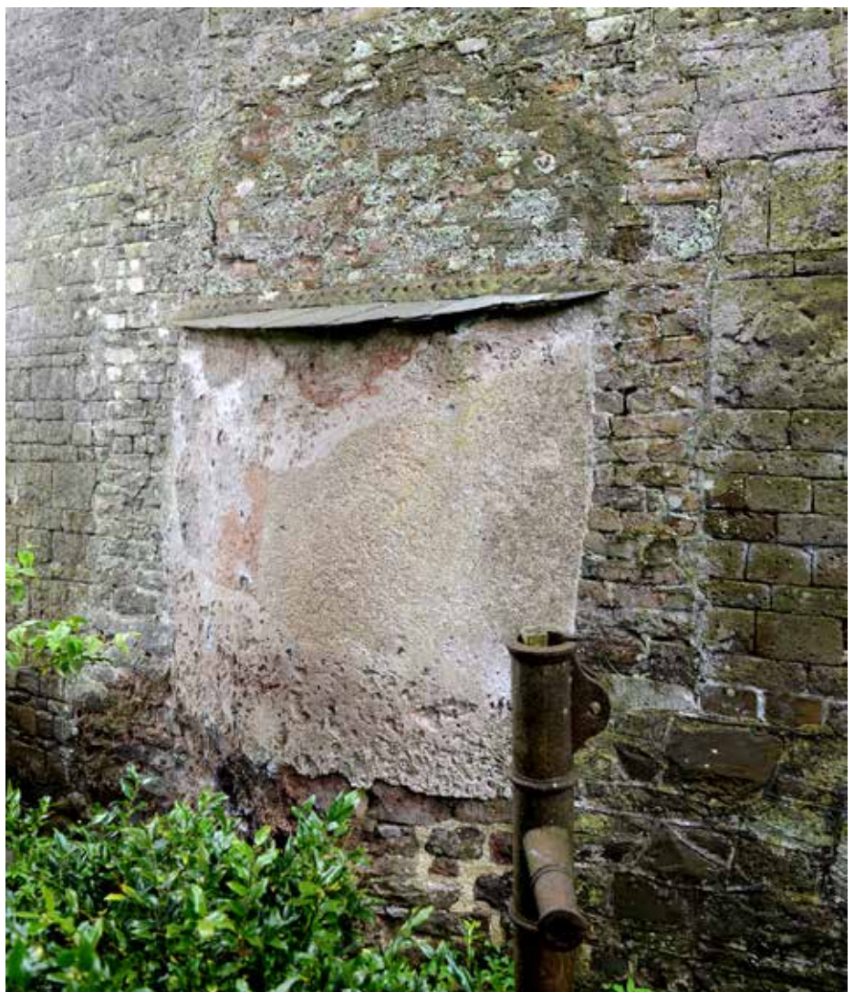
7. The oven housing within the blocking of an earlier feature associated with the kitchen fireplace.
