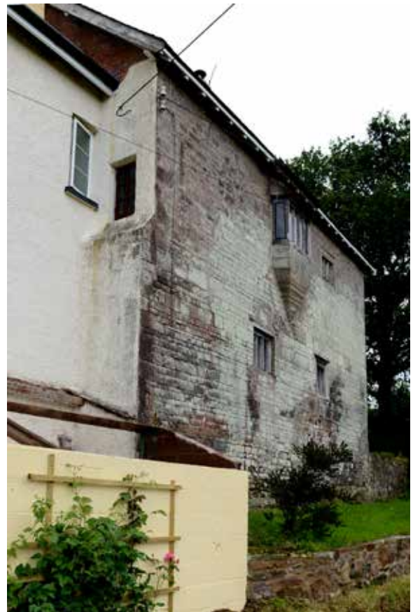
12. The south end from the east.
