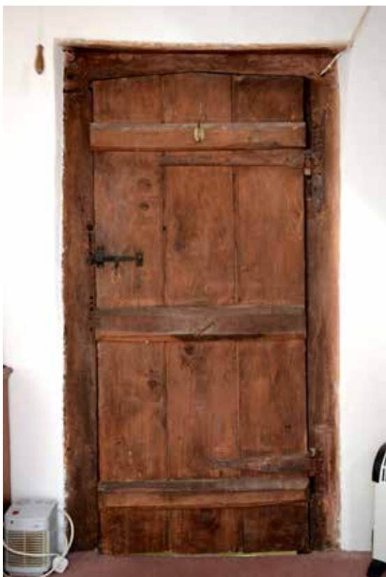
27. The door from the stair to the attic. During repairs to the adjacent wall plaster Gill Juleff noted that the studs were clad with primary laths clad with a base coat of mud plaster mixed with red cows hair finished with a skim of lime.
