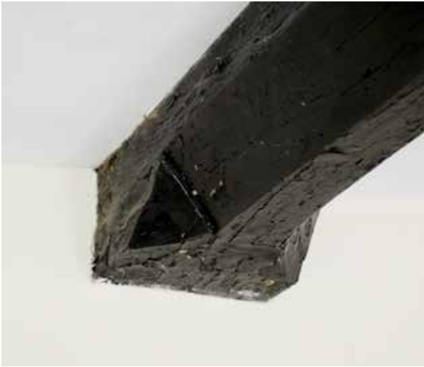
14. Detail of the chamfer and stop at the east end of the northern crossbeam
