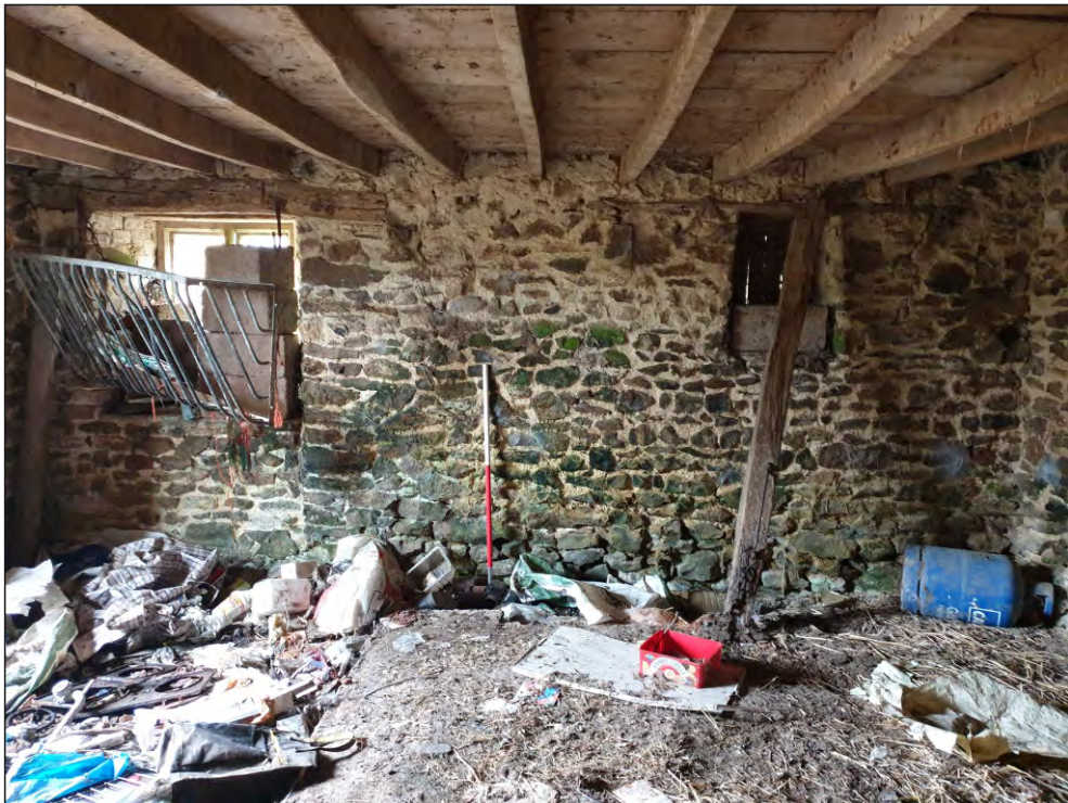
Pl. 38 General view of north elevation in G01 showing earlier door arrangement and narrow first-floor joists. 1m scale. Looking north.
