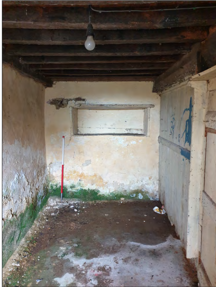
Pl. 15 General view of former corridor G03 showing position of partially blocked doorway re-using remains of former screen. 1m scale. Looking east.
