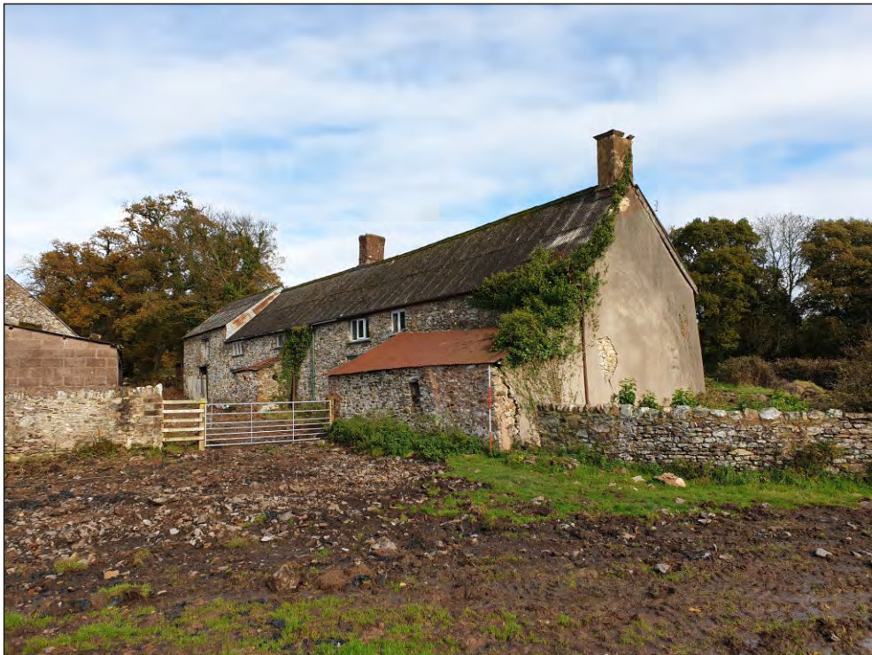
Pl. 4 General view of the farmyard elevation showing the Ham stone chimney at the southern end of the main range. 2m scale. Looking northeast.
