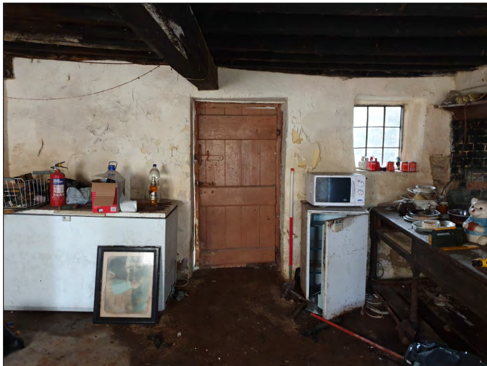
Pl. 12 General view of east elevation in G02 showing plank door and window with leaded lights giving onto 19th century outshut extension G07. 1m scale. Looking east.
