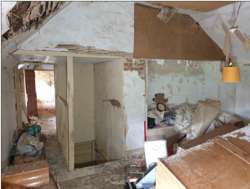
Pl. 32 General view of north elevation in F03 showing inserted chimney stack and stair, with corridor leading to F04 and F05. Looking north.
