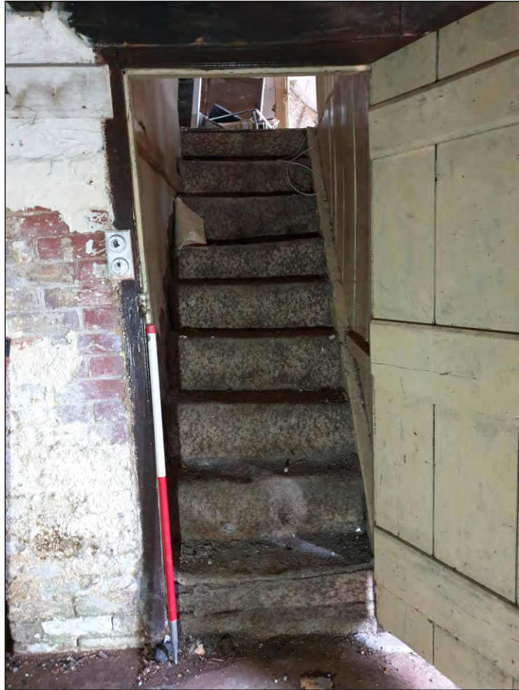
Pl. 11 Close-up of staircase leading to F03. 1m scale. Looking south.
