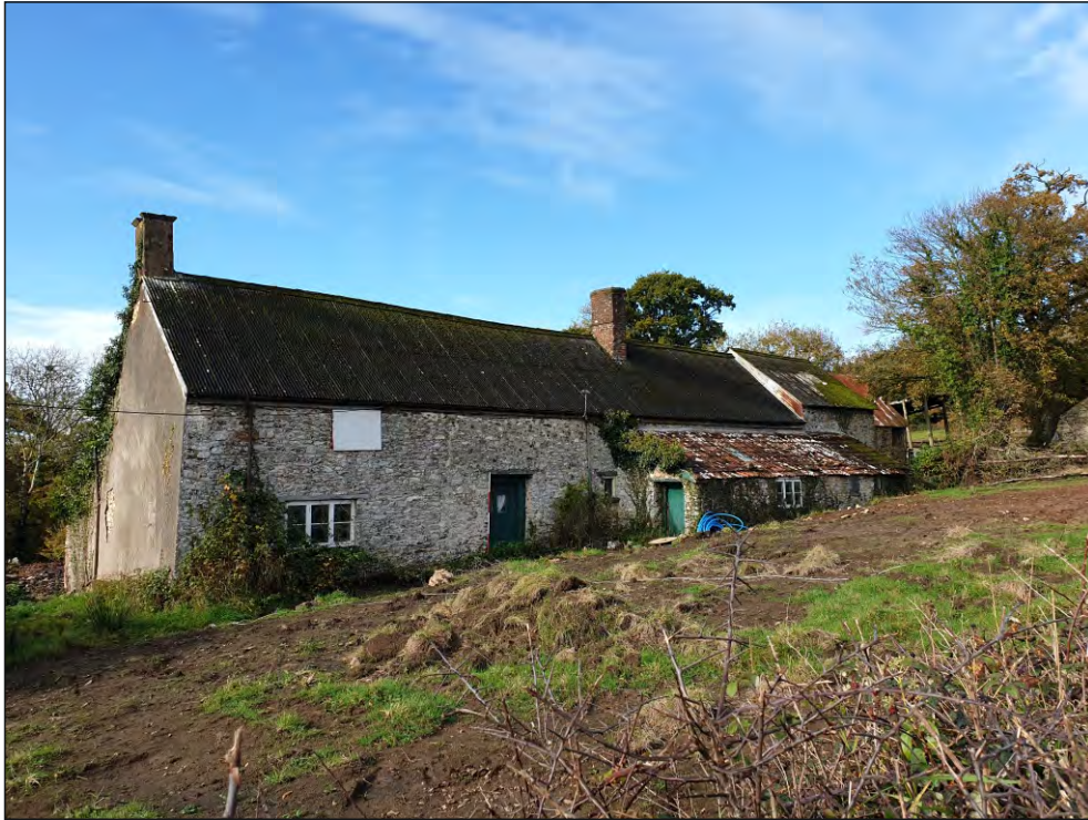
Pl. 1 General view of former main elevation showing Ham stone chimney, position of cross-passage and position of later outshut. 2m scale. Looking northwest
