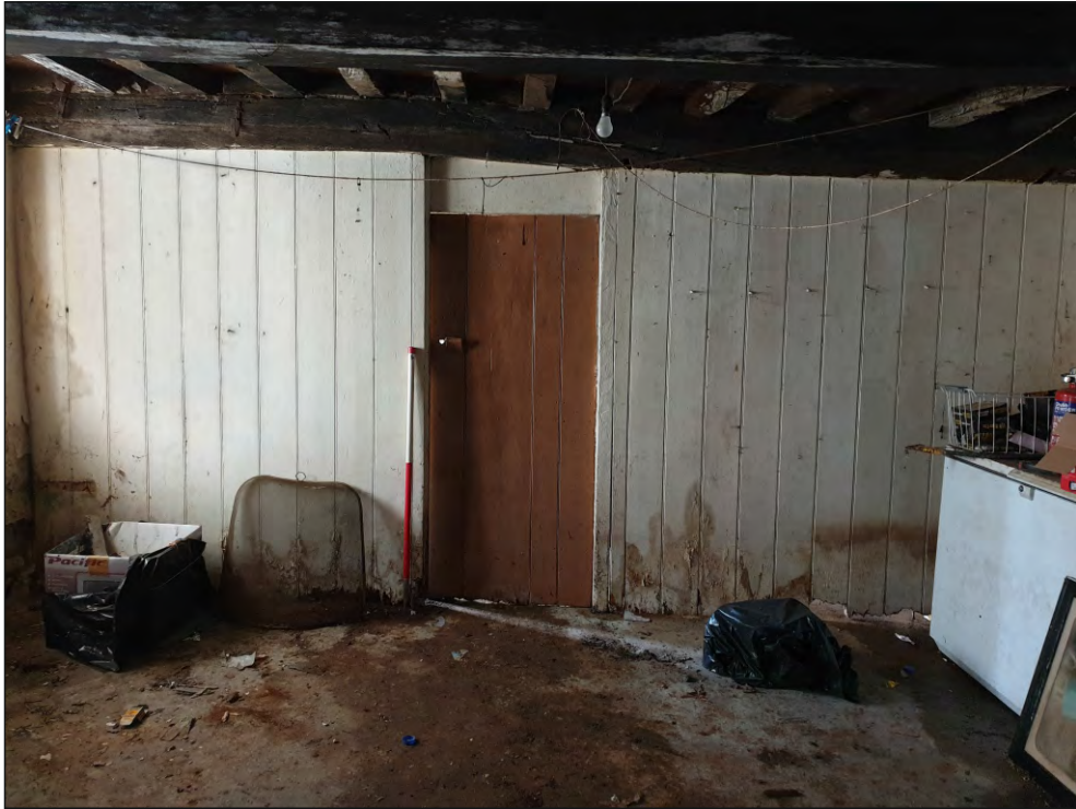
Pl. 13 General view of north elevation in G02 showing 19th century partition and doorway with original 17th century beam above. 1m scale. Looking north.
