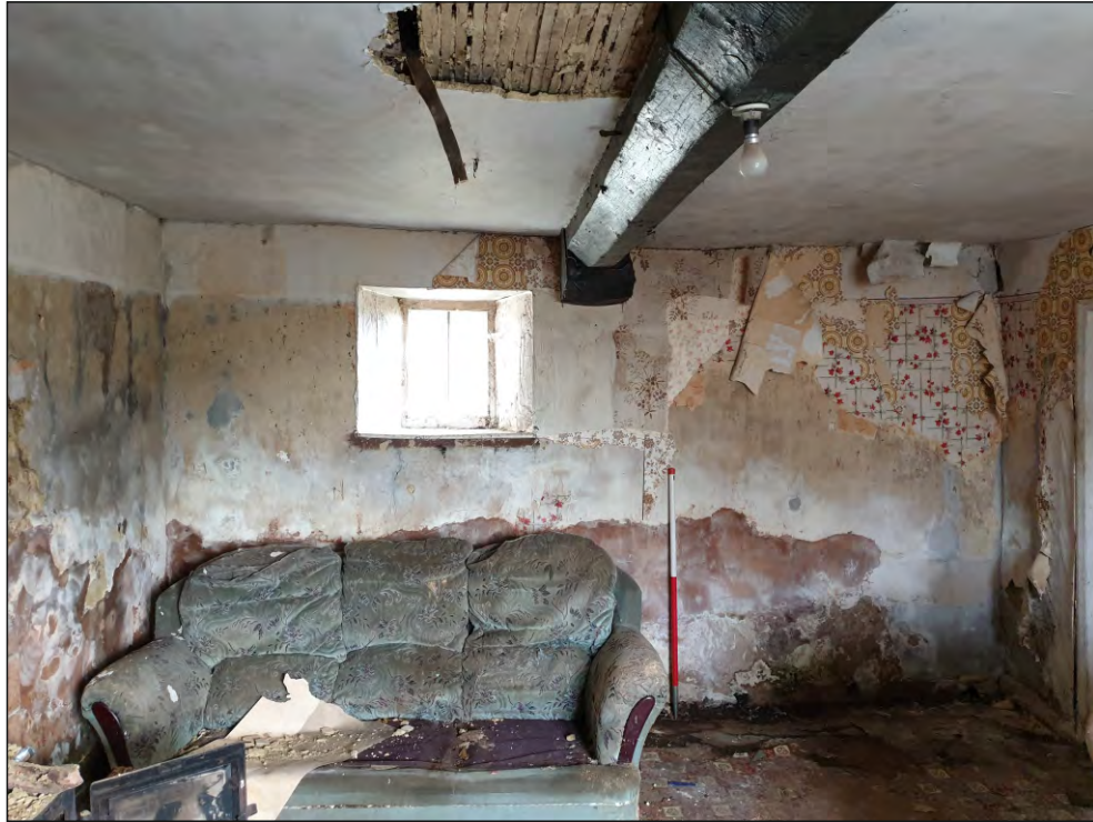
Pl. 17 General view of east elevation in G03 showing reduced wall width with the 17th century beam resting on a projecting bracket. 1m scale. Looking east.
