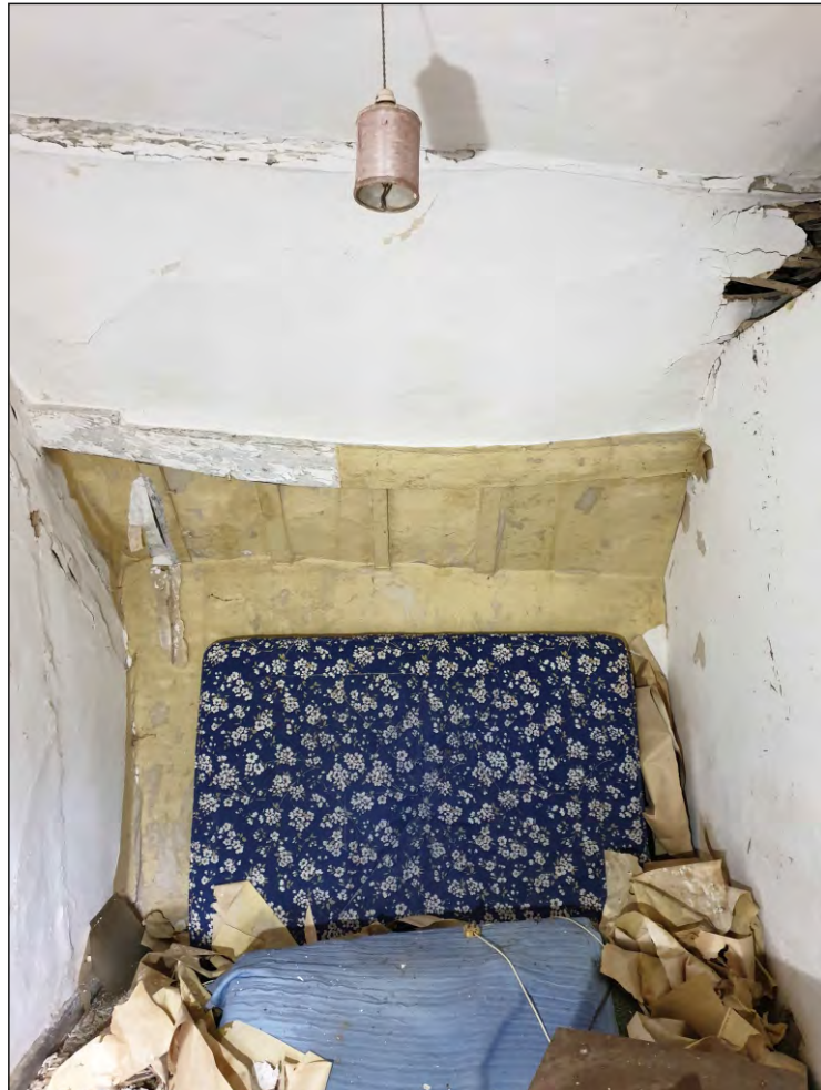
Pl. 36 General view of lower purlin with rafters in F04. Looking east.
