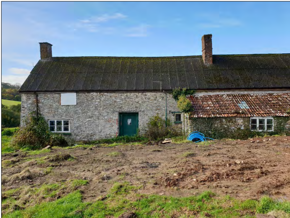
Pl. 2 Close-up of south end showing ground- and first floor fenestration, position of cross-passage with 17th century doorway and the 19th century outshut extension. 2m scale. Looking west.
