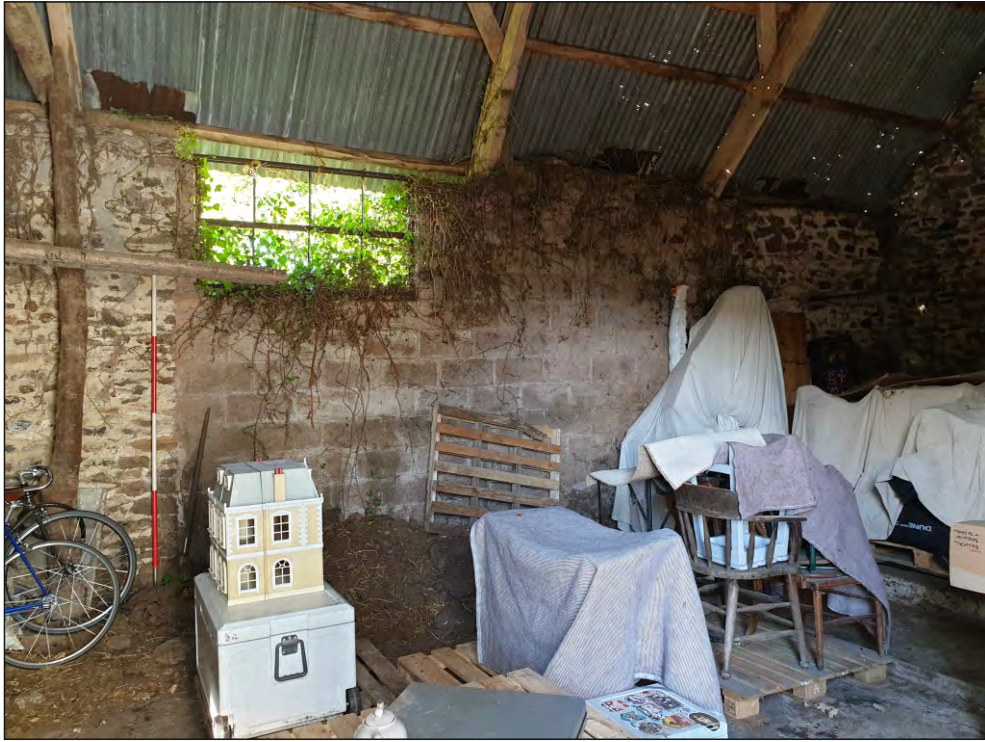
Pl. 45 General view of former west doorway. 2m scale. Looking west.
