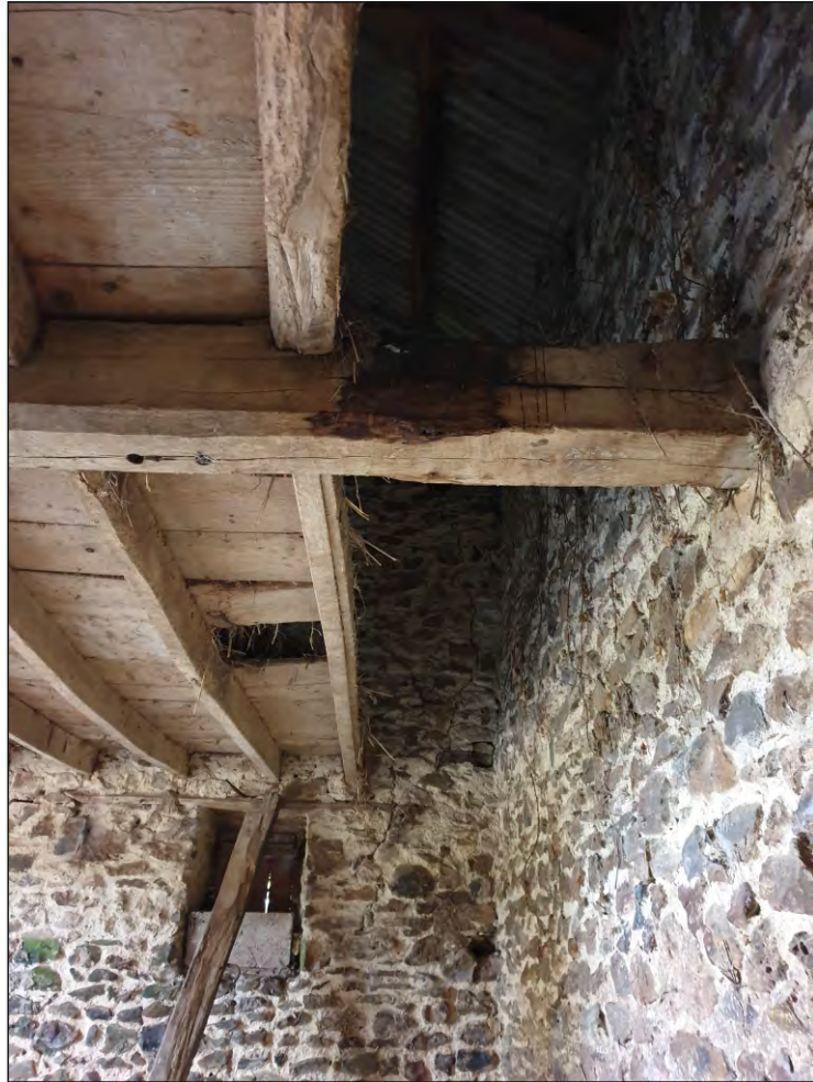
Pl. 39 Close-up of first-floor structure in G01 showing feeding void. Looking north.
