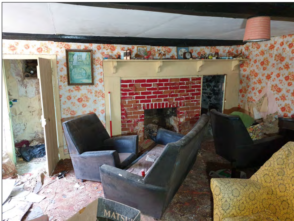
Pl. 24 General view of south elevation in G06 showing modern fireplace. This was formerly the kitchen and subsequently the parlour fireplace and occupied most of the gable elevation while the small cupboard to the left is the possible position of a former staircase. 1m scale. Looking south.
