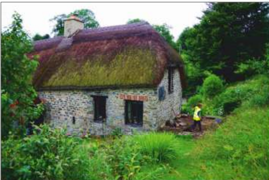
Plate 3: Excavation in progress, looking northwest
