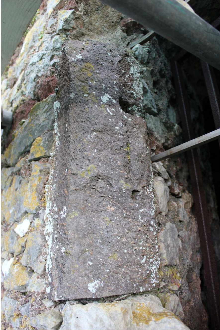
Fig. 12: St Michael's Chapel, higher west window, detail of north jamb.
