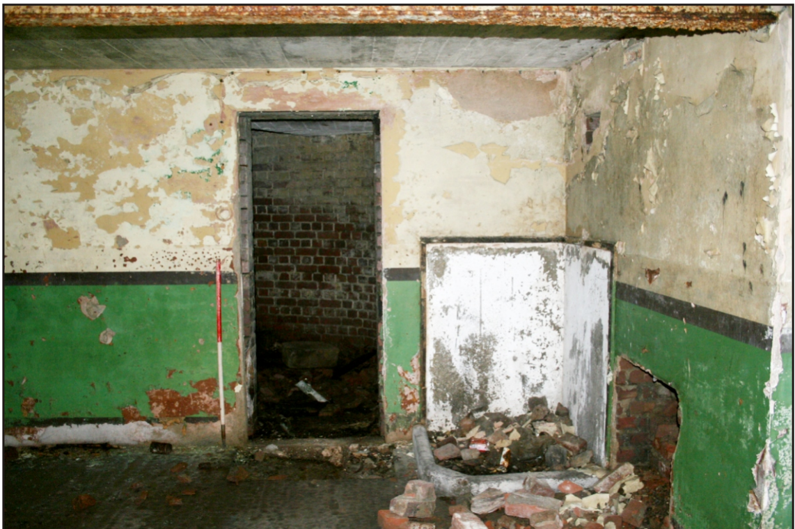
Plate 3 No. 2 gun crew war shelter showing door opening and stove base, looking south-east. 1m scale.
