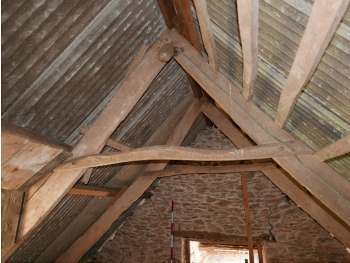
Plate 37. Interior. Roof south end looking north.
