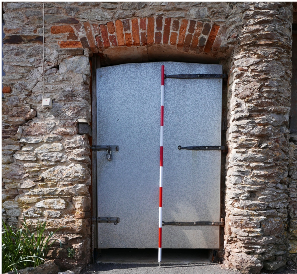
Plate 9. Bay 2 metal door with hand-forged hinges, east elevation.
