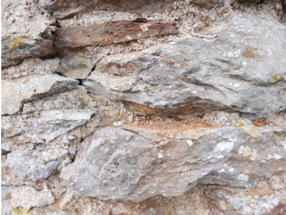
Plate 6. East elevation showing bedding and pointing mortar.
