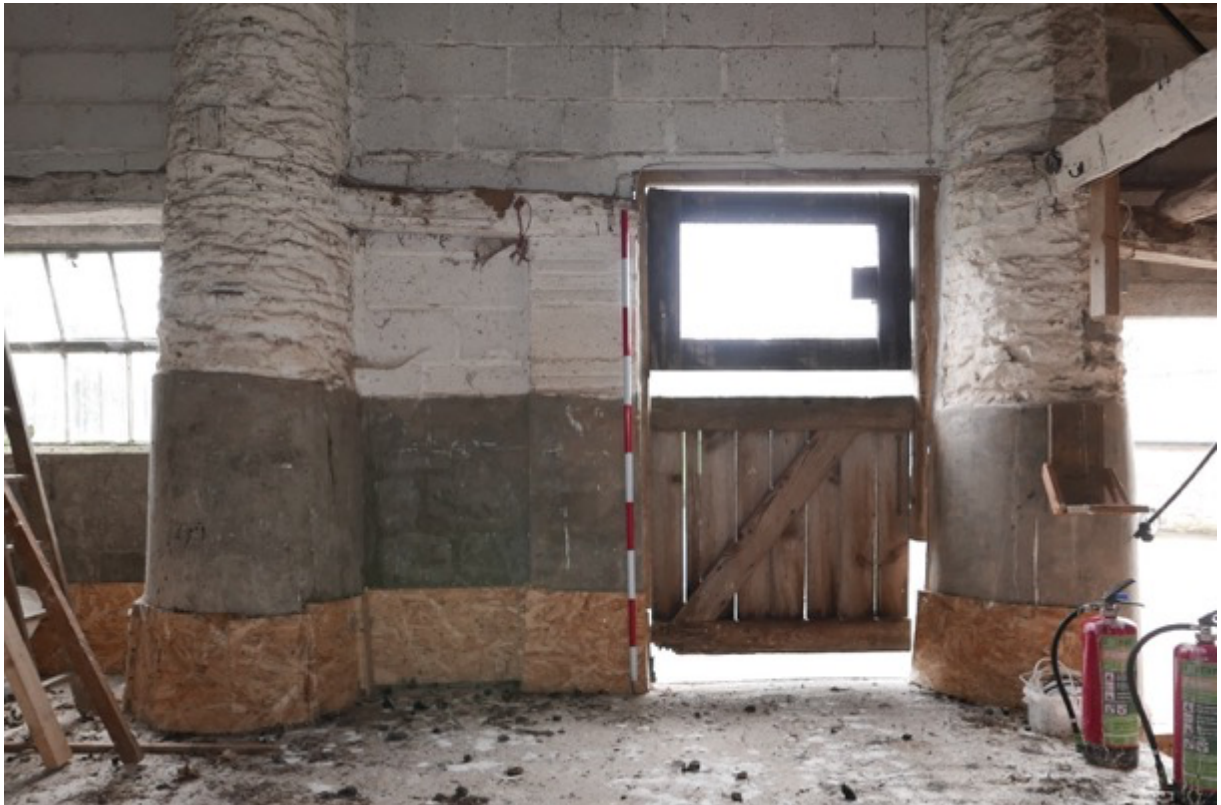
Plate 31. Interior. North end Bay 6.
