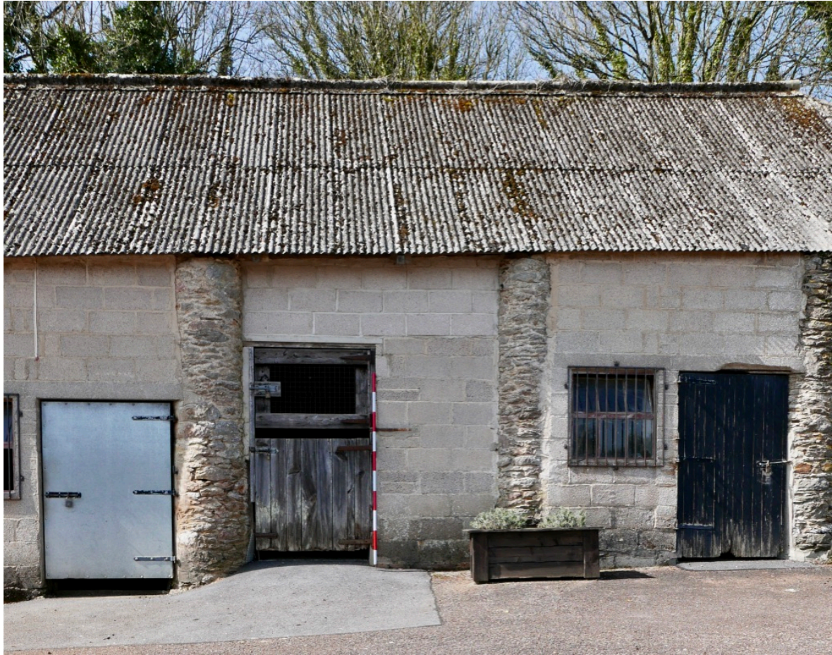
Plate 15. East elevation, Bay 6.
