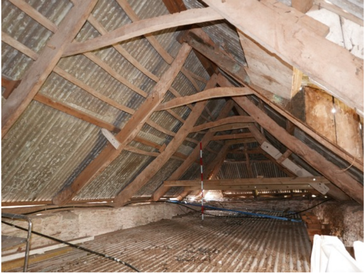
Plate 33. Interior. Upper floor south end looking SE.
