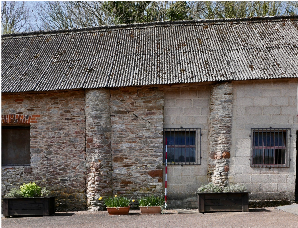
Plate 13. East elevation, Bay 4.
