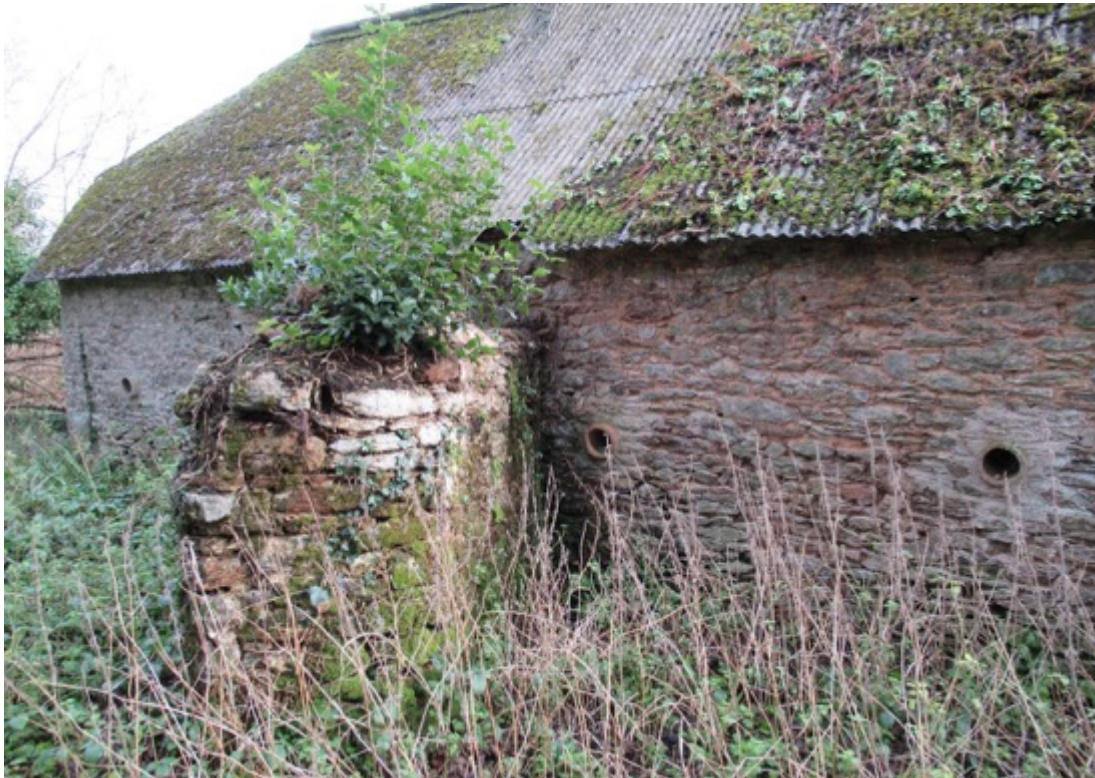
Plate 22. West elevation showing projecting gate pier and earthenware drain pipes.
