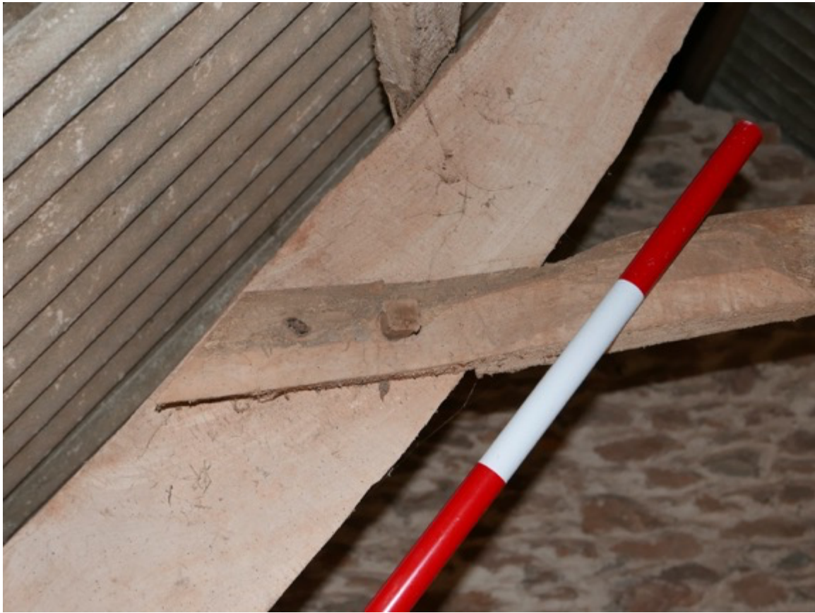
Plate 39. Interior. Roof south end collar detail.
