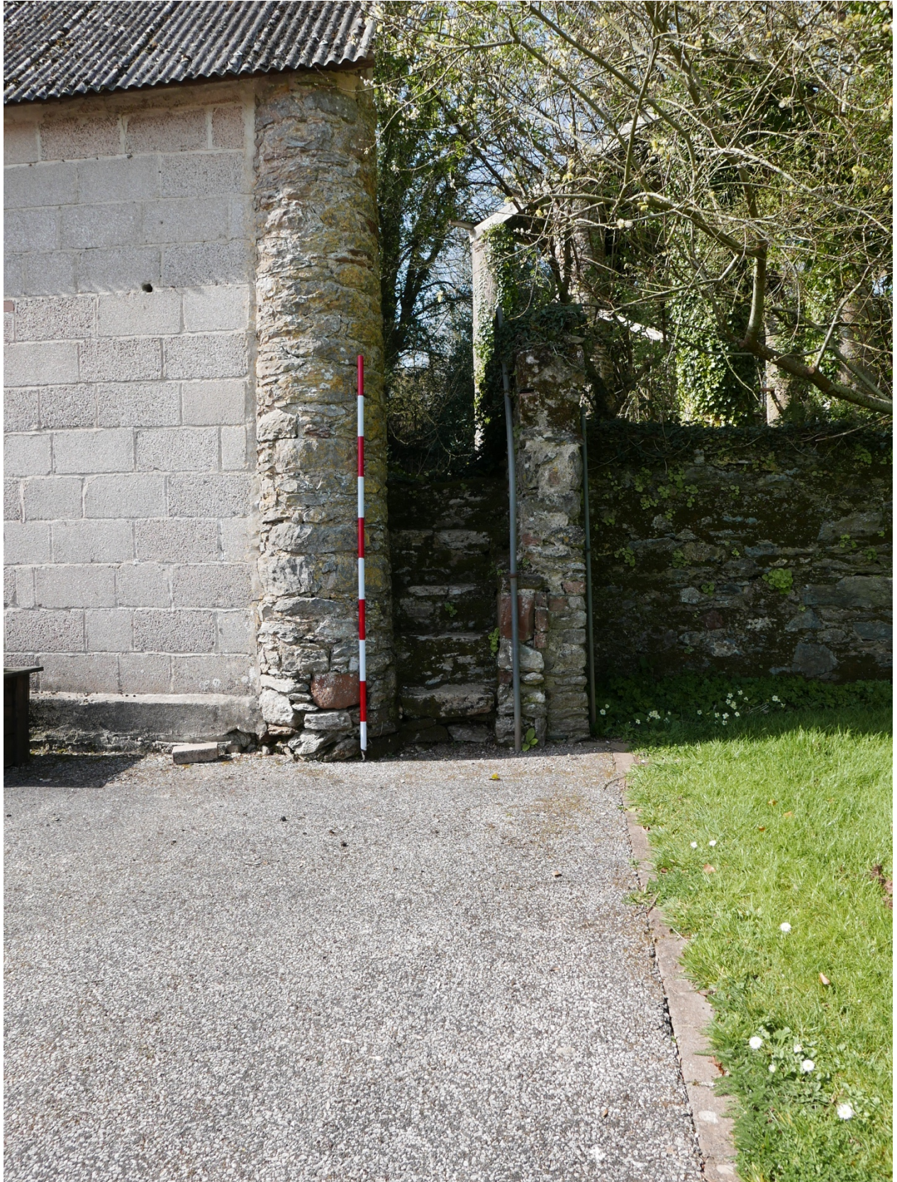
Plate 3. Sandridge Barton Linhay. Stair at NE corner.
