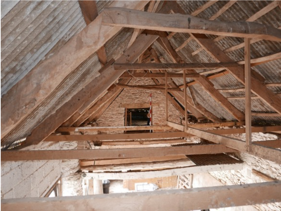
Plate 35. Interior. Upper floor north end looking south towards cross wall.
