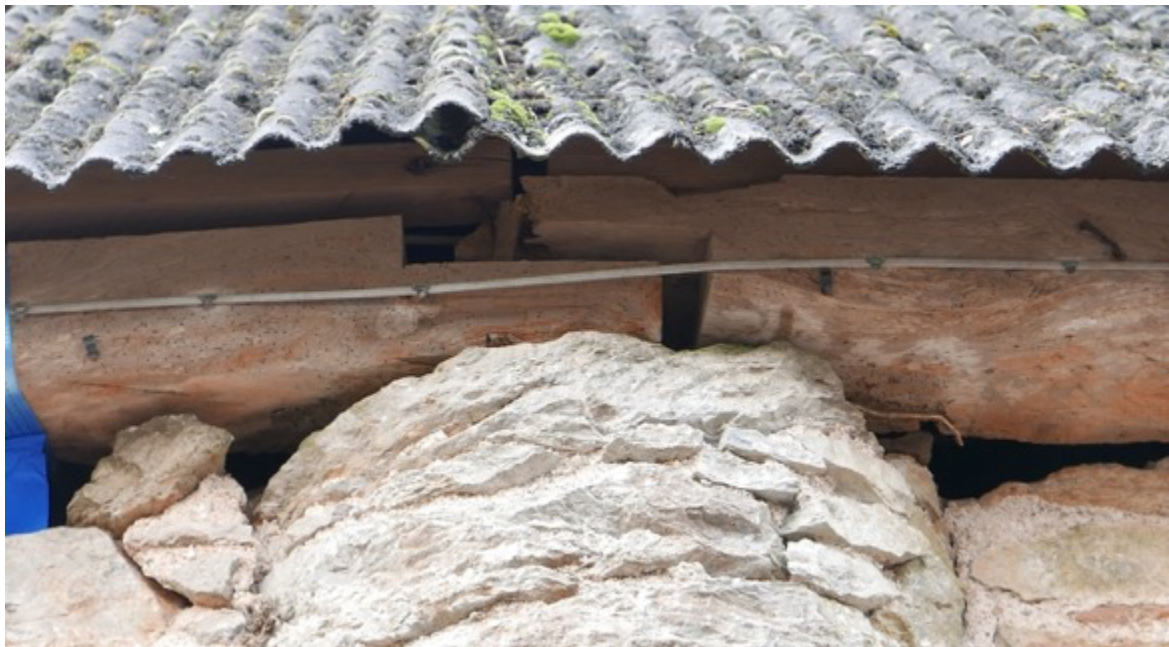
Plate 42. East elevation. Jointed wall plate over pier.
