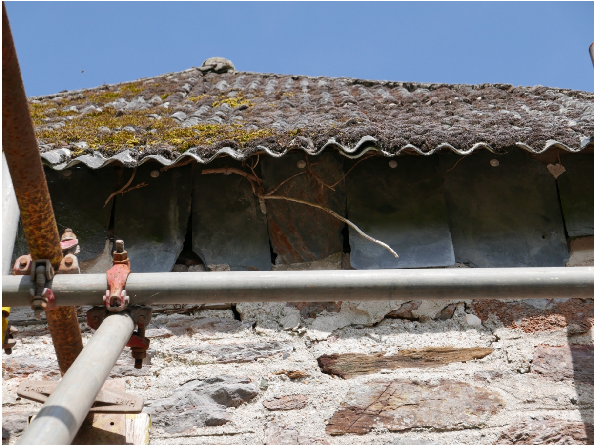
Plate 20. South elevation showing slates under eaves.
