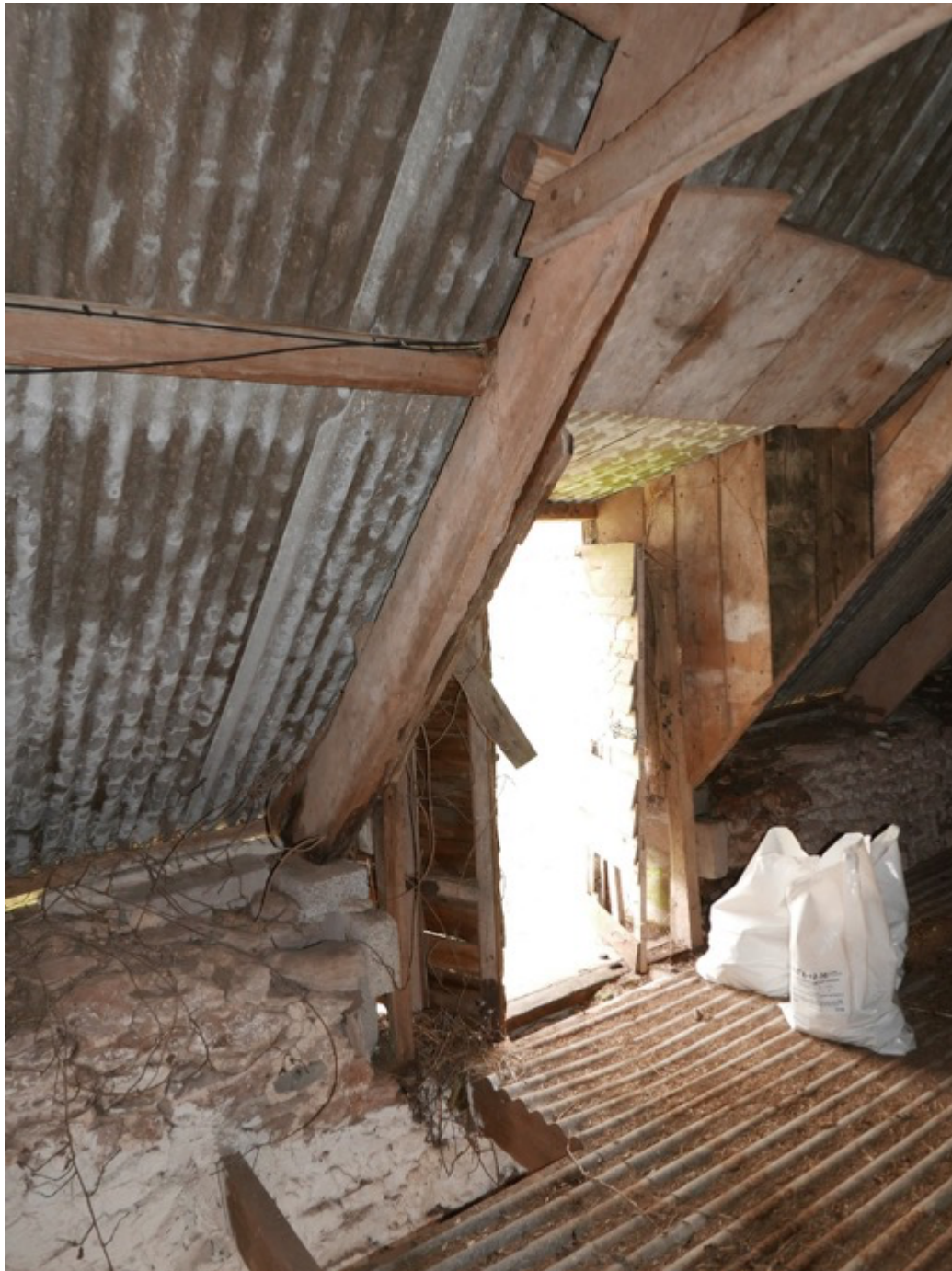
Plate 34. Interior. Upper floor south end. West elevation pitching door.
