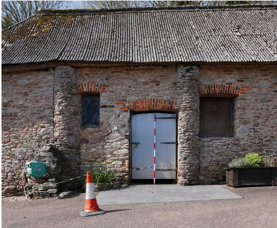
Plate 8. East elevation, Bay 2.
