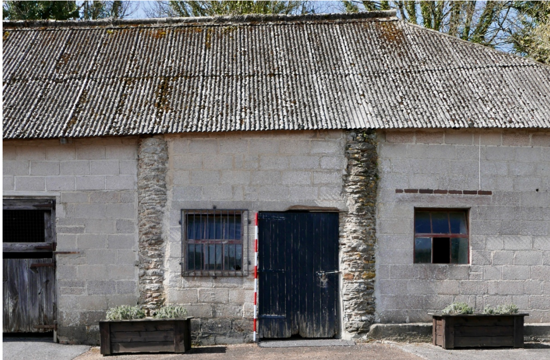
Plate 16. East elevation, Bay 7.
