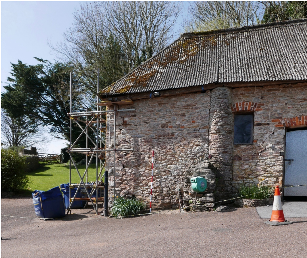
Plate 7. East elevation, Bay 1.
