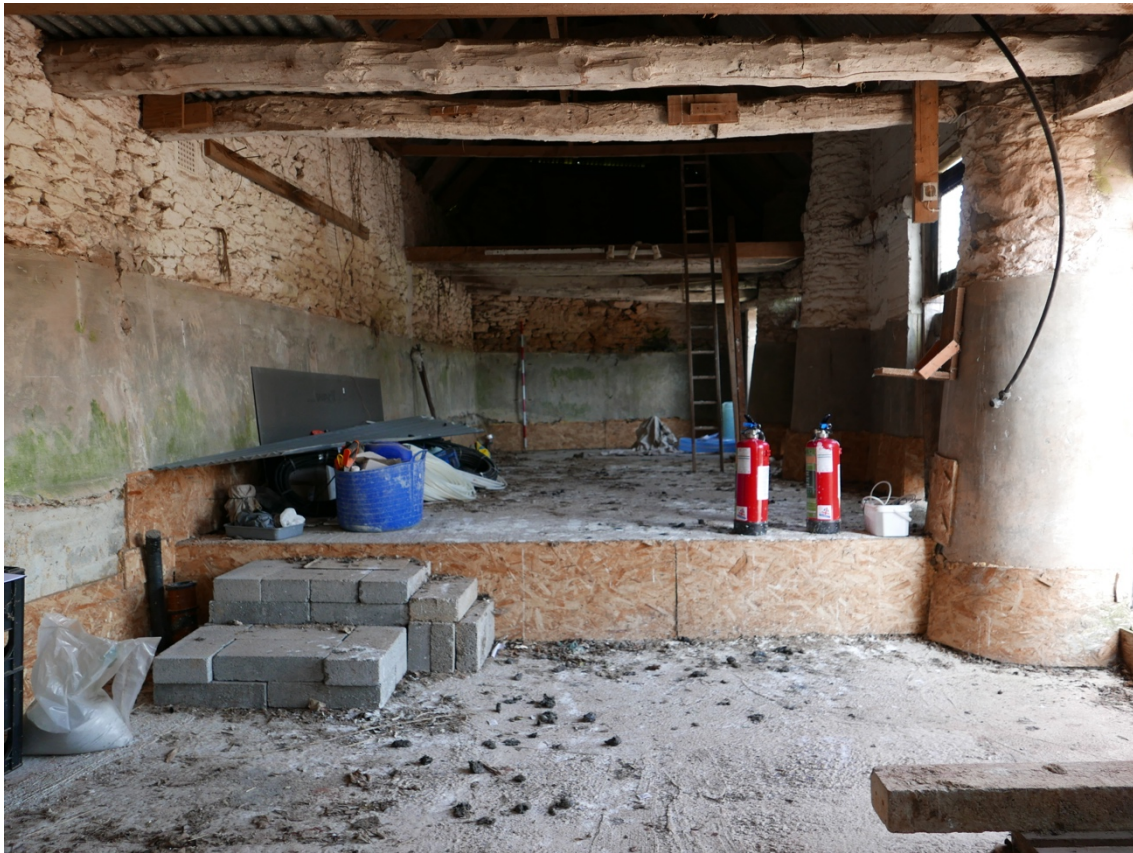
Plate 28. Interior. North end looking north.
