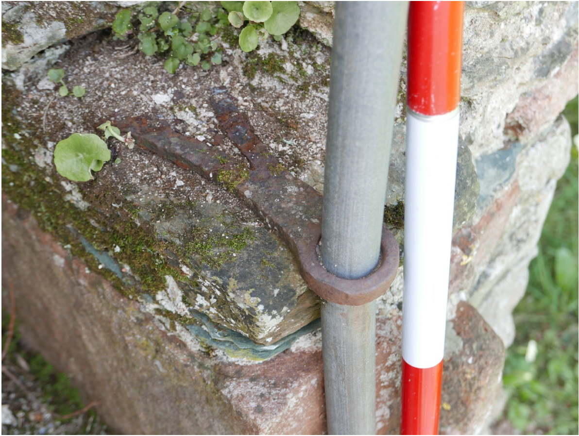
Plate 4. Iron stay for handrail.
