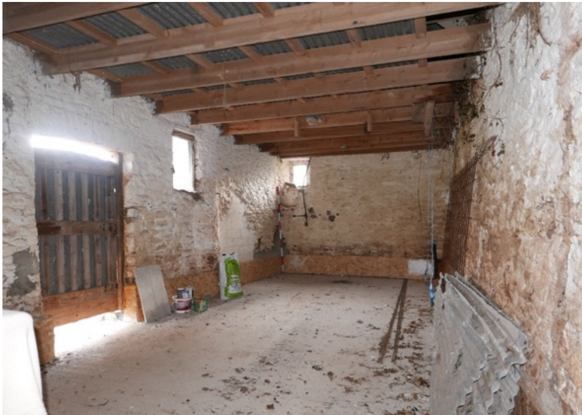
Plate 25. Interior. South end looking towards SE.
