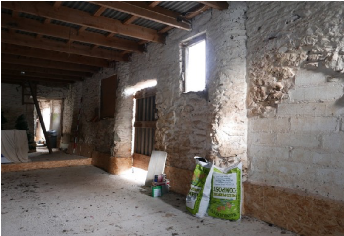
Plate 27. Interior. South end looking towards NE.
