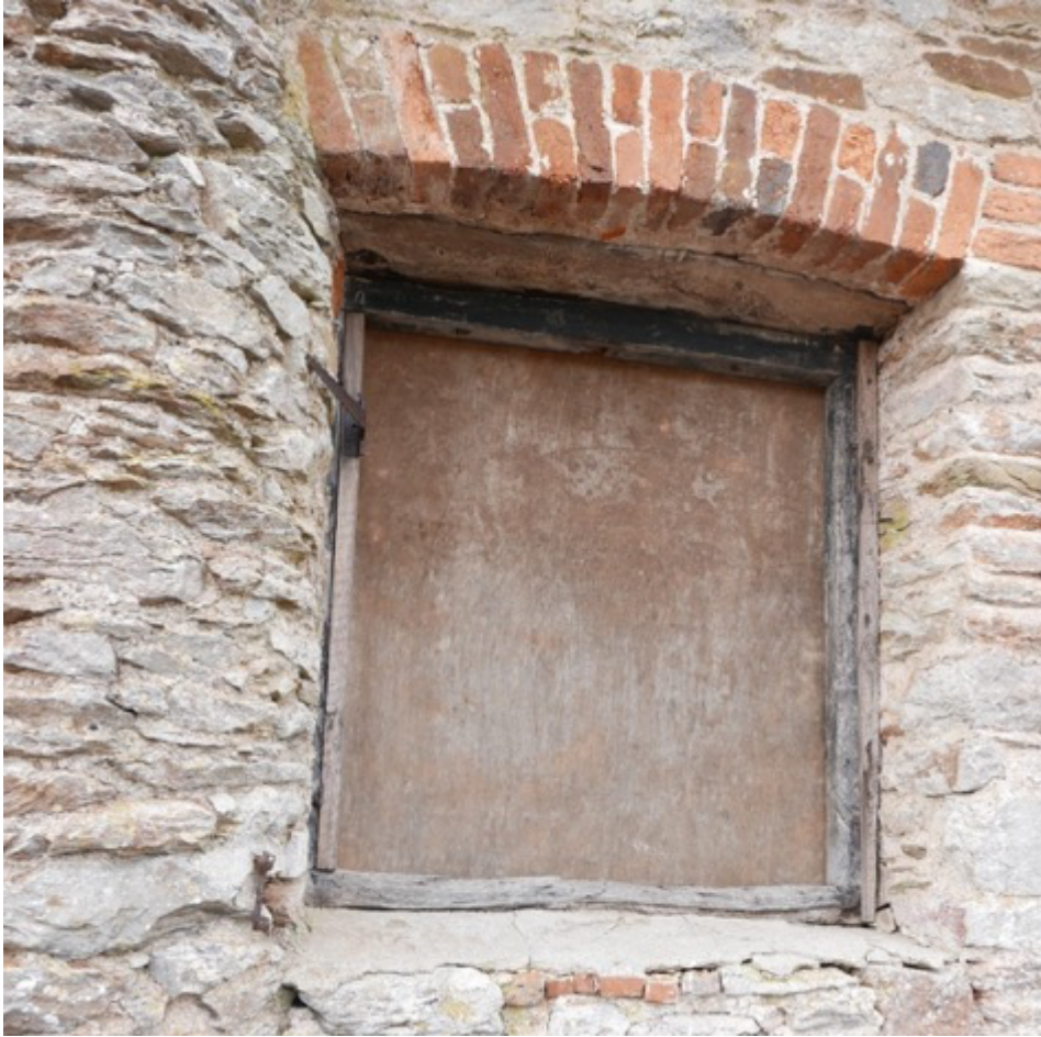
Plate 11. Bay 3 window, east elevation.
