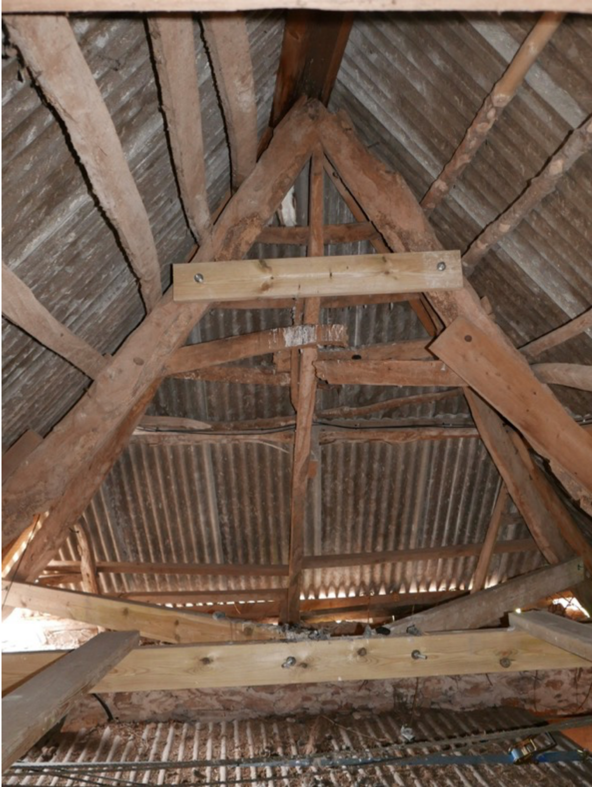
Plate 44. Interior. Roof - South end hipped roof structure (spot the barn owls).
