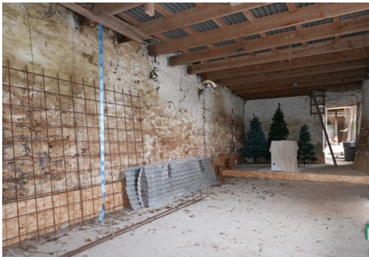
Plate 26. Interior. South end looking towards NW.
