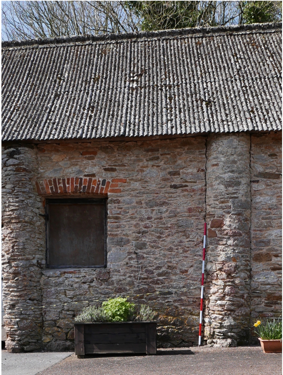
Plate 10. East elevation, Bay 3.
