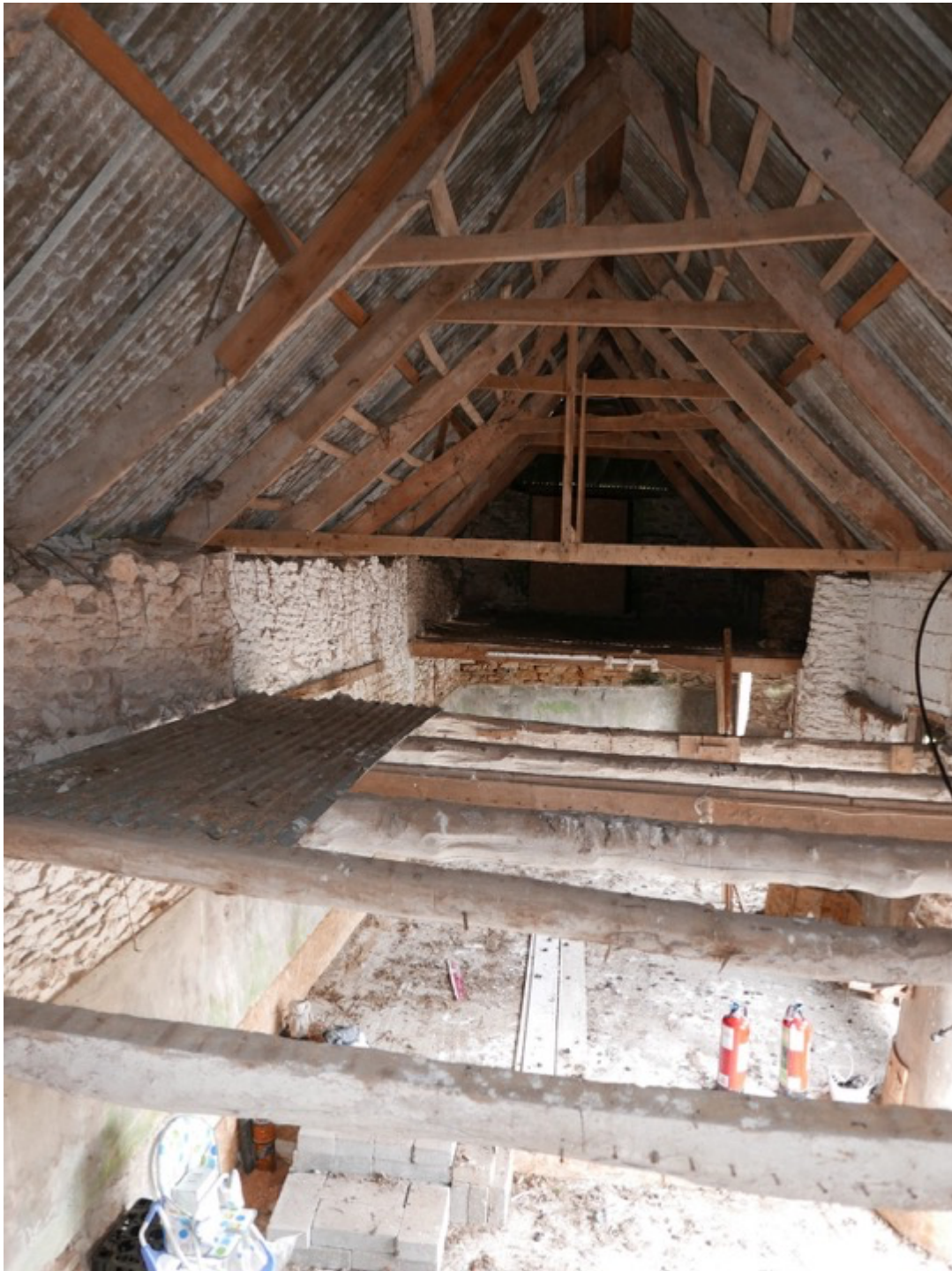
Plate 36. Interior. Upper floor north end looking north.
