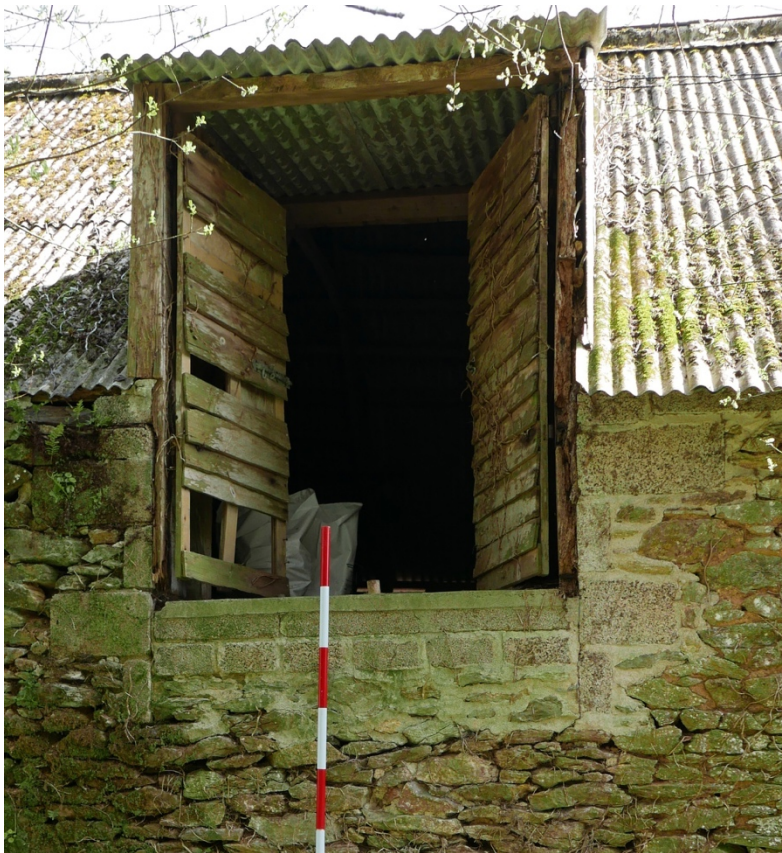
Plate 23. Pitching door, west elevation.
