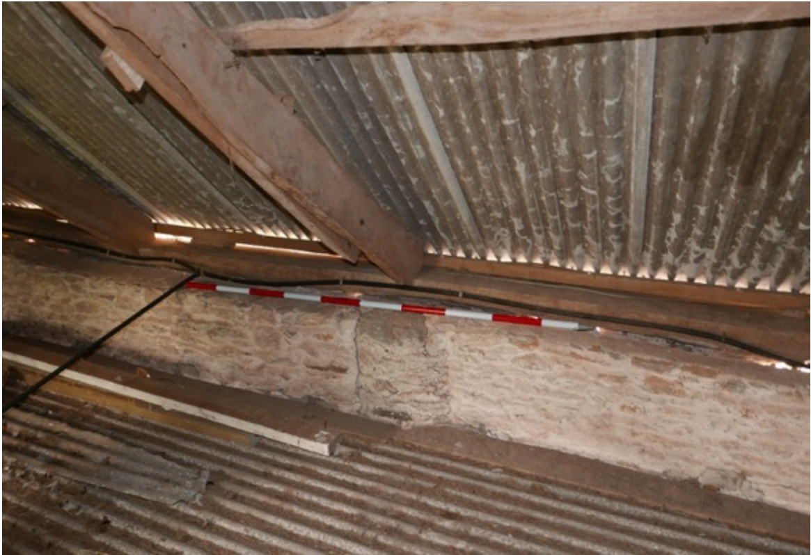
Plate 41. Interior. Roof south end pier and wall plate detail.
