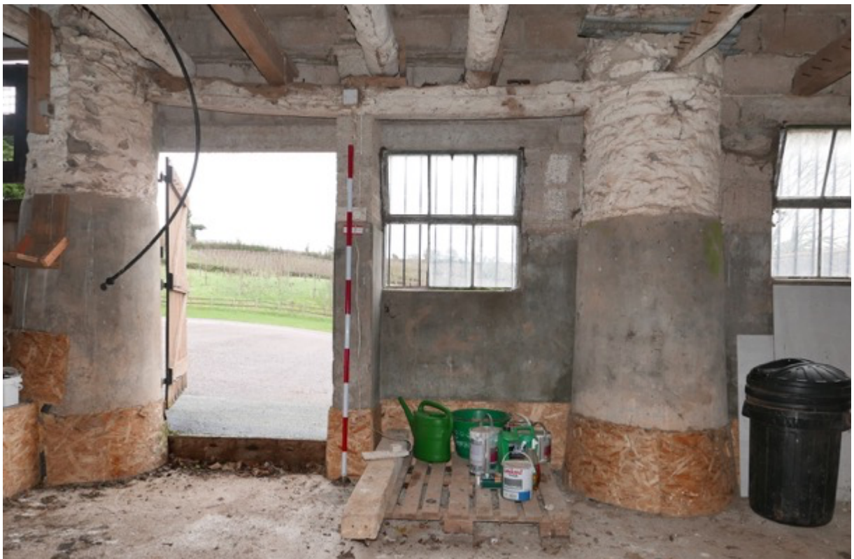
Plate 32. Interior. North end Bay 5.
