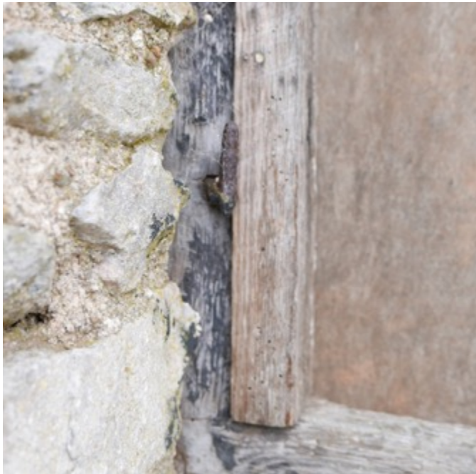
Plate 12. Pintle on Bay 3 window, east elevation.
