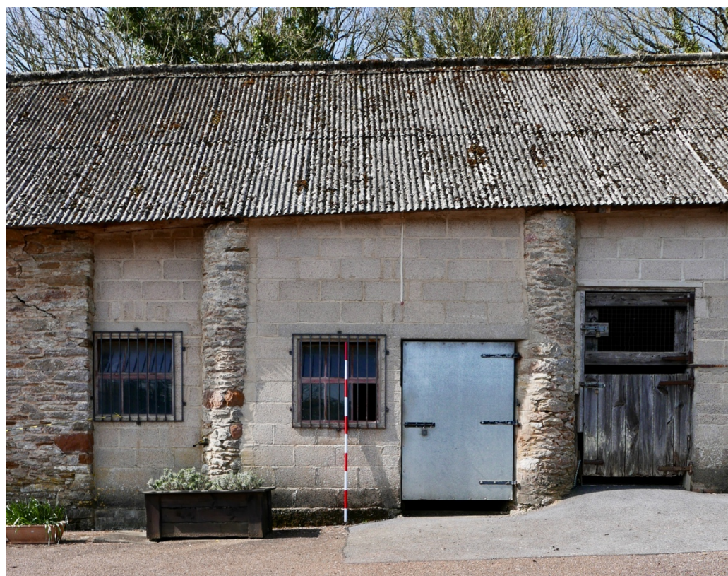
Plate 14. East elevation, Bay 5.
