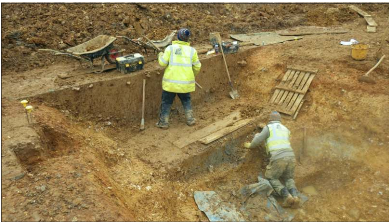
Plate 6: Excavation area, working in progress, excavating southern section of cross ridge dyke ditch F1012, looking southwest
