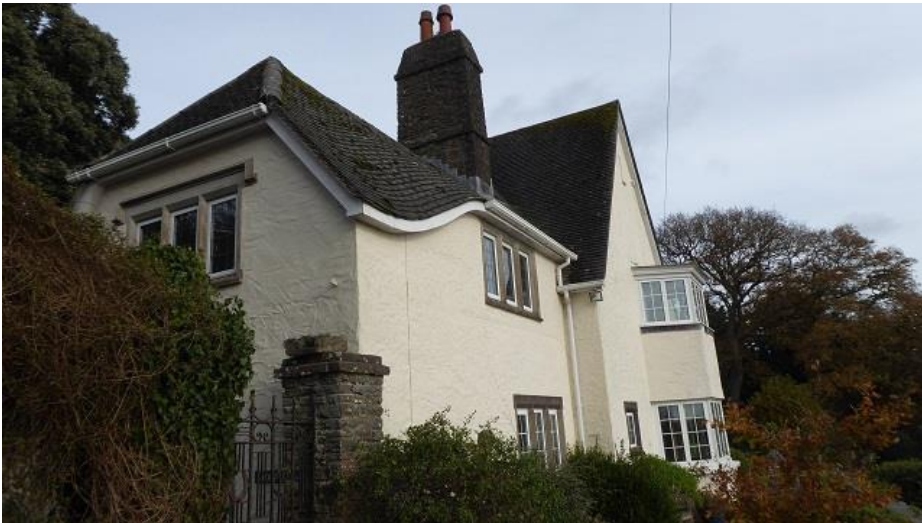
South-west corner shows that the hipped gable (shown above) has a swept eaves to the right-hand side.
