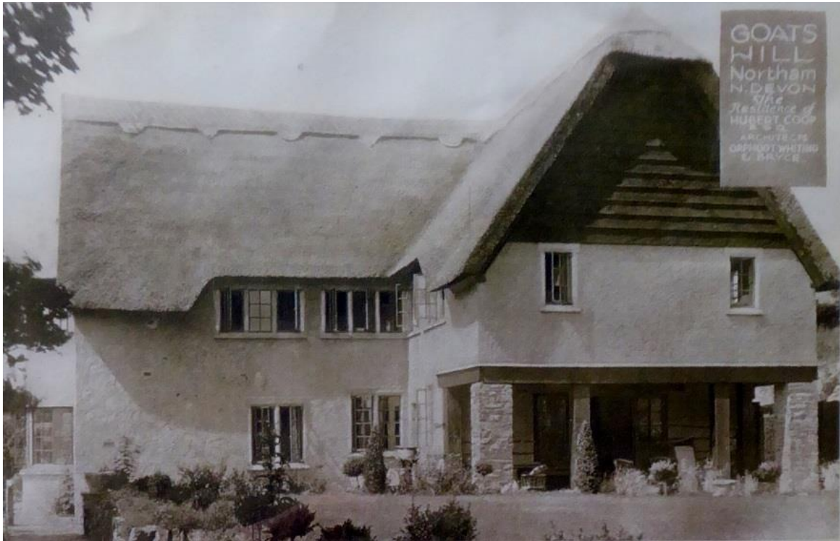
“Goats Hill, Northam, Devon, is an example of the small and essentially modern house which has happily recaptured local characteristics and the charm of older buildings - rough plastered cob walls, plinths of tar, thatch, and buttressed chimney stacks.” (Ideal Home Magazine, April 1925)
