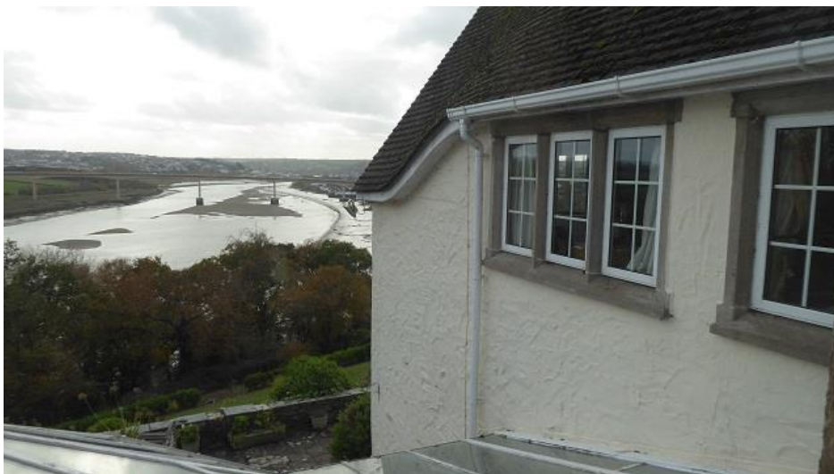
General views of First Floor rooms. No discernable antique or architectural features evident on this floor.
