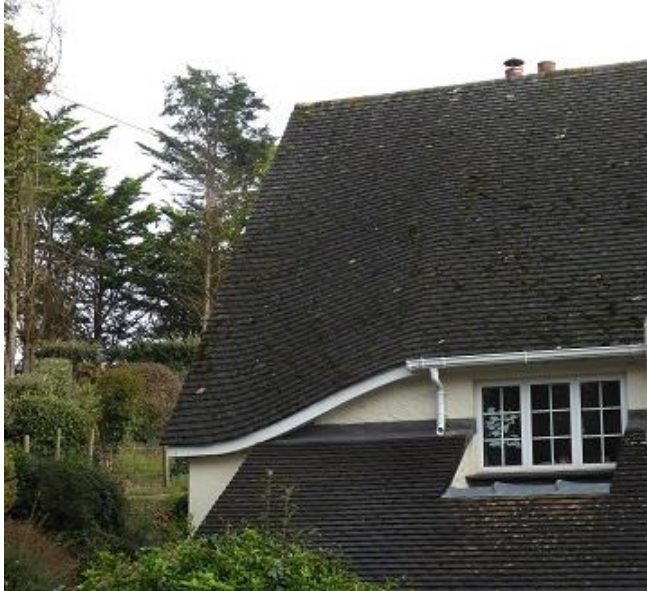
North-facing gable end showing swept eaves. The roof was originally thatched, but when re-tiled in the 1950s, the same detail was retained.
