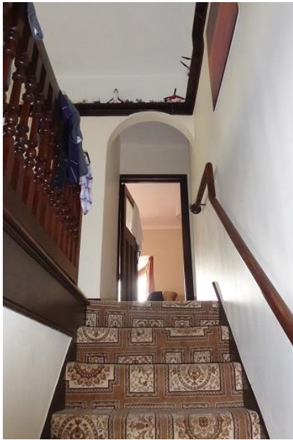
Above: Stairs to First Floor
