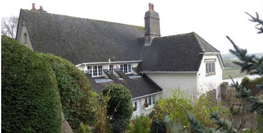
View from the rear – the north-west corner.
