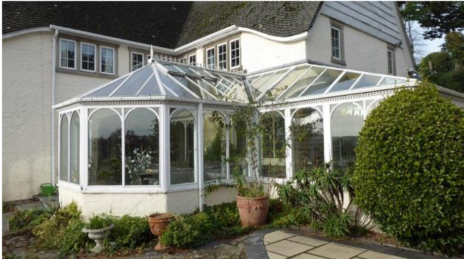
South-east corner showing conservatory.
