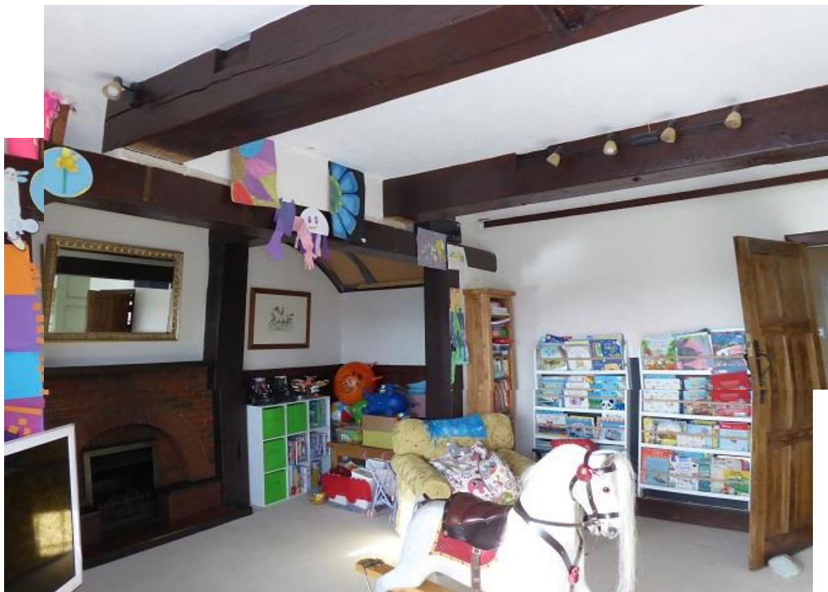
View looking towards the fireplace recess, which is partly screened on each side with small wings formed from stained timber uprights similar to those used each side of the fireplace itself. The Living Room is dominated by two large-sectioned stained softwood beams, each 11-inches square. These run in towards the fireplace area and align with the uprights each side of the fireplace. These beams bear many marks of having been used in a previous structure – this will be detailed further in the section of this report called ‘Beam Markings.
