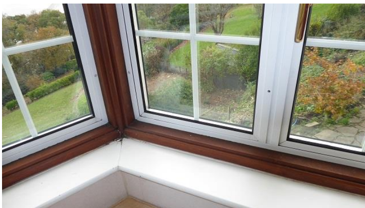
Above: Double-glazed uPVC windows throughout upper floor level.
