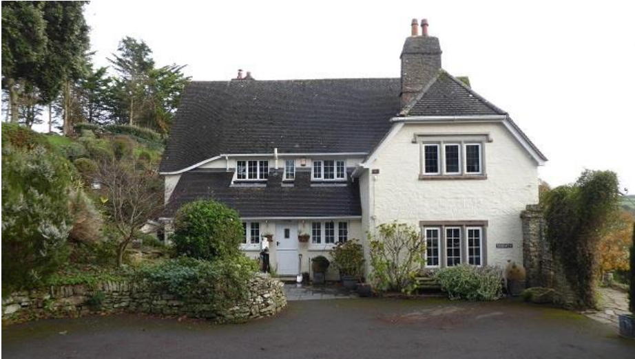
West-facing façade from the driveway. Note the hipped gable end to the western wing.
