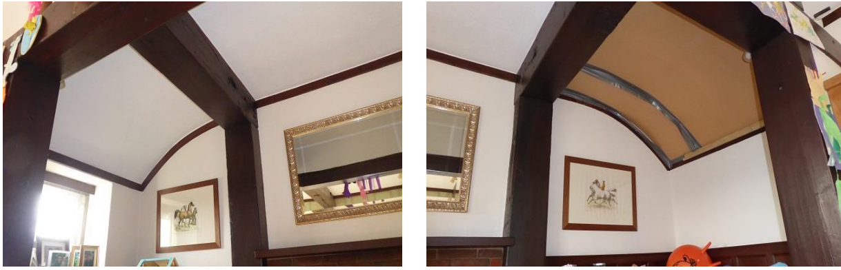
Above: Images showing the two inglenook wings each side of the fireplace, which are topped with curved plastered ceilings with dark-stained timber trims.
