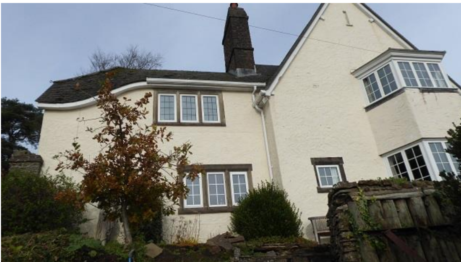
South-facing façade. The double-height bay window was not shown on the original plans, so was presumably a later addition. All windows are upvc replacements in original stone frames.
