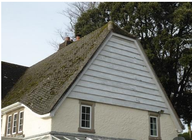
East-facing gable showing small hipped end and straight-edge overlapping timber cladding. Note the swept eaves to this elevation.
