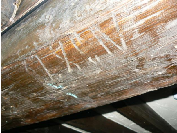
Left: Cargo marks on beams at 3 Bridge Street, Bideford.
