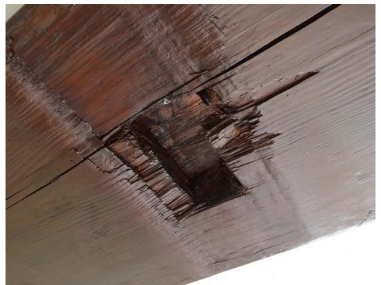
Above: beam and post sockets in the imported softwood beams, showing further evidence of their former use.
