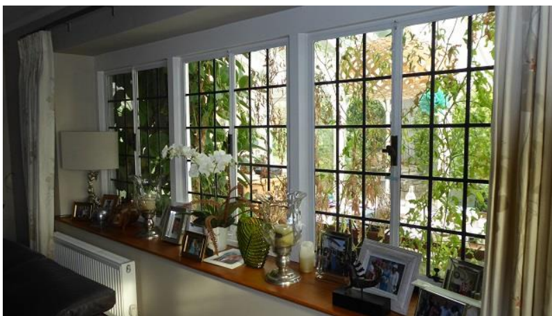
South facing window.
