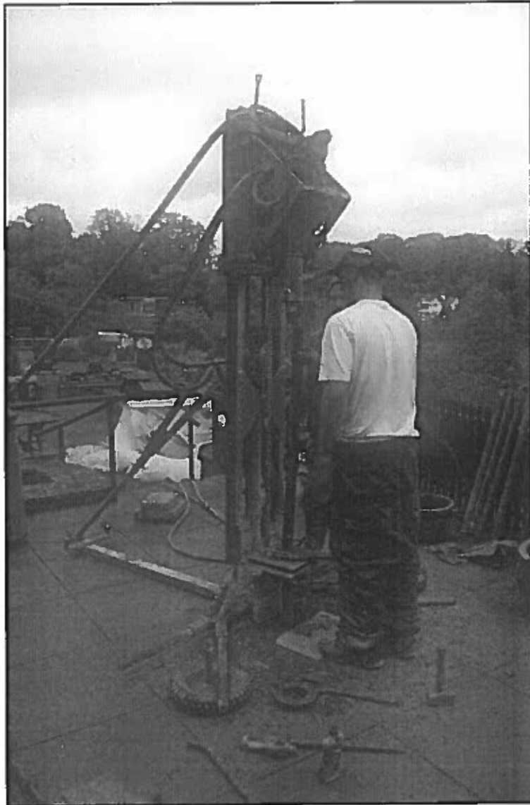
Pl. 3 Drilling rig set up over borehole 3. Looking north.
