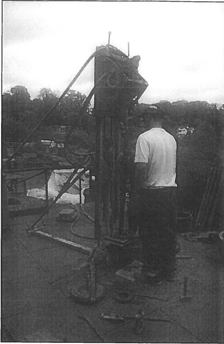
Pl. 3 Drilling rig set up over borehole 3. Looking north.
