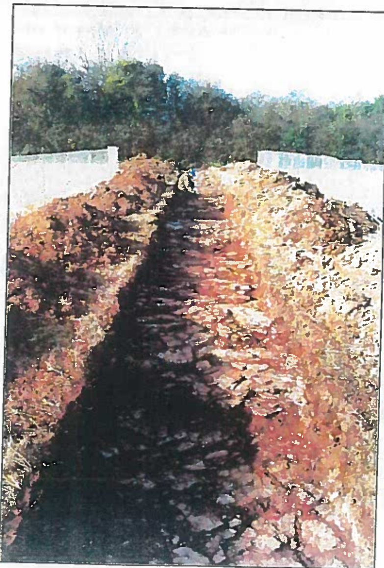
Pl. 2 Trench 1 (looking north-west).
