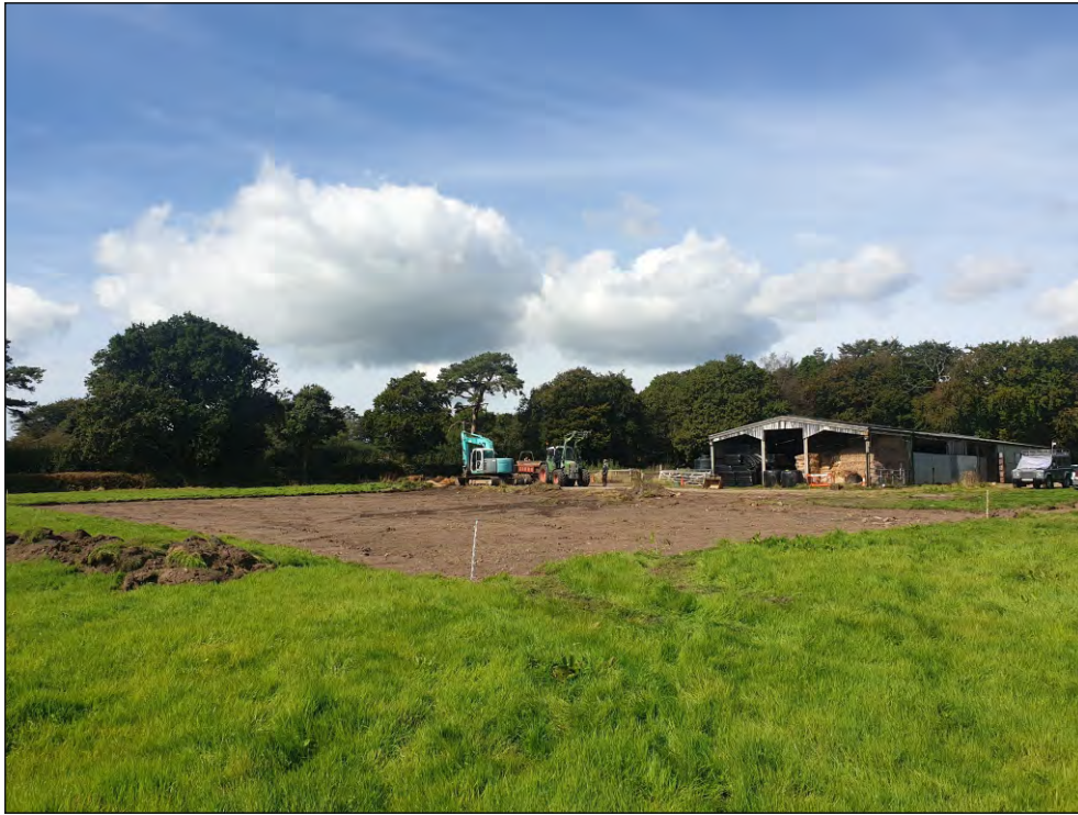
Pl. 1 General view of the manege. Looking northwest.
