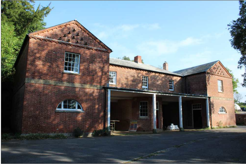
Plate 1: Southeast elevation, looking north (1m scale)
