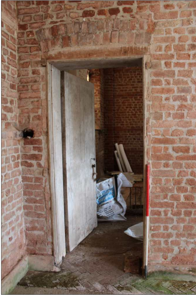
Plate 5: Original four-panel door in the east garage, looking north (1m scale)
