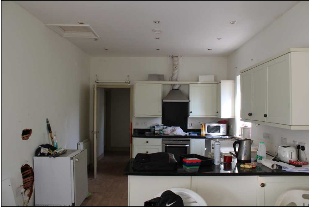
Plate 13: Kitchen on first floor, showing modern finishes and fittings, looking northwest (1m scale)
