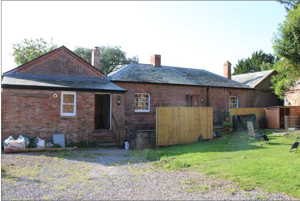
Plate 7: Northwest elevation, looking southeast (1m scale)
