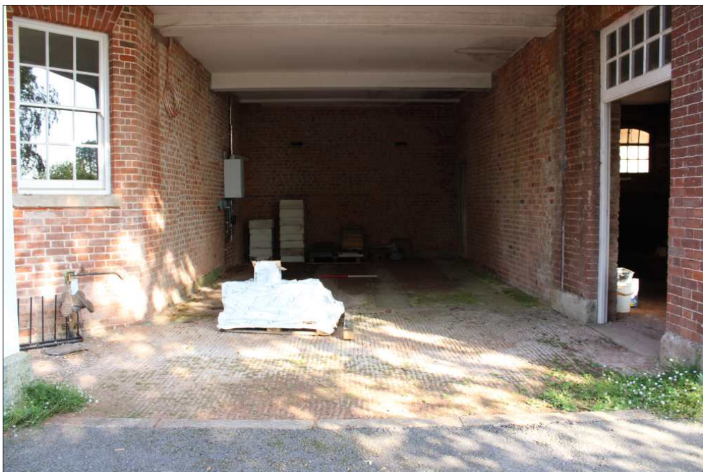
Plate 2: East garage, looking northwest (1m scale)
