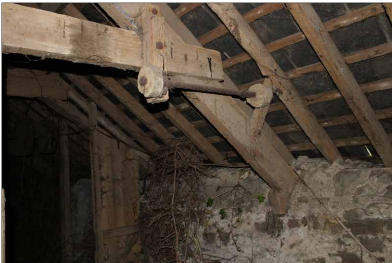
Plate 17: First-floor granary, detail of driving spindle, view from below, looking northeast
