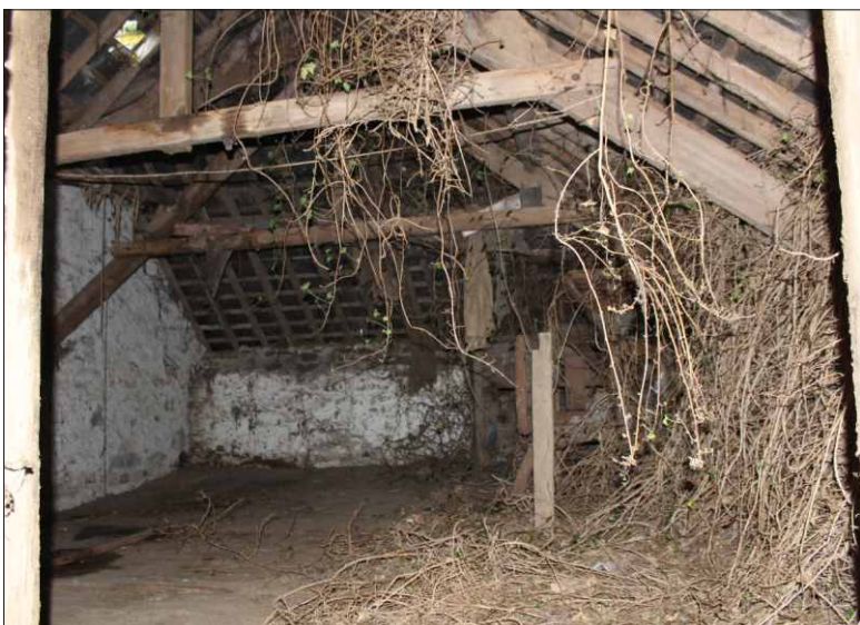
Plate 18: First-floor hayloft/engine house in the south range, looking north
