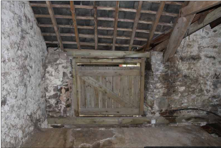
Plate 19: First-floor hayloft/engine house, detail of hayloft door, looking west
