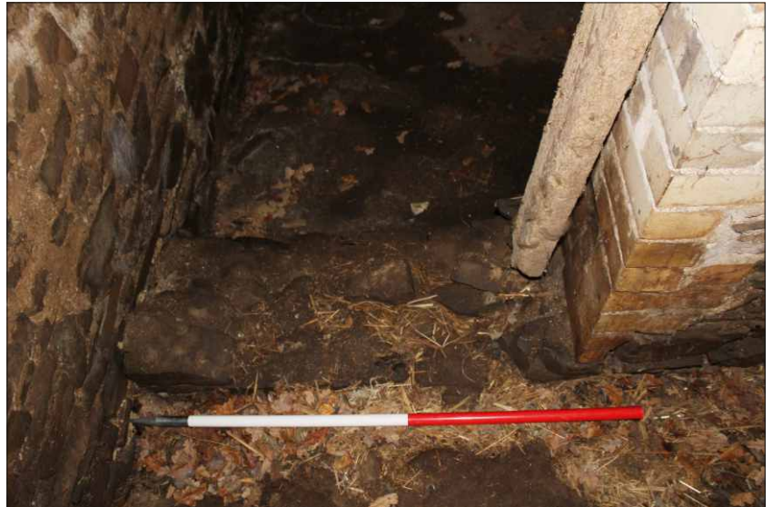
Plate 8: Detail of inserted opening at north end of threshing barn into granary, view from above, looking south (1m scale)
