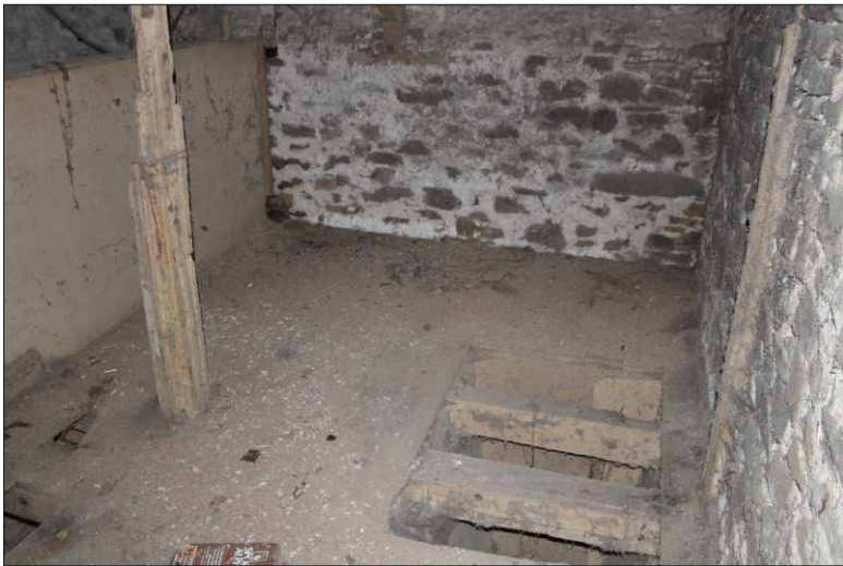
Plate 16: First-floor granary within partitioned corner, showing shaft to grain chute below, looking east
