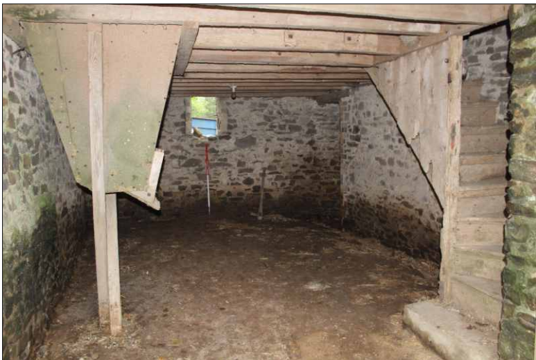
Plate 11: Ground-floor granary in the south range, looking east (1m scale)
