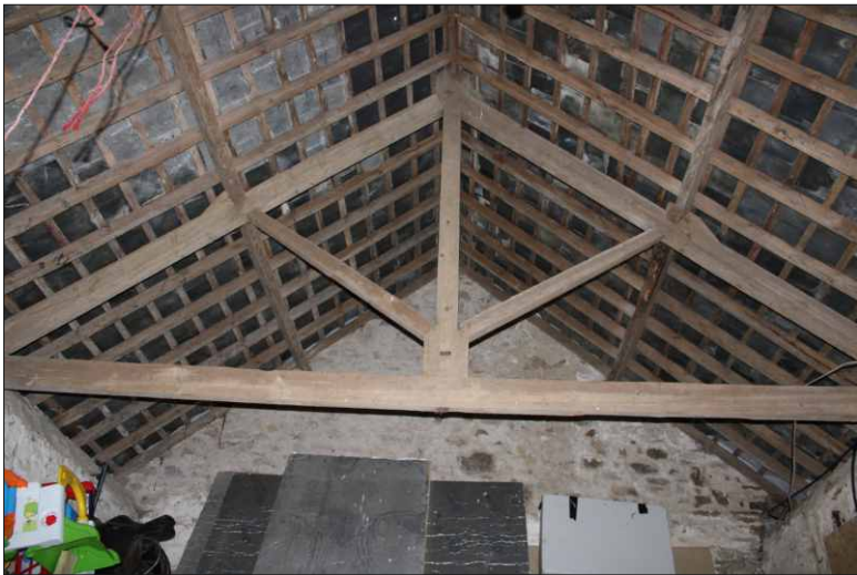
Plate 28: Roof structure in east room of north range, looking east
