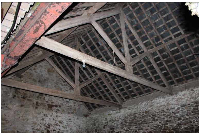
Plate 30: Roof structure in west room of north range, looking northwest
