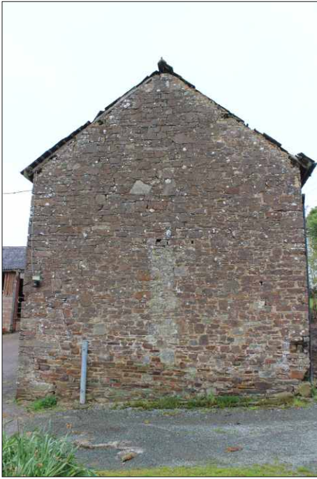
Plate 4: South elevation of south range, looking north
