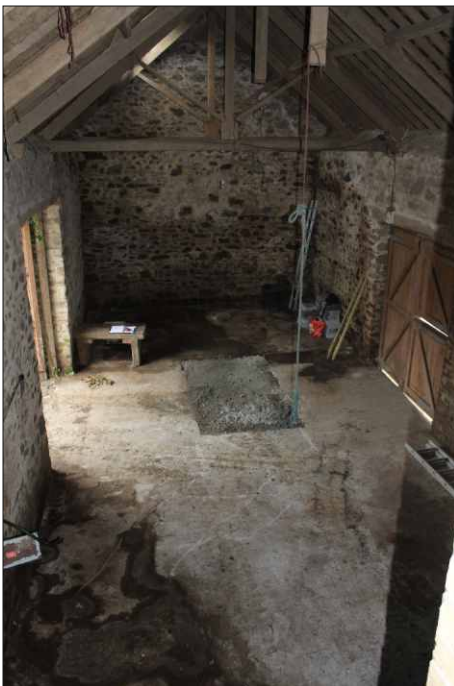
Plate 6: Internal view of threshing barn in the south range, looking south
