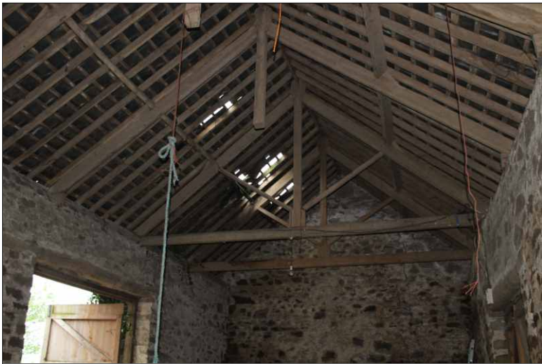
Plate 10: Roof trusses within the threshing barn, view from below, looking southeast
