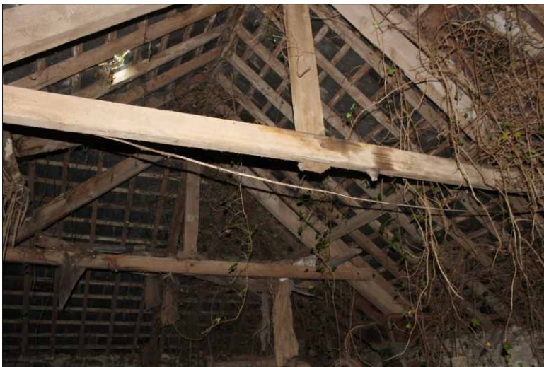
Plate 20: First-floor hayloft/engine house, detail of trusses, view from below, looking northeast
