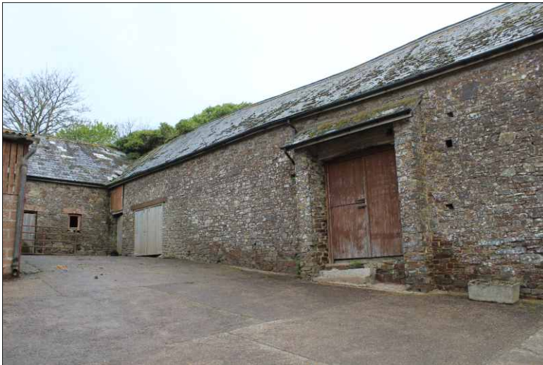
Plate 2: West elevation of south range, looking northeast
