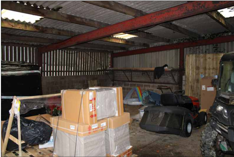
Plate 25: Internal view of the late 20th century lean-to, looking southwest
