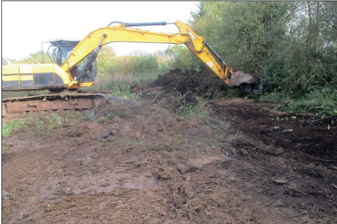
Site clearance and demolition of earthwork bank in Area 1, looking north-west
