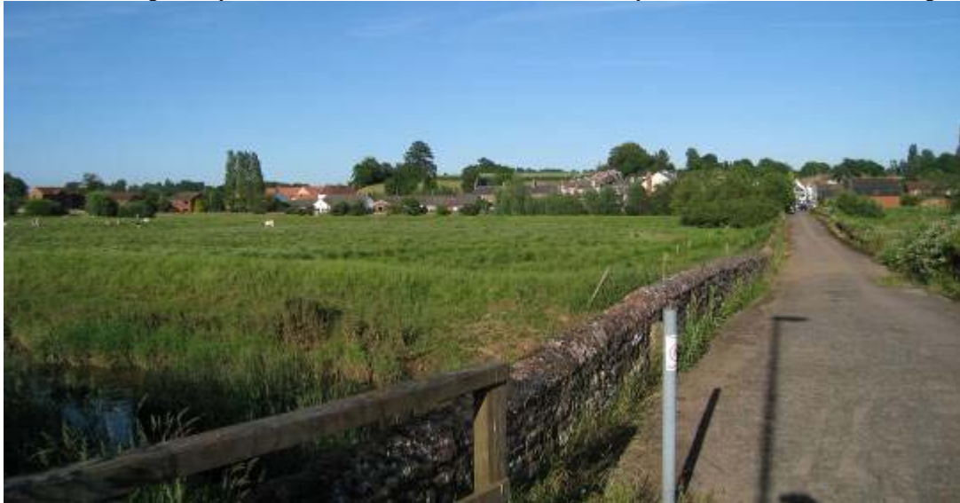
Figure 14: View from Clyst Bridge looking back towards Bishop's Clyst. The length and narrow width of the causeway made possible the defence of the bridge by a single artillery piece.
